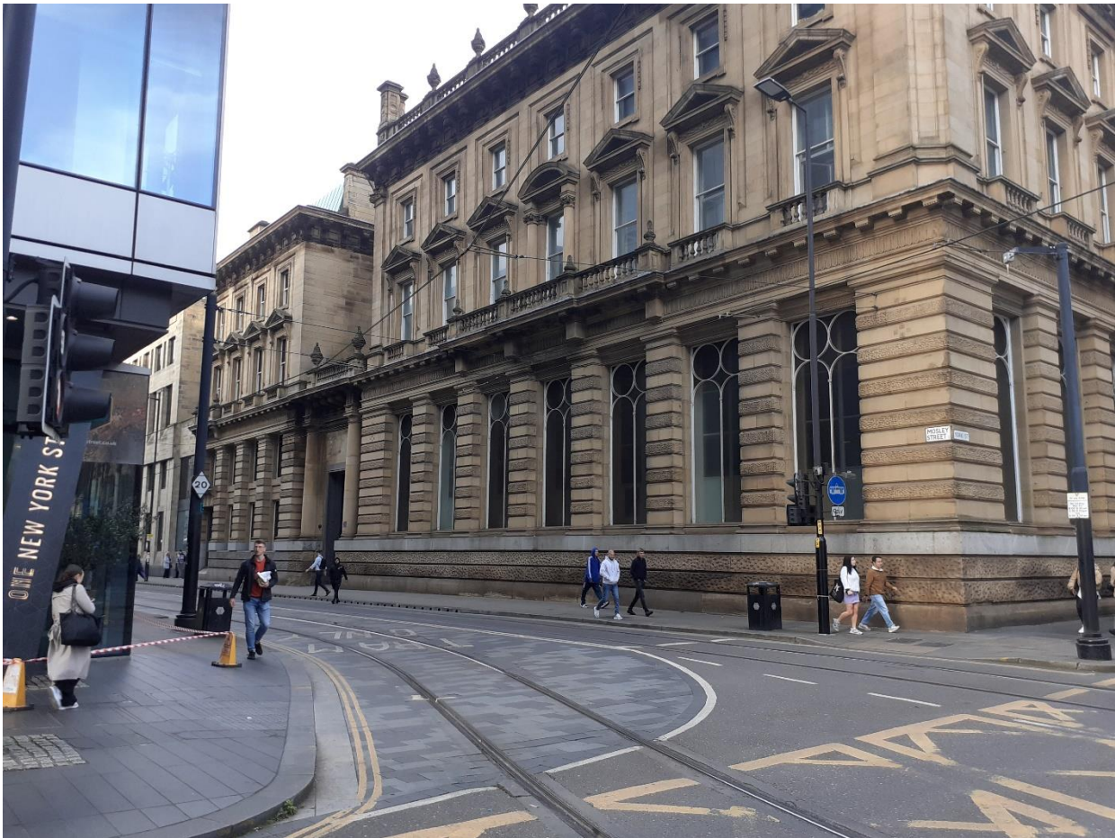
Figure 2: View along the Mosley Street elevation of the building.
