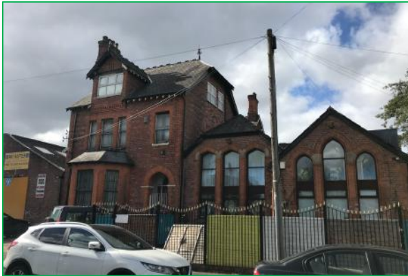
The northeast elevation (front) of the Nursery (2022)
