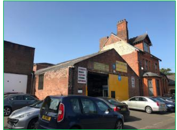
The northeast and southeast elevation of Structure A of the MOT Centre (2022)
