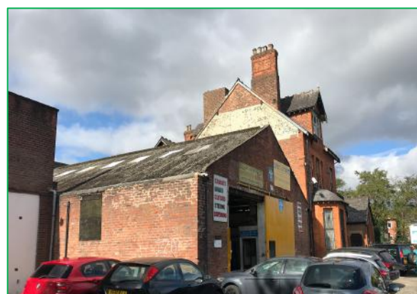
The northeast and southeast elevation of Structure A of the MOT Centre (2020)
