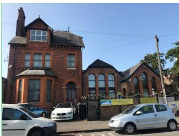
The northeast elevation (front) of the Nursery (2020)
