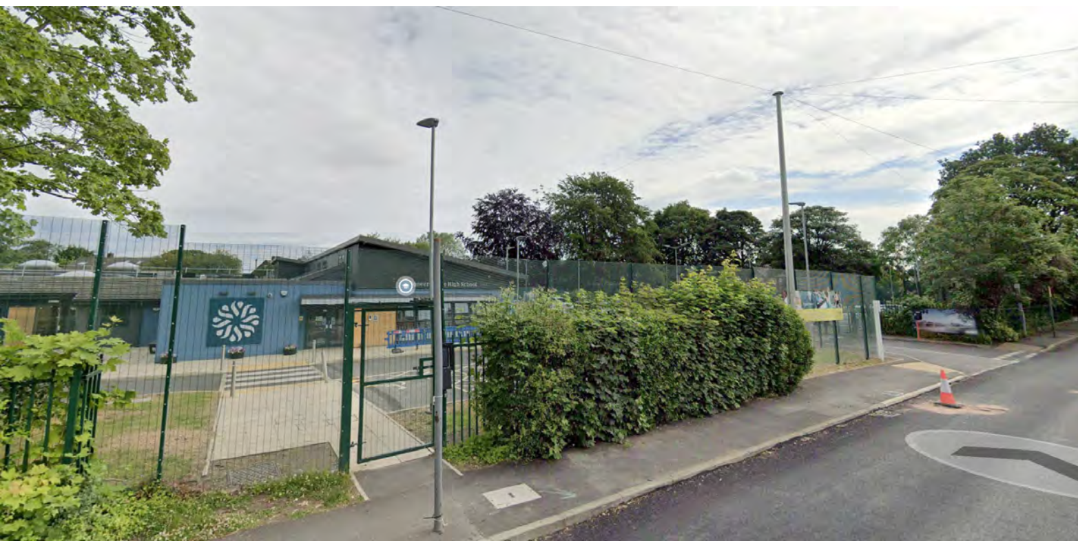
Existing 3m high security fence
