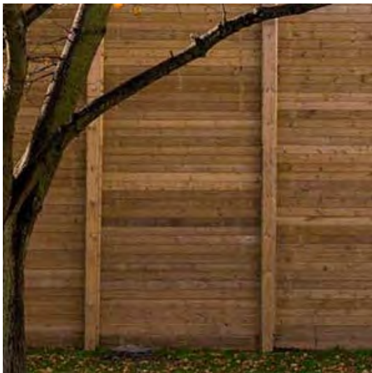
6. Timber fence to outdoor classroom
