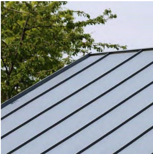
2. Standing seam metal roof. Mid-grey
