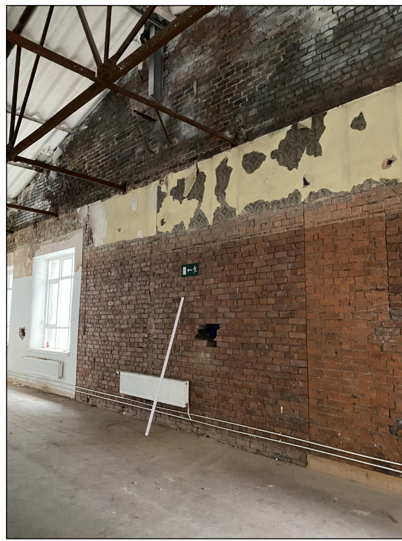
IMAGE 3 Existing semi-exposed brick to be fully exposed up to new suspended ceiling level. Brickwork to be re-pointed. It is believed that any historic wall coverings are not salvageable and beyond repair
