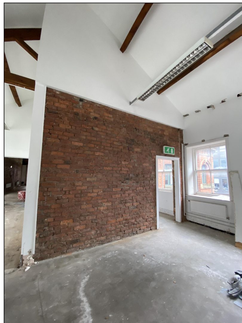
IMAGE 1 Existing exposed wall finish to remain exposed and re-pointed where required
