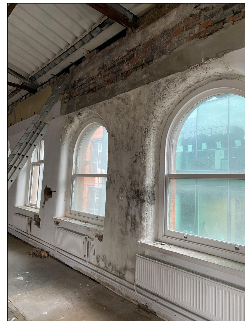
IMAGE 4 Existing wall finish to be replastered up to new suspended ceiling level which is approximately 3500mm. Any perforations through walls to be made good
