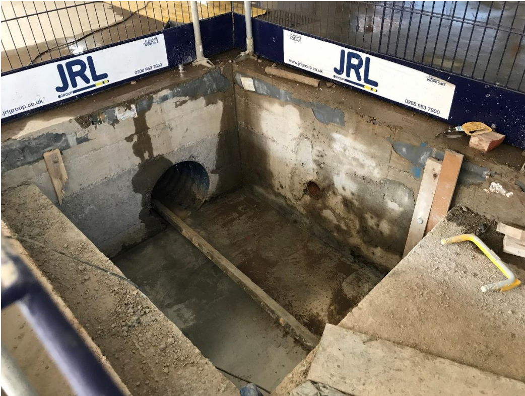
Photo 3 – Flow Control Chamber Construction – Incoming 600mm diameter storage pipe
