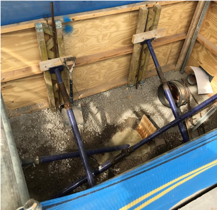
Photo 2 – Installation of Winsor Interceptor on outfall of flow control chamber
