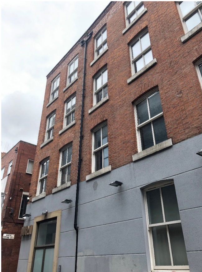
Figure 2.13: Principal elevation of the Spear Street Warehouse, facing Spear Street
