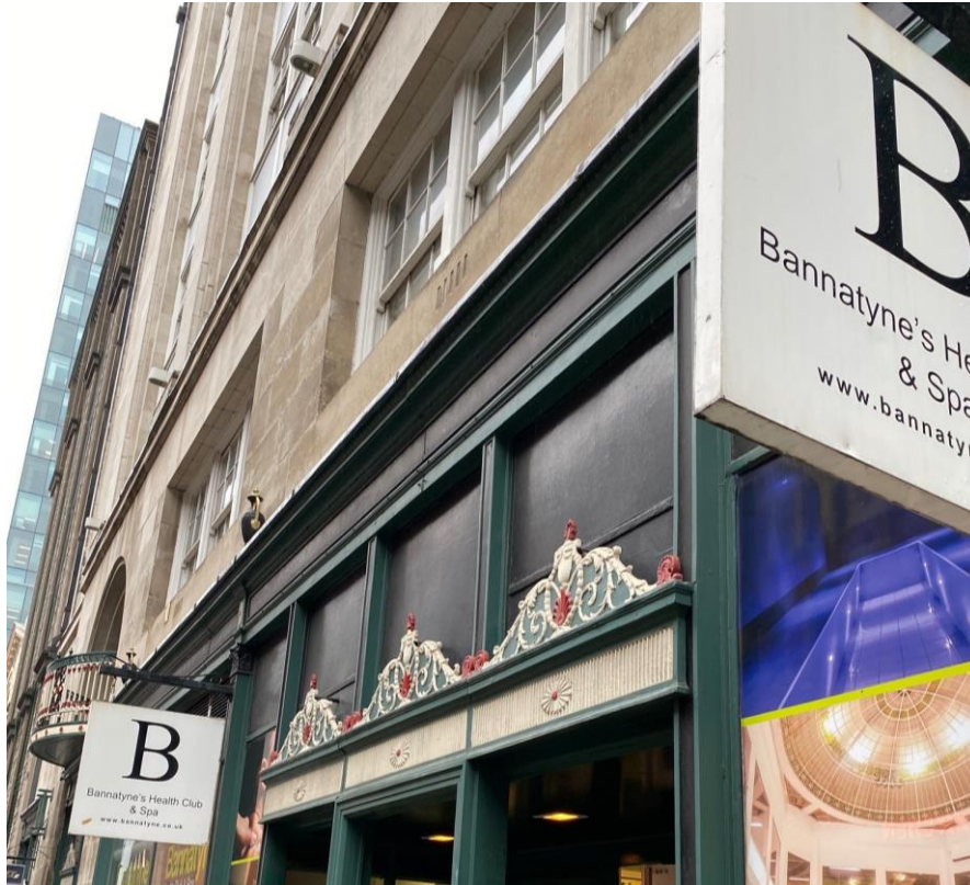
Photographs from Site Visit – 16 th November 2022
