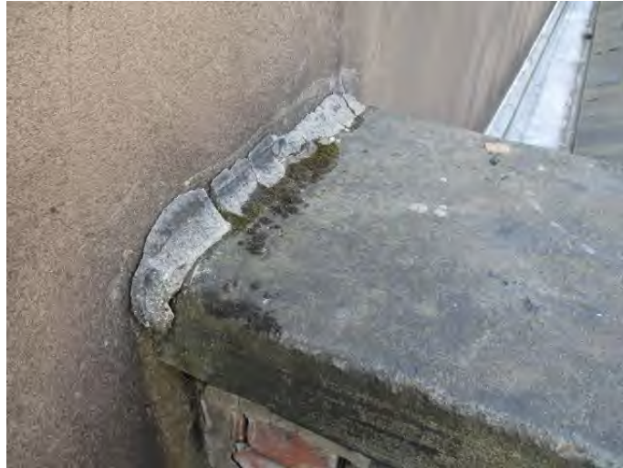
7. The render to the central parapet had cracked.
