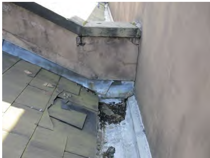
7. The render to the central parapet had cracked.
