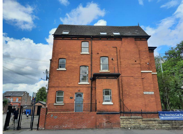
Plate 2: Eastern Elevation of B1.
