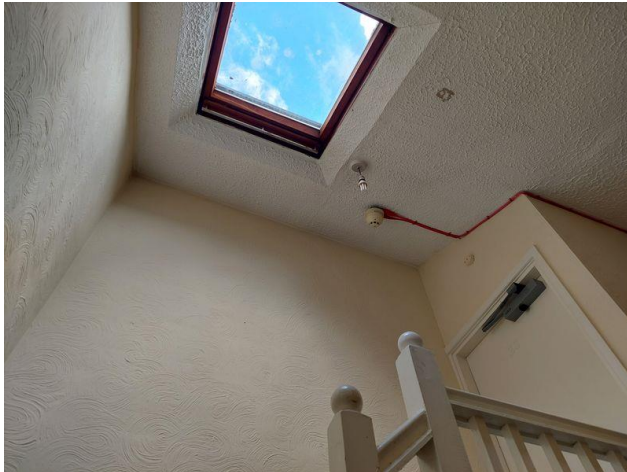
Plate 15: Inside of Building Redeveloped Into Flats with Narrow Corridors and Stairwells
