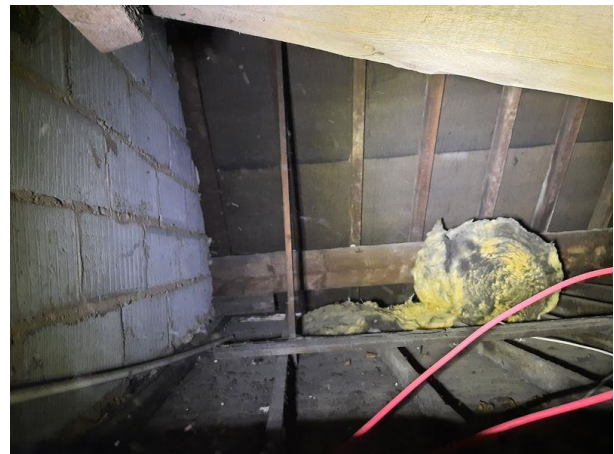
Plate 8: Some Areas of Insulation within the Roof Space
