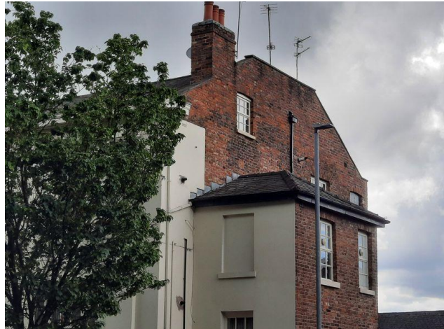
Plate 11: Mansard Style Roof, Wooden Fascia Boards, and Wooden Framed Windows Consistent Throughout The Building
