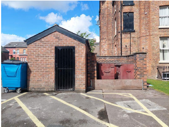
Plate 18: Small Bike Shed Structure to The South of The Main Buildings
