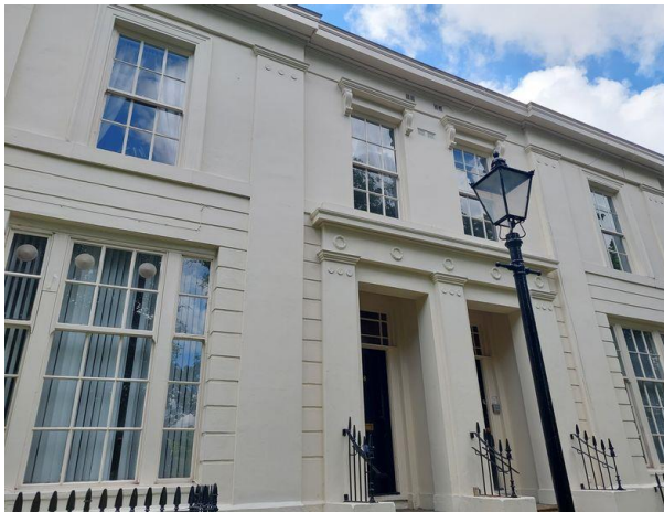
Plate 12: North Of The Building Entirely Painted up To Roof and in Good Condition
