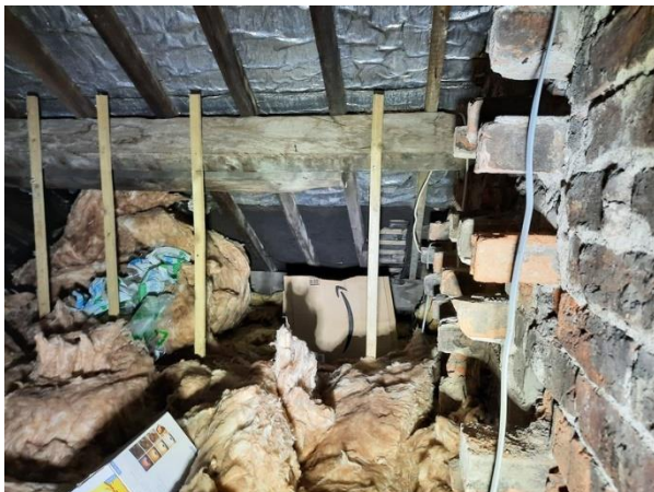
Plate 17: Foil Lined Roof Felting Visible to the West
