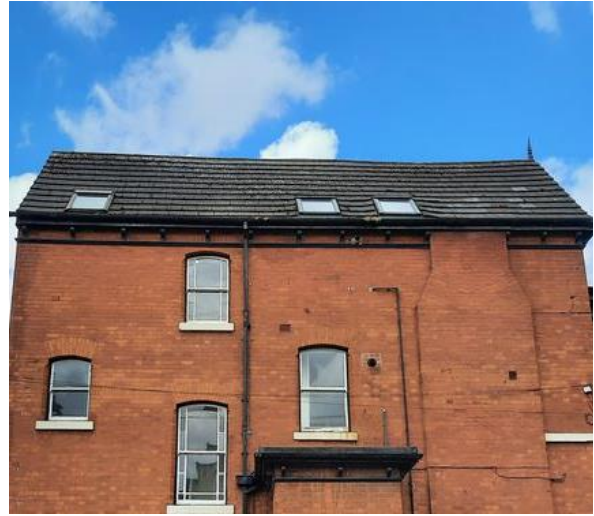
Plate 6: Skylights Visible From The Outside Of The Building Associated With the Attic Flats
