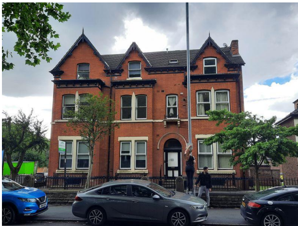
Plate 3: Ornate Fascia Boards on Southern Elevation
