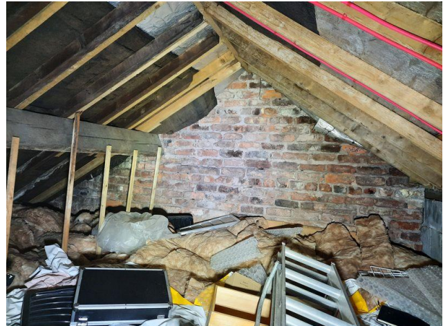
Plate 16: Inside of the Attic Space with Insulation and Aerial Cables Visible
