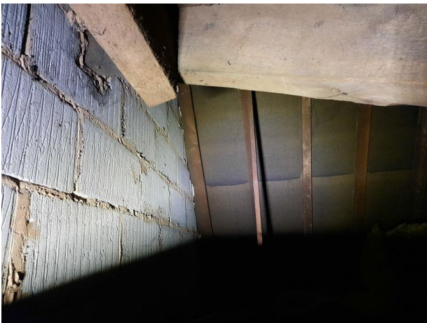
Plate 7: Area within The Attic Space, Separated By Breezeblocks
