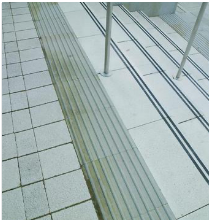
4- Scoutmoor corduroy tactile paving
