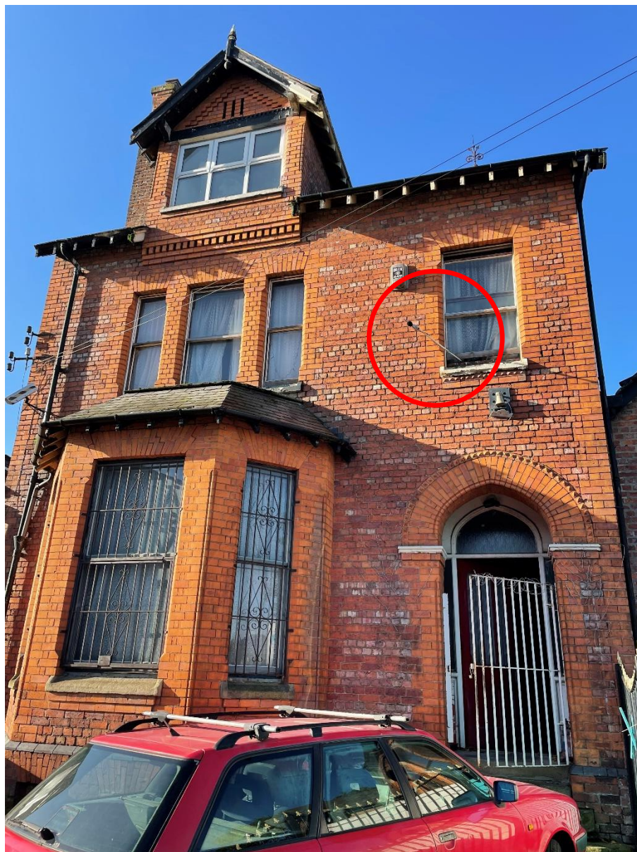
Noise monitoring location at first floor of existing dwelling, overlooking Carmoor Road.
