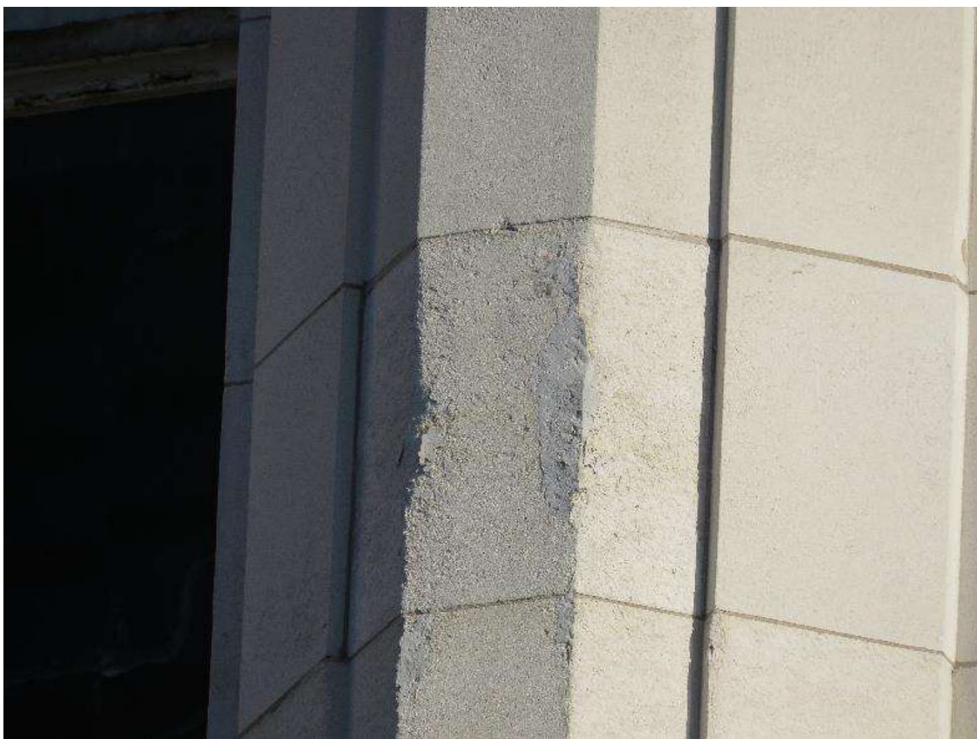
Fig. 5: The fine joints of the Portland stone cladding has a cream coloured mortar with very little aggregate, most likely a lime putty mortar with a fine aggregate.
