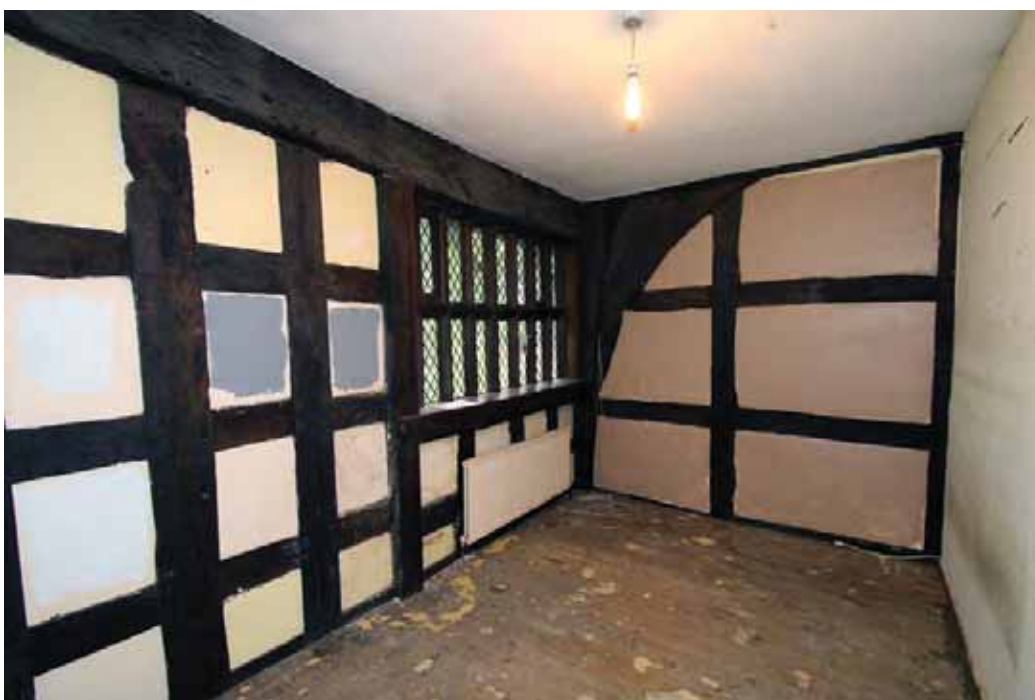
Plate 32. Bay 2, first floor, bedroom 2, viewed from north.
