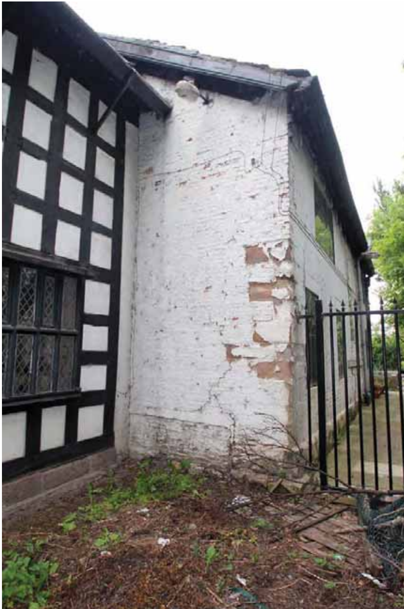
Plate 8. East elevation, junction between bays 2 and 3, viewed from south-east.
