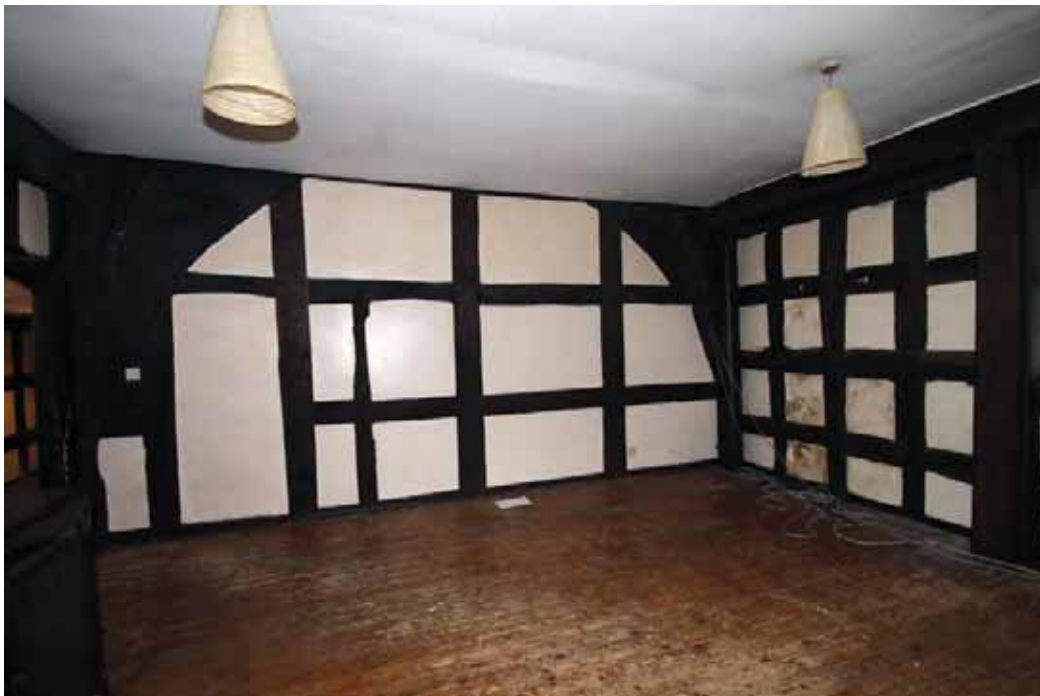
Plate 28. Bay 1, first floor, south bedroom, viewed from south.
