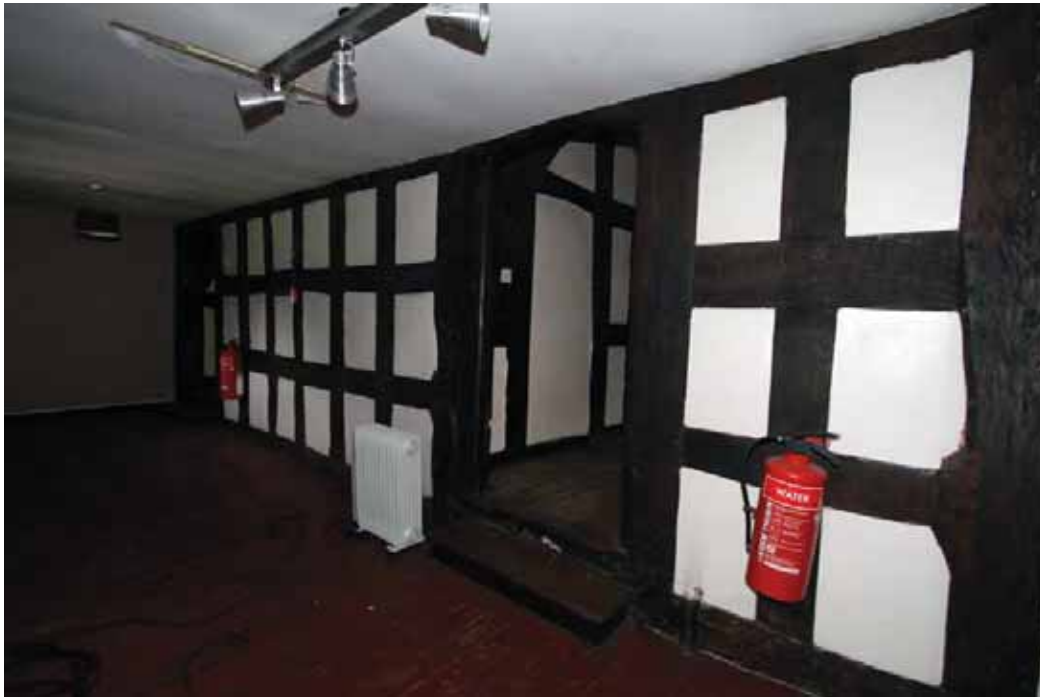
Plate 23. Bays 1 & 2, first floor corridor, viewed from south-west.
