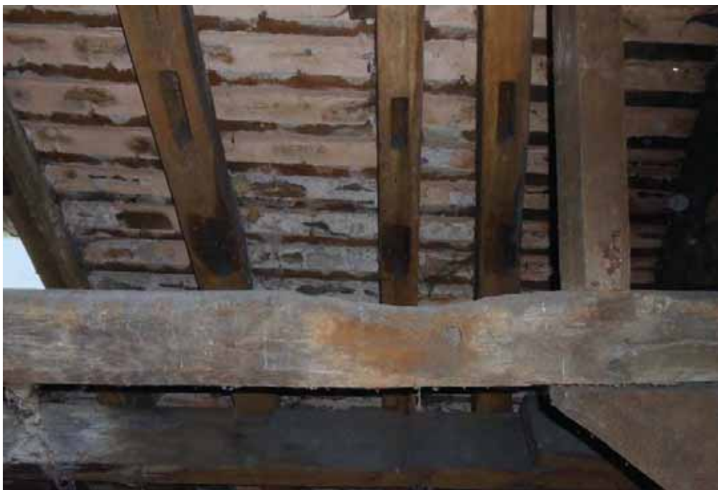
Plate 37. Bay 2, roof space, crown plate and double mortices to rafters, viewed from west.
