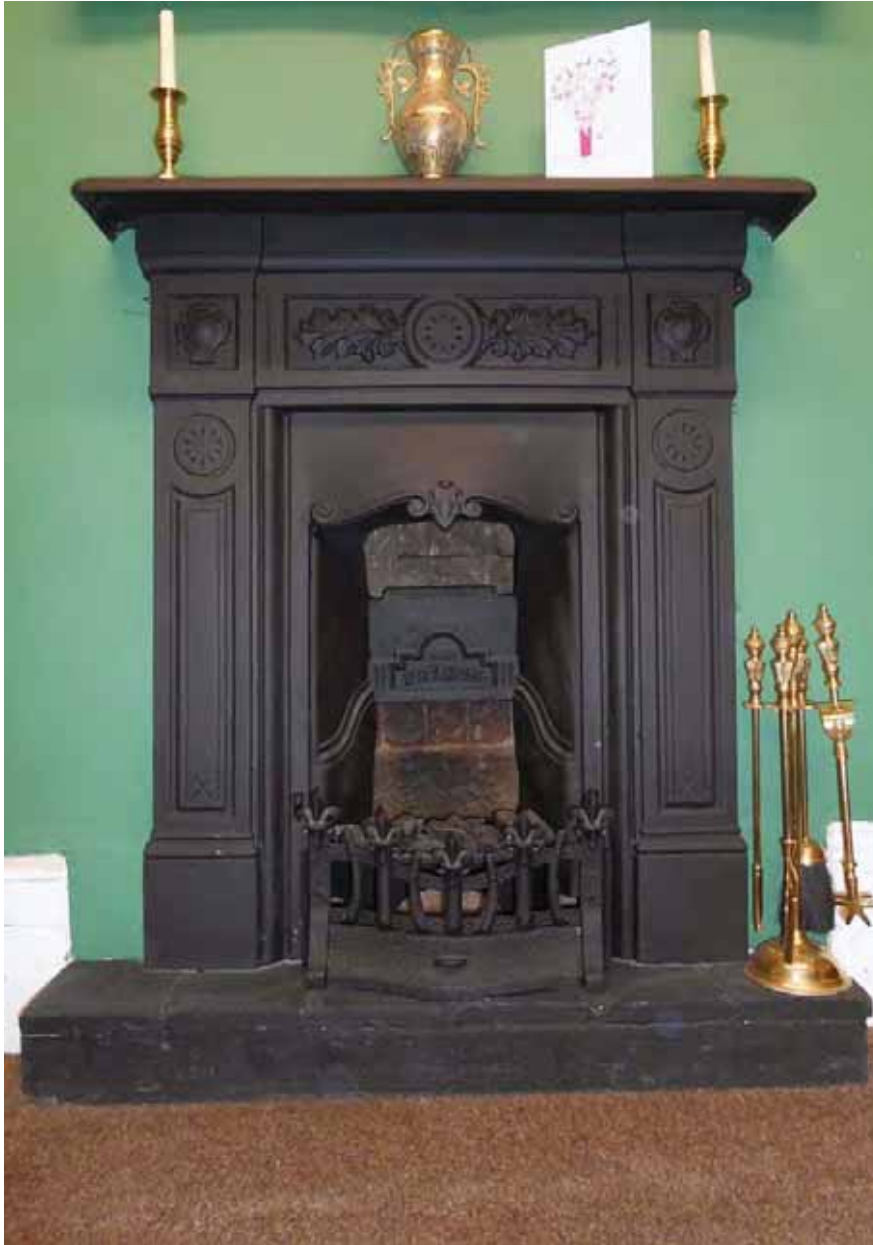
Plate 66. Brick house, first floor, bedroom over dining room, inserted fire-surround, viewed from west.
