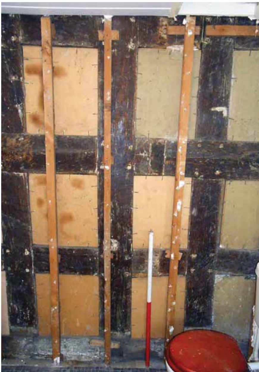
Plate 69. Watching brief – exposed east wall of first floor bathroom.
