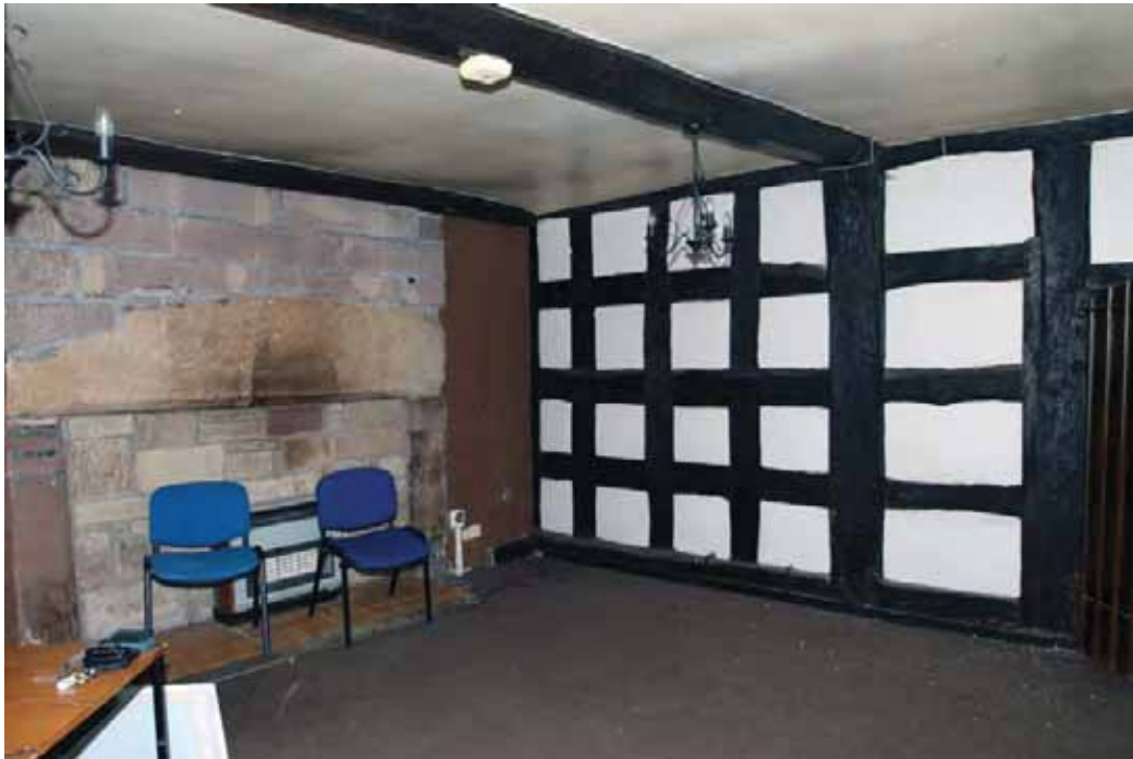
Plate 13. Bay 1, ground floor, living room, viewed from north-east.
