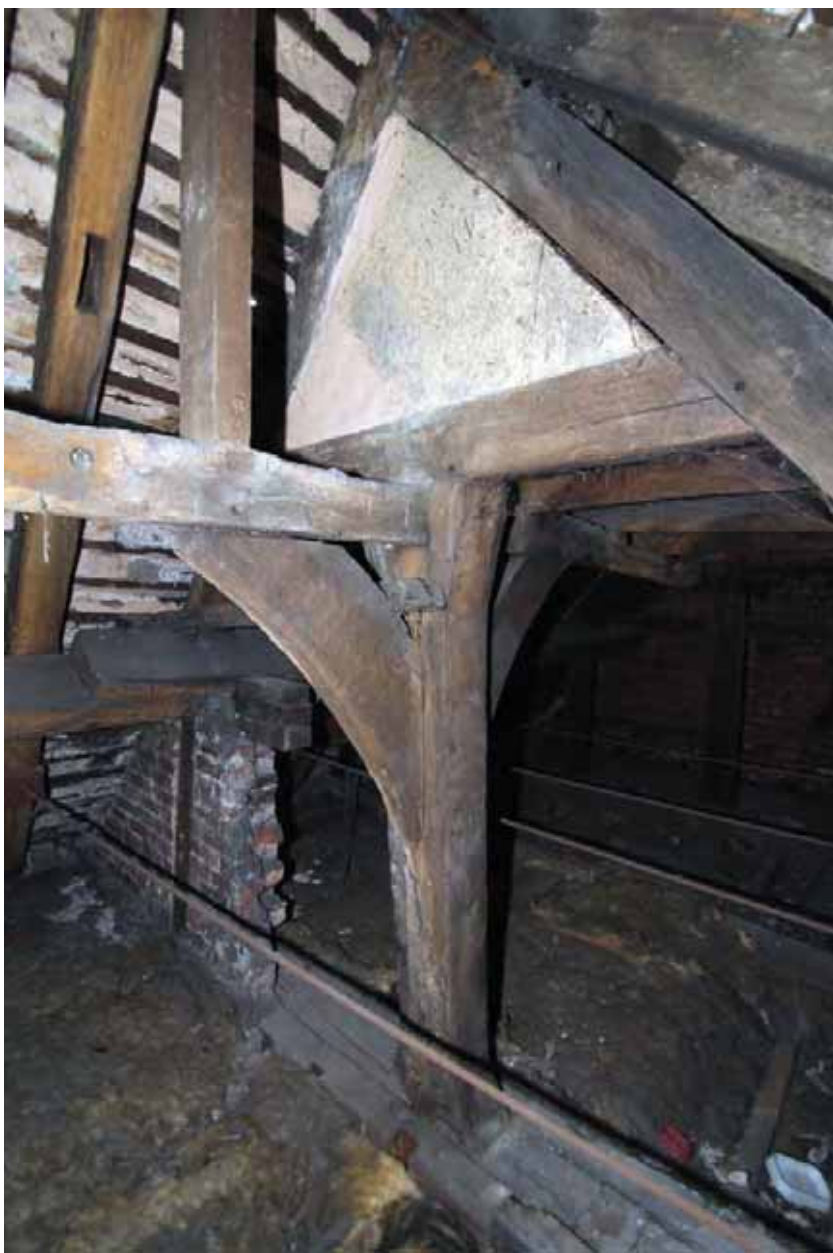
Plate 38. Bay 2, roof space, general view of central crown post truss, viewed from north-west.
