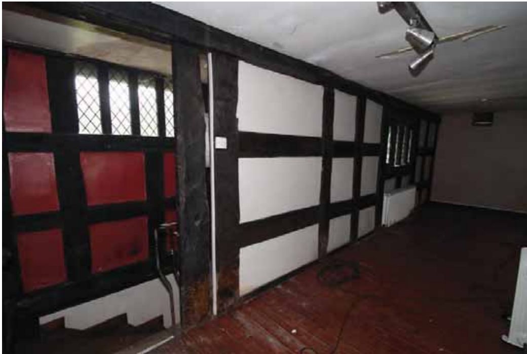
Plate 25. Bays 1 & 2, first floor corridor, viewed from south-east.
