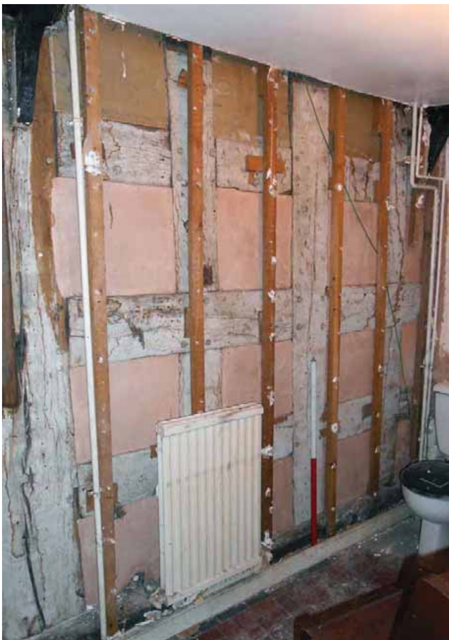
Plate 70. Watching brief, exposed east wall of ground floor W.C.
