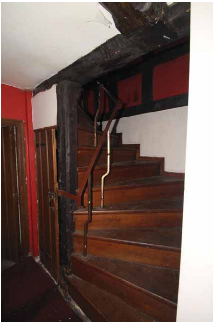
Plate 11. Bay 1, staircase, viewed from north-east.
