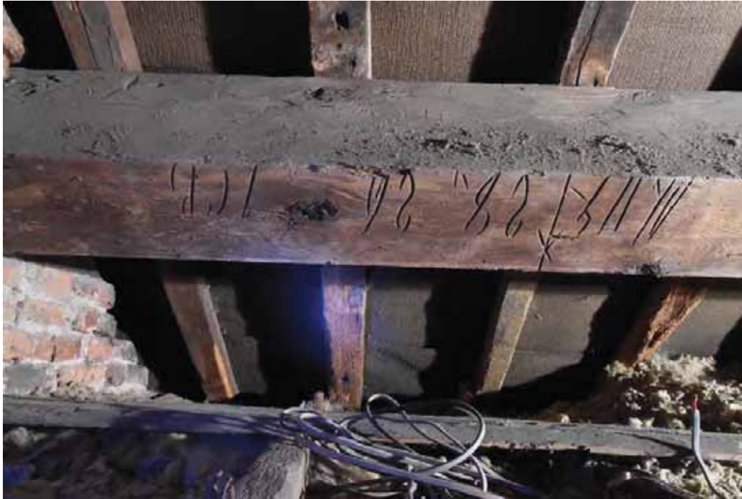
Plate 46. Brick house, bay 4, Baltic timber marks on easternmost purlin.
