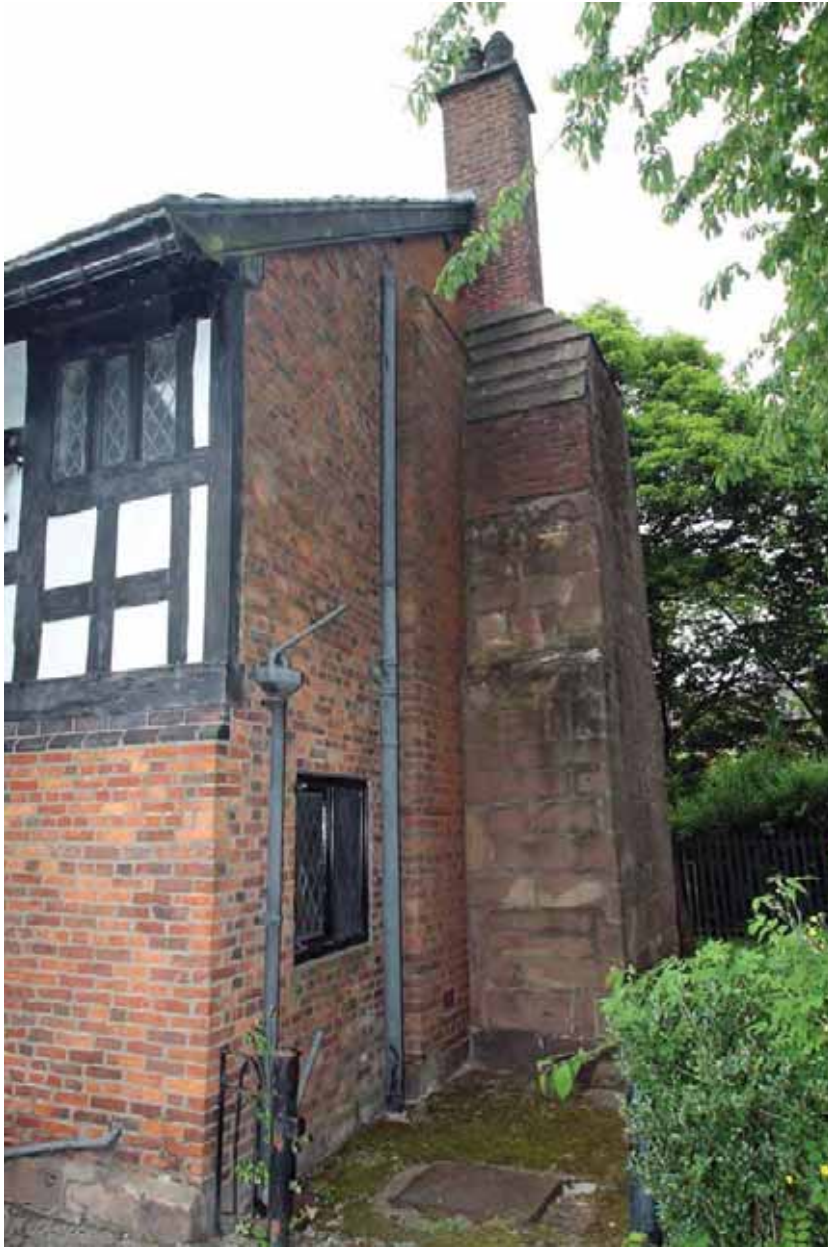
Plate 5. Bay 1, gable end, viewed from south-west.
