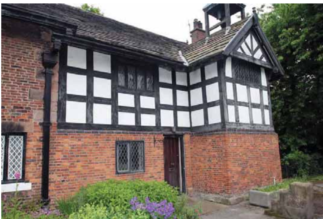
Plate 4. Bays 1 & 2, viewed from north-west.
