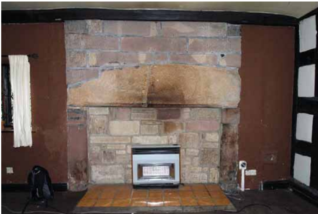
Plate 14. Bay 1, ground floor, fireplace in living room, viewed from north.
