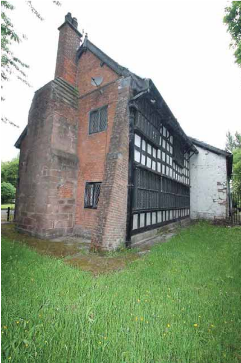
Plate 6. Bay 1, gable end, viewed from south-east.
