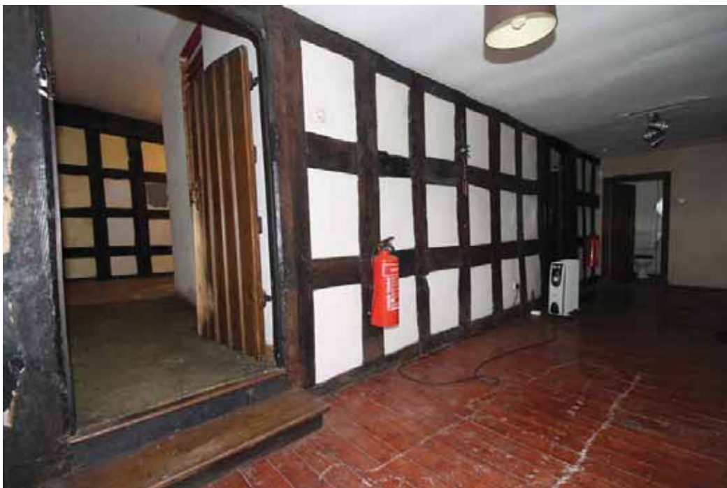
Plate 24. Bays 1 & 2, first floor corridor, viewed from north-west.
