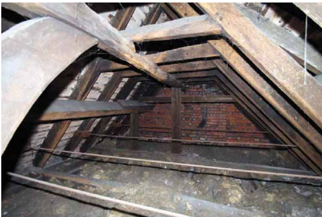
Plate 42. Bay 1, roof space, roof structure to south of central truss (crown plate, collars and rafters), viewed from north-west.
