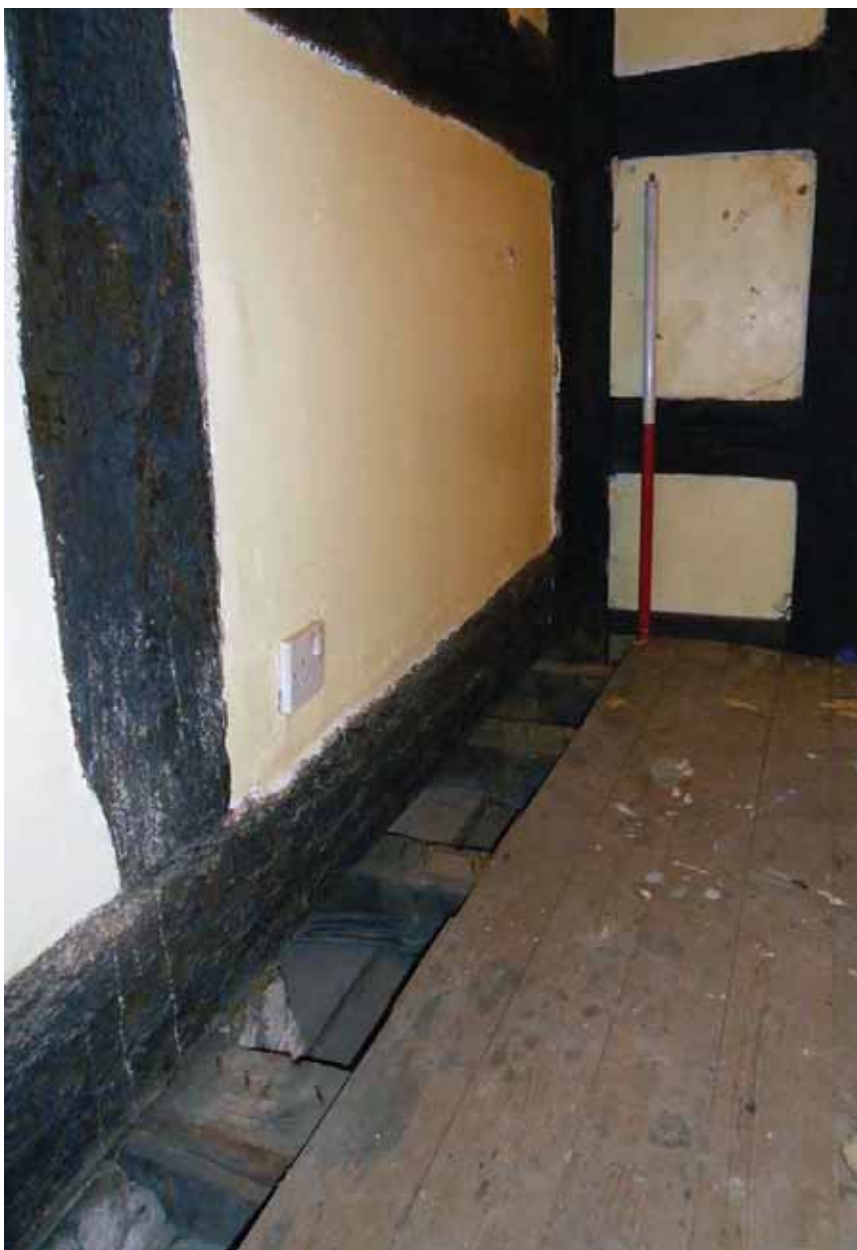
Plate 73. Watching brief, first floor, bedroom 2, north wall, detail of inserted floor.
