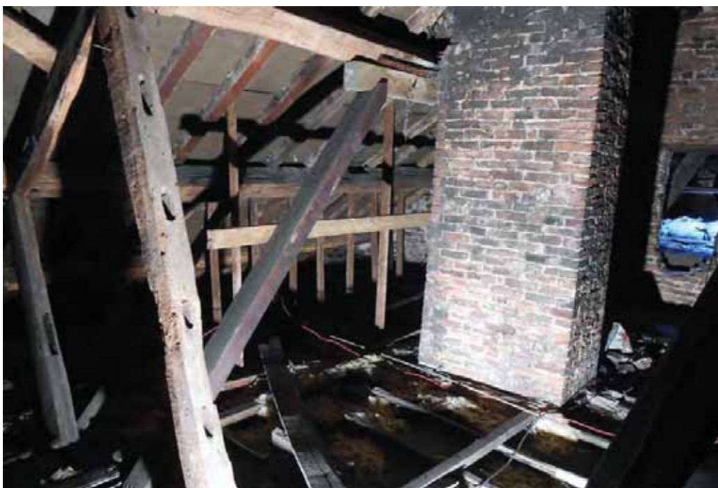
Plate 45. Brick house, bay 3, roof structure and south stack, viewed from north-west.
