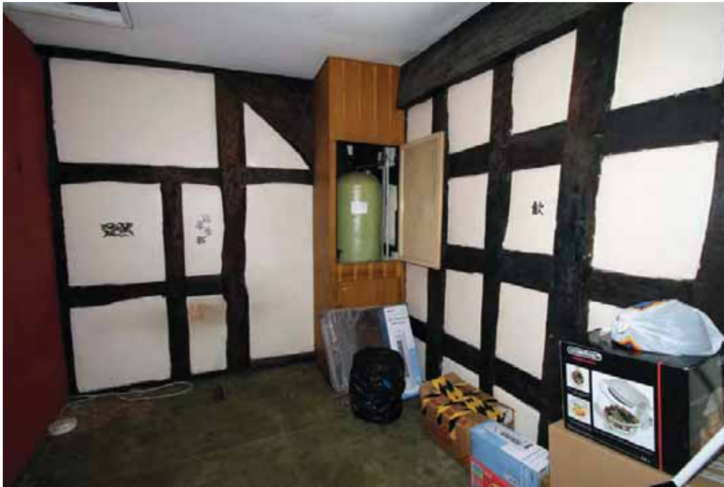
Plate 29. Bay 2, first floor, bedroom 3, viewed from north.
