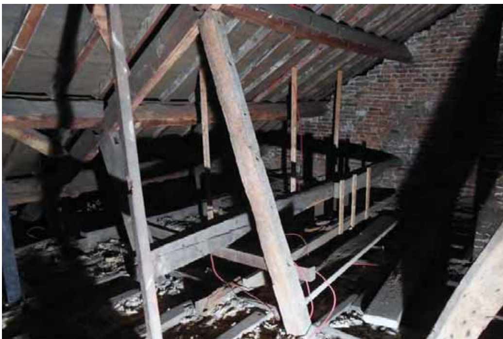
Plate 44. Brick house, roof structure of mainly reused timbers, viewed from south-east.
