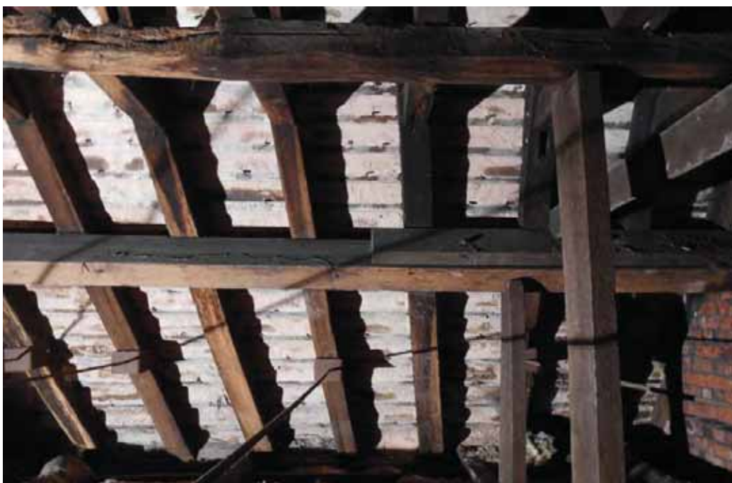
Plate 43. Bay 1, roof space, rafters to south of central truss, viewed from west.
