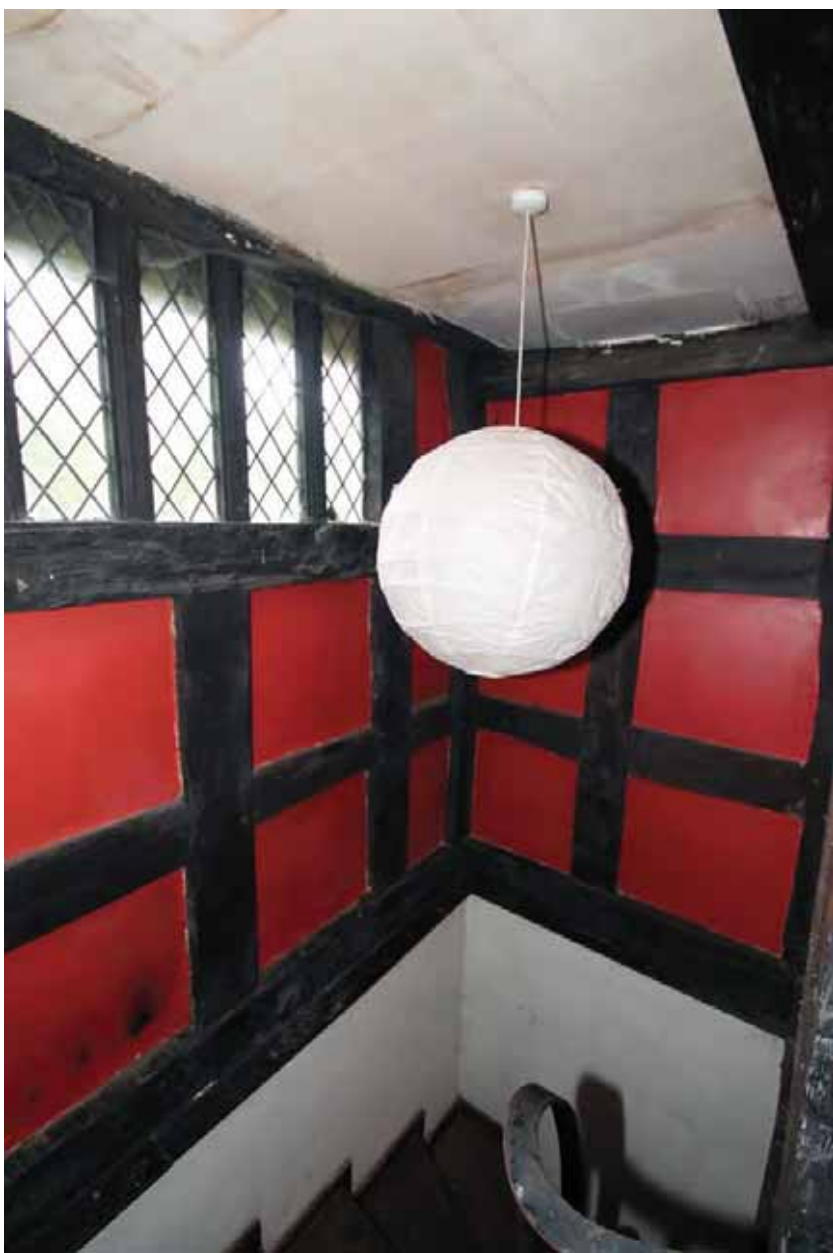
Plate 21. Bay 1, staircase, viewed from south-west.
