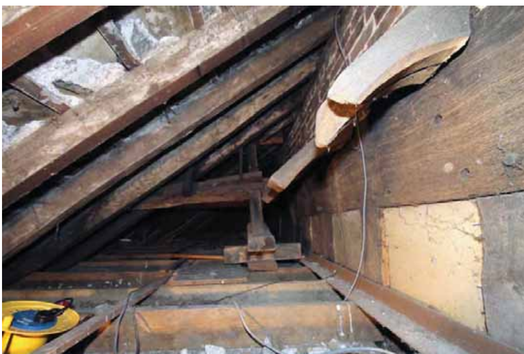
Plate 34. Bay 1, roof space over west corridor, viewed from south, showing original roof rafters at eaves (upper right), with chamfers.
