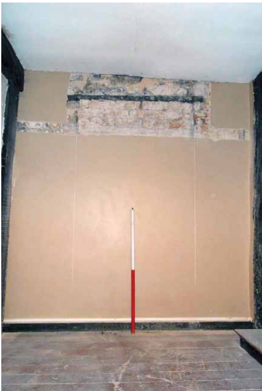
Plate 75. Watching brief, blocked doorway at north end of first floor corridor.
