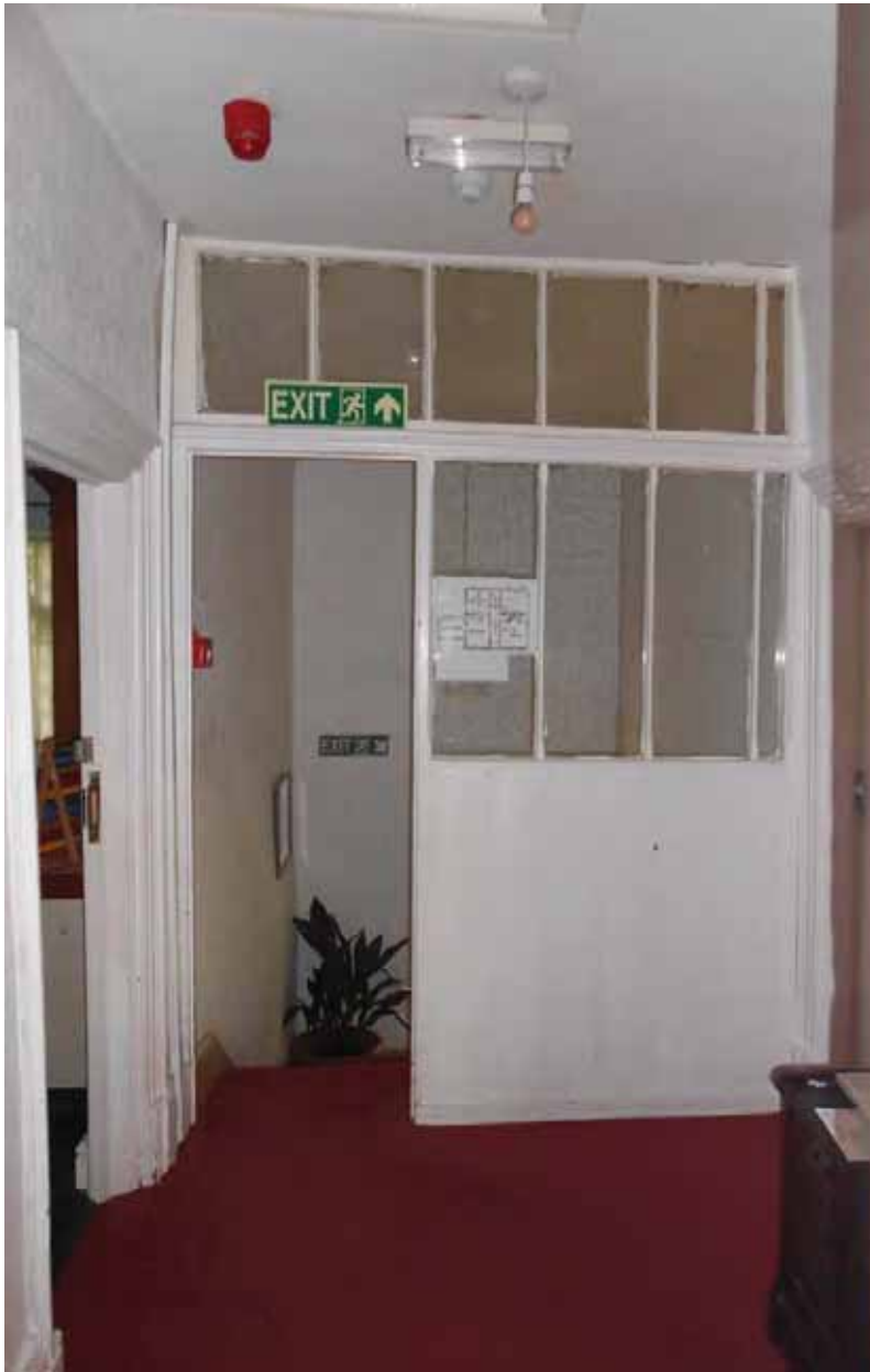
Plate 63. Brick house, first floor, landing and partitions, viewed from west.
