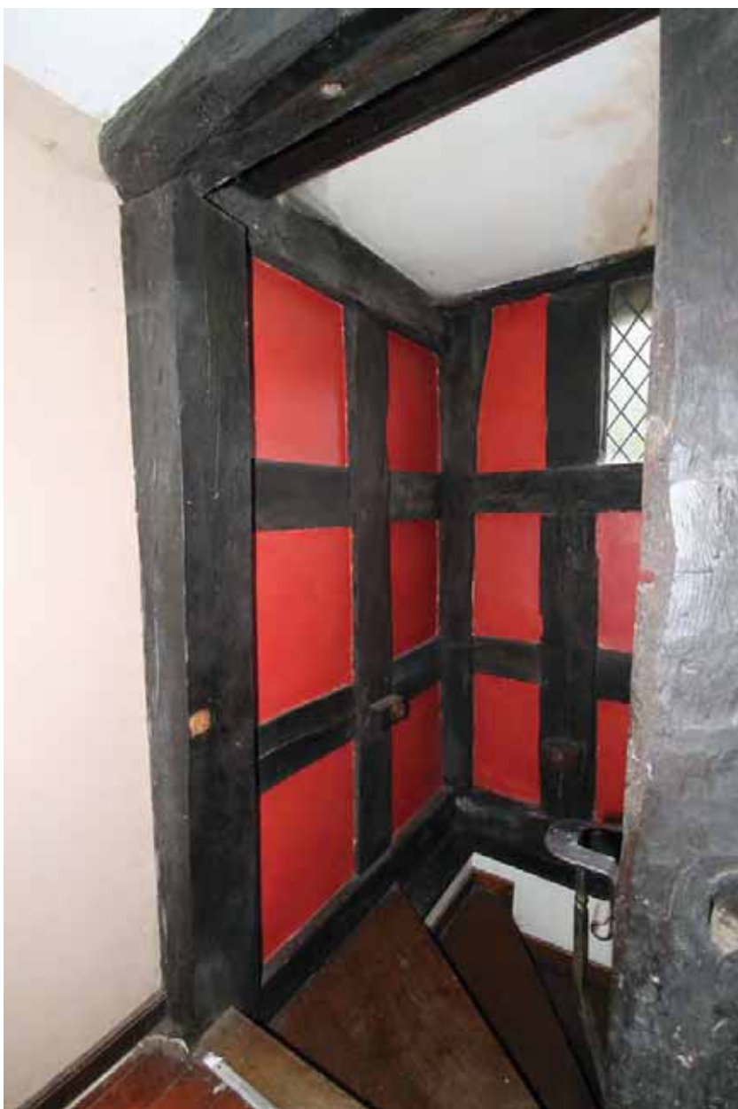
Plate 22. Bay 1, staircase upper entrance, viewed from north-east.
