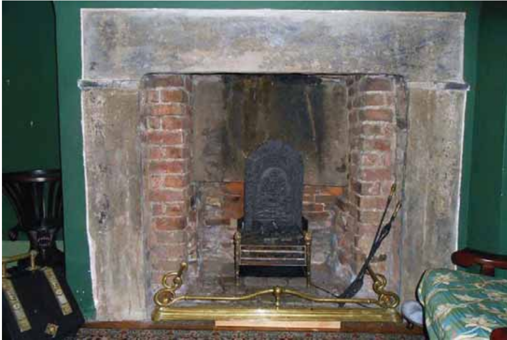
Plate 55. Brick house, ground floor, dining room, inserted fireplace, viewed from west.
