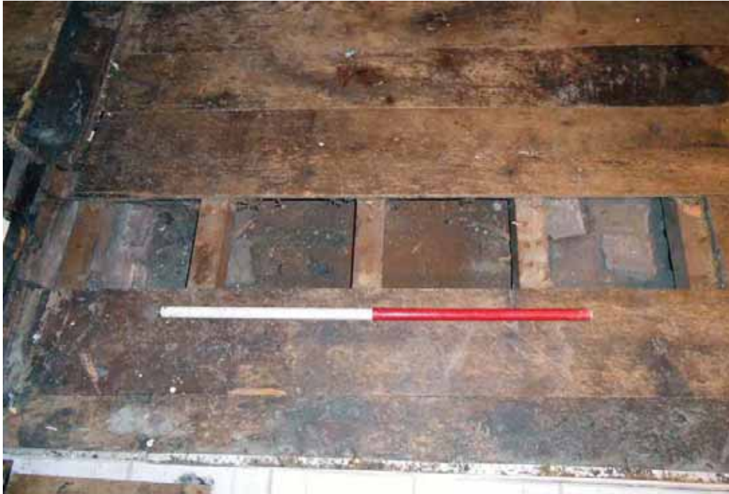
Plate 74. Watching brief, ground floor, bay 2, remains of fireplace below the raised timber floor.
