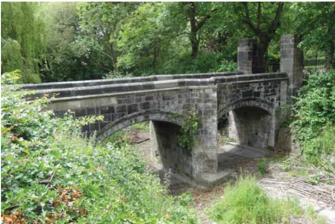
Plate 2: The bridge over the moat viewed from the east.
