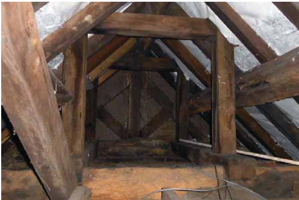
Plate 35. Bay 1, roof space, bellcote and gable pike over stairs, viewed from east.
