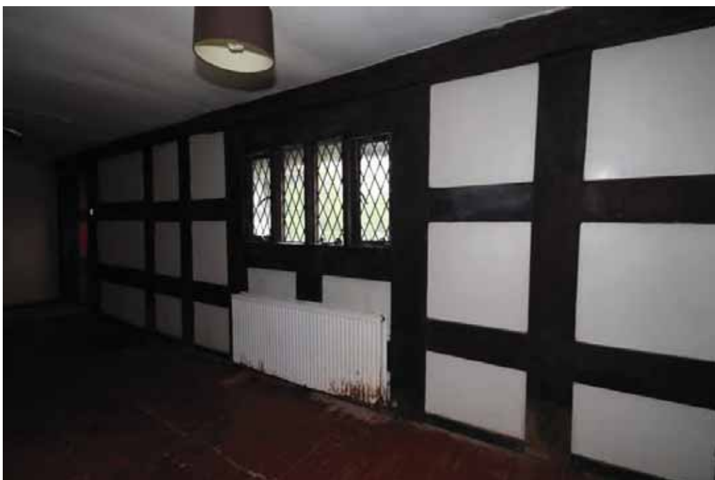
Plate 26. Bays 1 & 2, first floor corridor, viewed from north-east.
