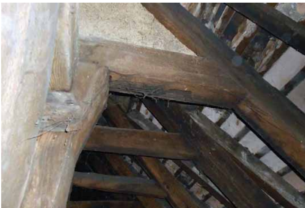
Plate 40. Bay 2, roof space, viewed from north, detail of collar on central truss, showing stave hole in soffit.
