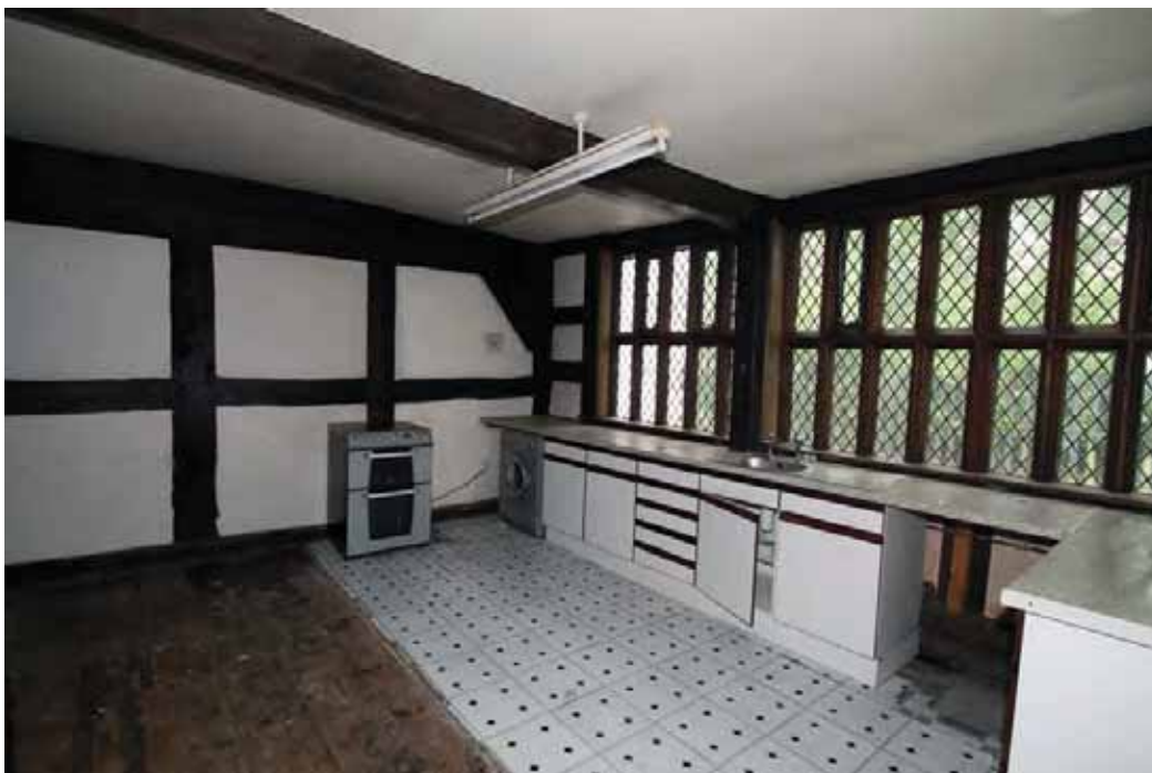
Plate 16. Bay 2, ground floor, kitchen, viewed from south-west.
