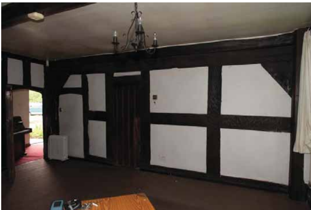
Plate 19. Bay 1, ground floor, living room, viewed from south-east.
