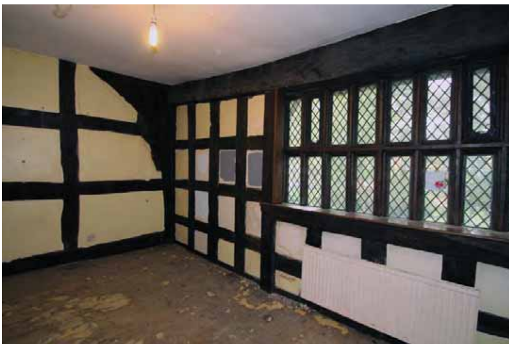
Plate 33. Bay 2, first floor, bedroom 2, viewed from south-west.
