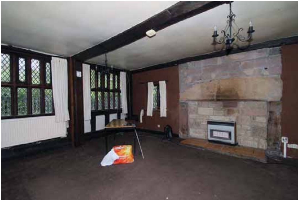
Plate 15. Bay 1, ground floor, living room, viewed from north-west.
