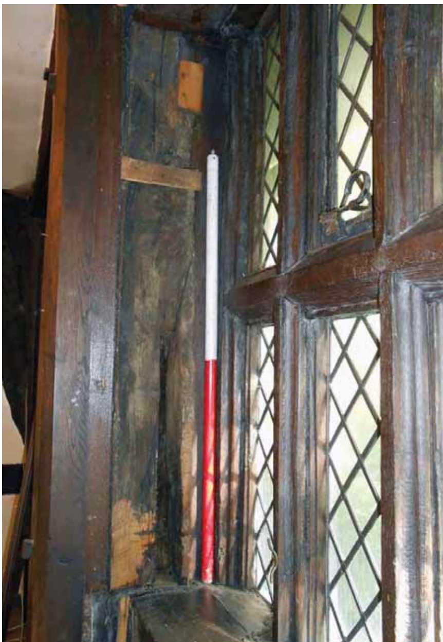
Plate 71. Watching brief, first floor, bedroom 1, east wall, intermediate post, viewed from south.
