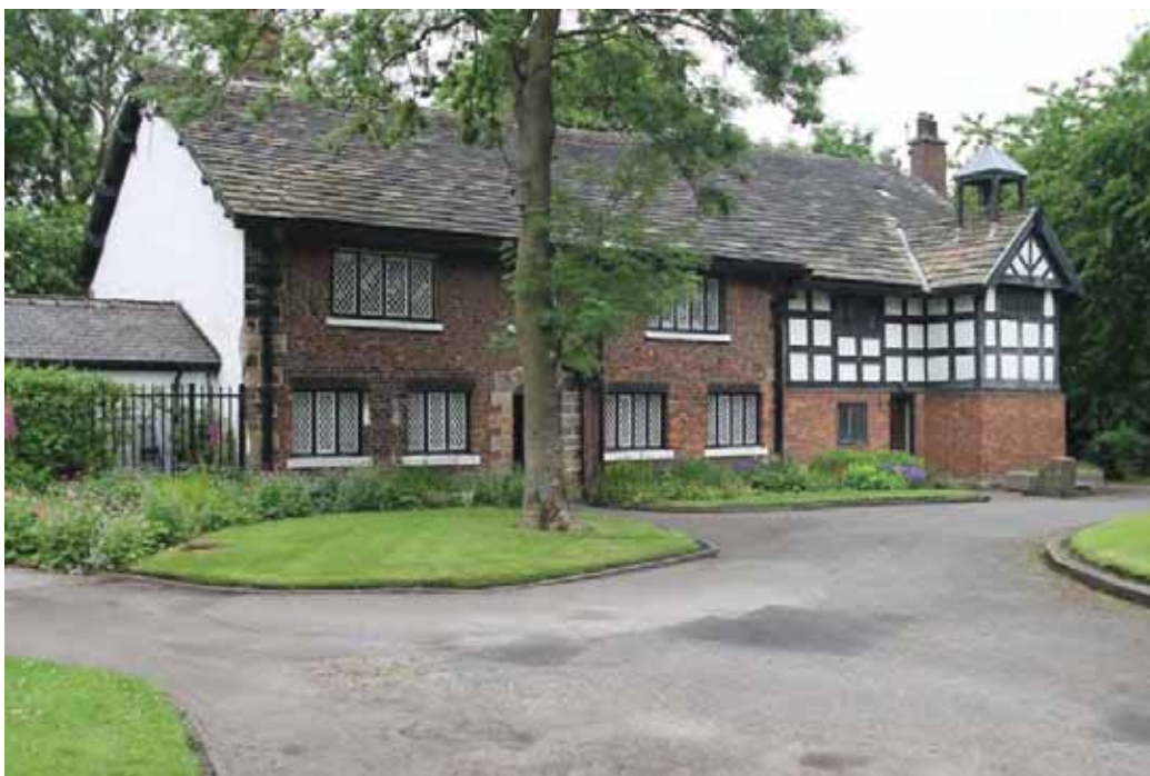
Plate 3. Building viewed from north-west.
