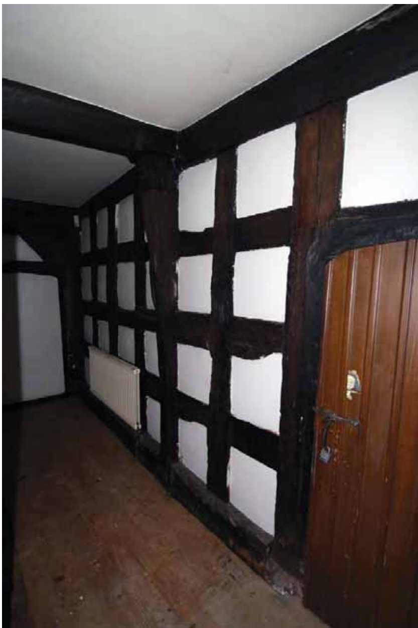
Plate 20. Bay 1, ground floor, kitchen, west side, viewed from north.
