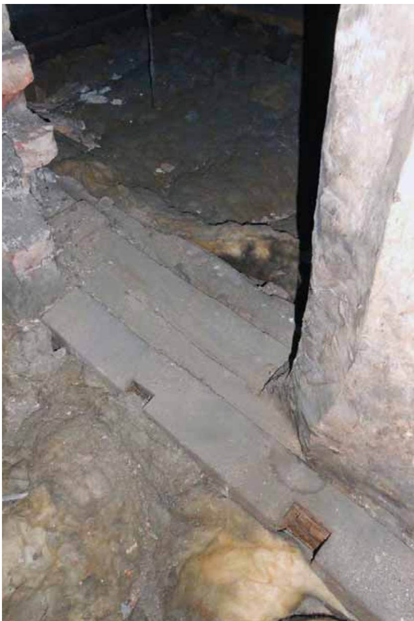
Plate 41. Bay 2, roof space, viewed from north-west, detail of collar (central truss) showing stave groove.
