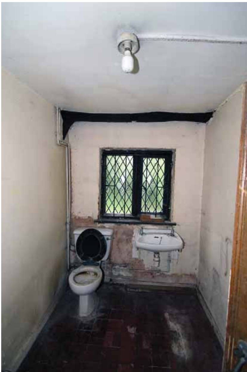
Plate 12. Bay 1, ground floor, WC viewed from north.
