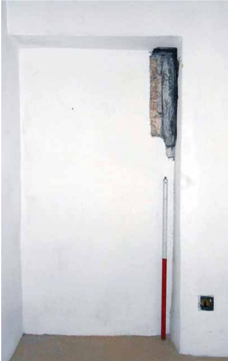
Plate 77. Watching brief, blocked doorway between larder and dining room, in brick house.
