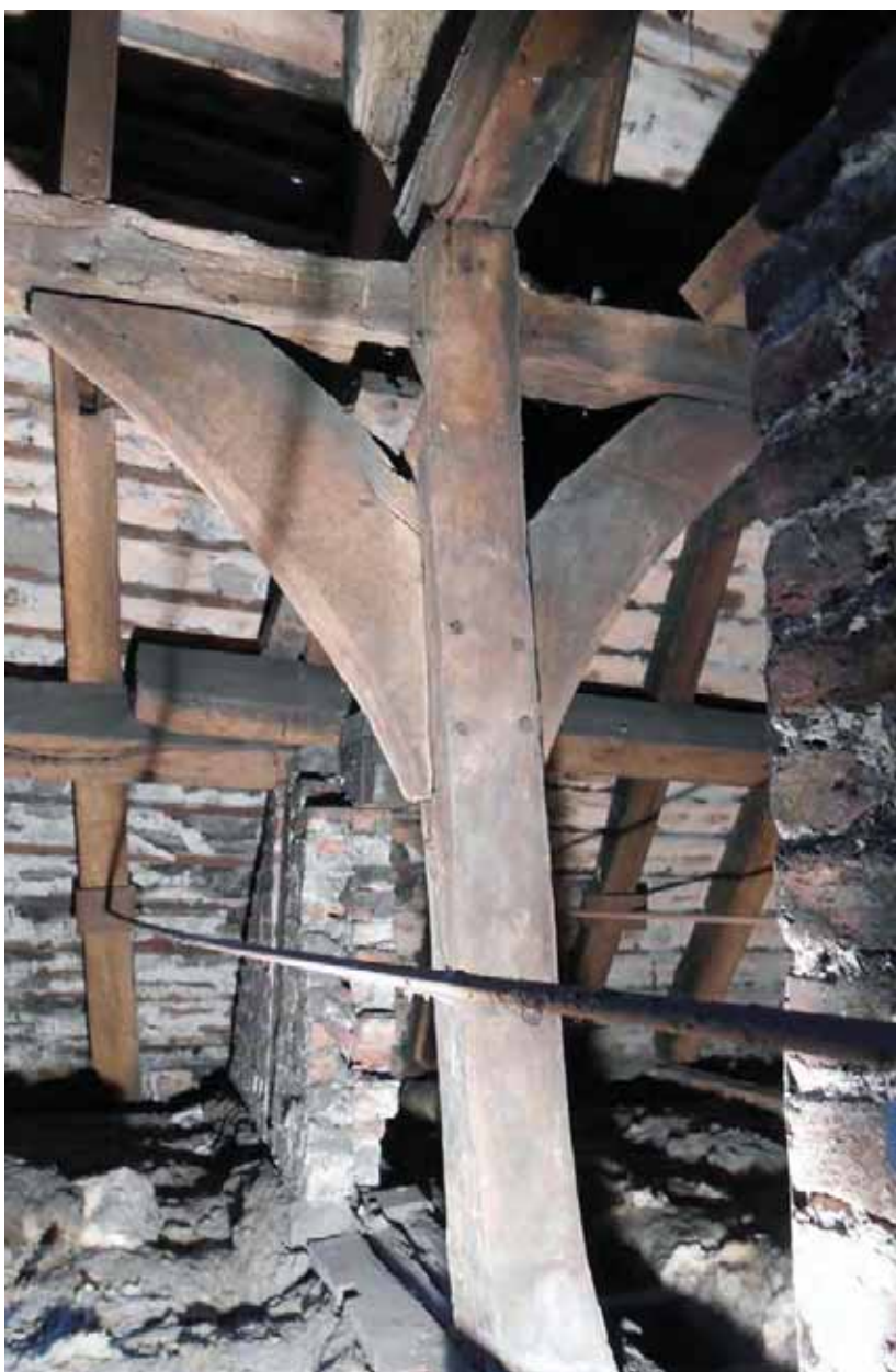
Plate 39. Bay 2, roof space, central crown post, viewed from west.
