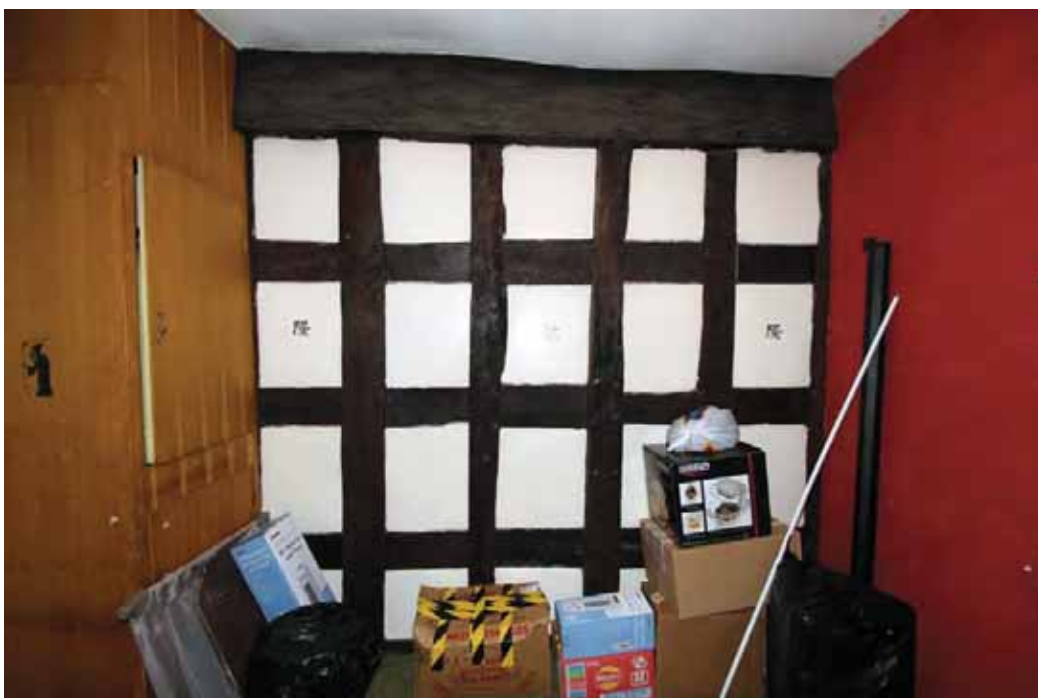
Plate 30. Bay 2, first floor, bedroom 3, viewed from east.
