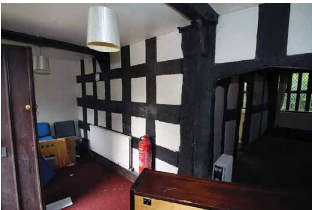
Plate 10. Bays 1 & 2, ground floor, corridor, viewed from south-west.
