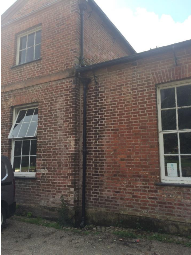
Photo 5 – Existing hopper arrangement.
