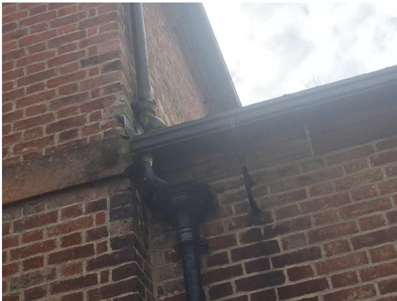
Photo 6 – Existing hopper arrangement.
