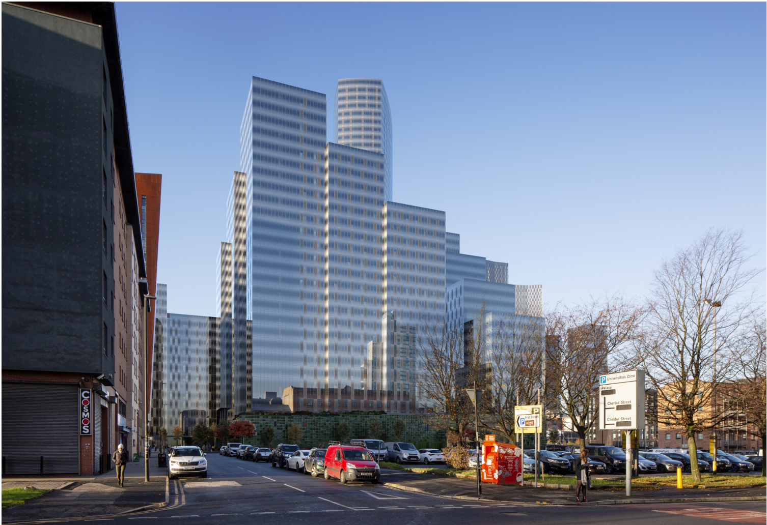
View West along Chester Street
