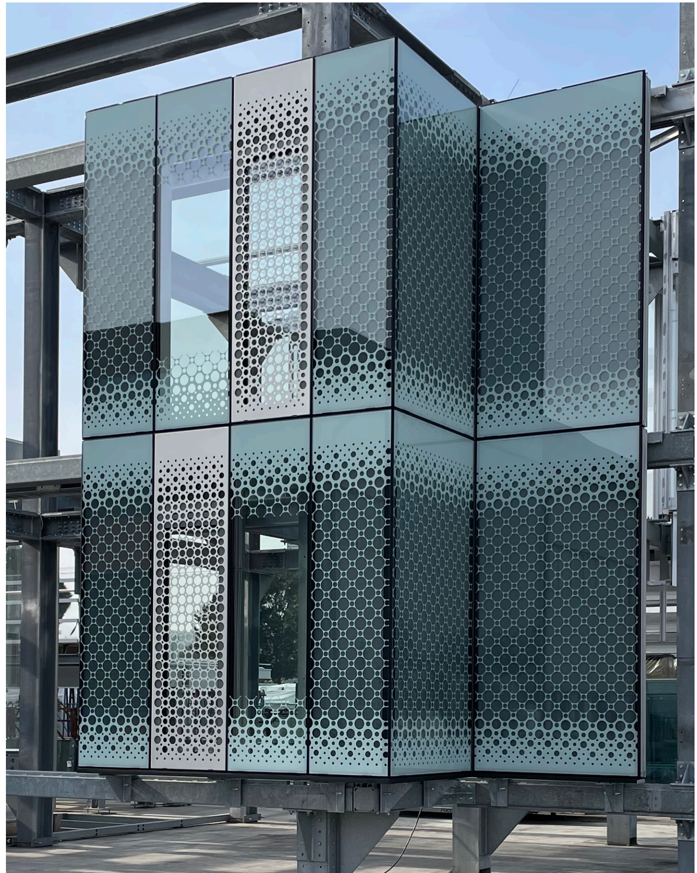
VISUAL MOCK UP - BUILDING A & B Photographed 12.10.2022
