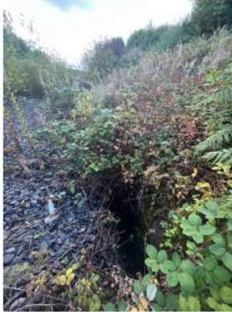
Fig. 2: Incoming pipe from the Showman's Guild direction @ CH430, with a significant flow of water. This water appears clear compared to the water in the channel.
