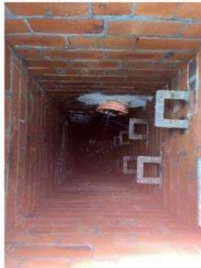
Fig. 14: 6m deep manhole which has water running through it. This manhole looks much more modern than the rest. Dye was put into the water in this chamber which was then seen on Hargreaves Street. We tried to sonde from this chamber but hit an obstruction. We suspect due to no water build up and the level difference between this chamber and Hargreaves Street that there is a drop shaft on this section.
