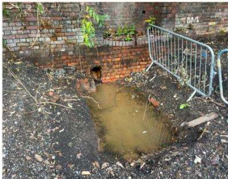
Fig. 8: A 200mm ceramic pipe coming from behind Honey Street wall @CH100. This pipe has had a constant trickle of water coming out since it was discovered.
