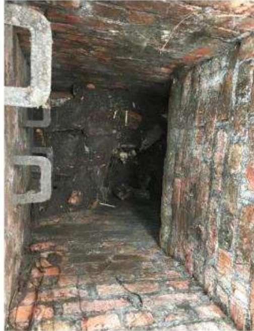
Fig. 14: 6m deep manhole which has water running through it. This manhole looks much more modern than the rest. Dye was put into the water in this chamber which was then seen on Hargreaves Street. We tried to sonde from this chamber but hit an obstruction. We suspect due to no water build up and the level difference between this chamber and Hargreaves Street that there is a drop shaft on this section.
