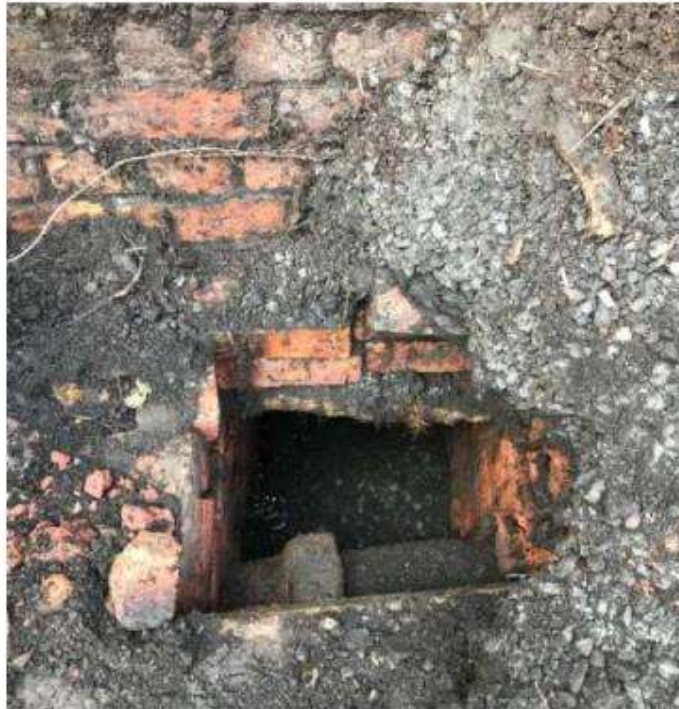
Fig. 6: In this location we observed the culvert running parallel to Honey Street retaining wall passing over a second culvert of similar construction, coming from under Honey Street Wall. The first culvert continues along the wall and the second one continues to a nearby chamber. Water has been observed to be running through this second run. These two runs eventually converge in the manhole that was found with a Kelly block in it.
