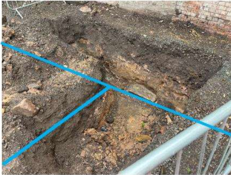
Fig. 12: Chamber at the bottom of the haul road. Picture taken on the inside, with the concrete 'V' shapes coming from the 'T' in figure 11 and a derelict and dry pipe running along the plateau.
