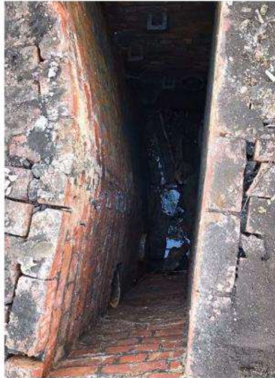
Fig. 8: A 200mm ceramic pipe coming from behind Honey Street wall @CH100. This pipe has had a constant trickle of water coming out since it was discovered.
