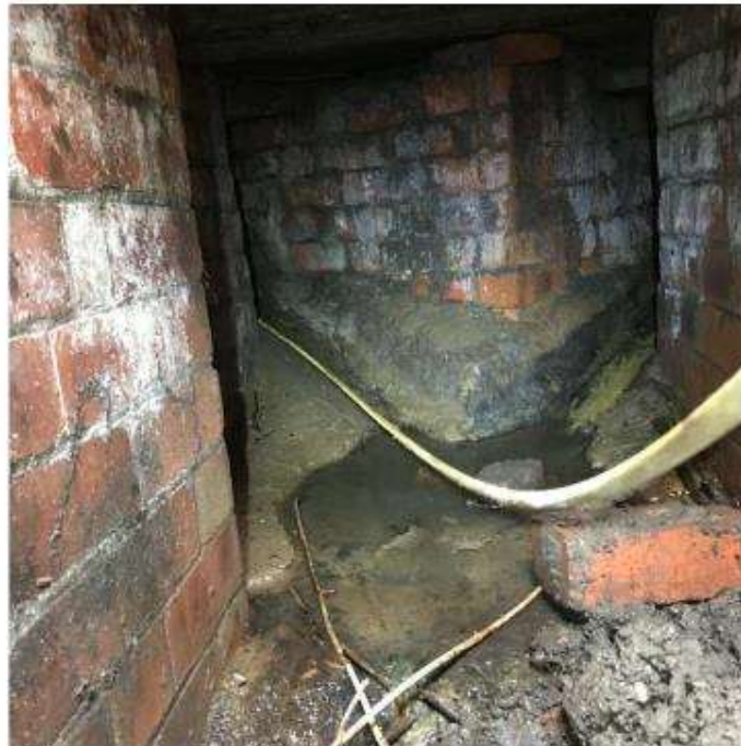
Fig. 12: Chamber at the bottom of the haul road. Picture taken on the inside, with the concrete 'V' shapes coming from the 'T' in figure 11 and a derelict and dry pipe running along the plateau.
