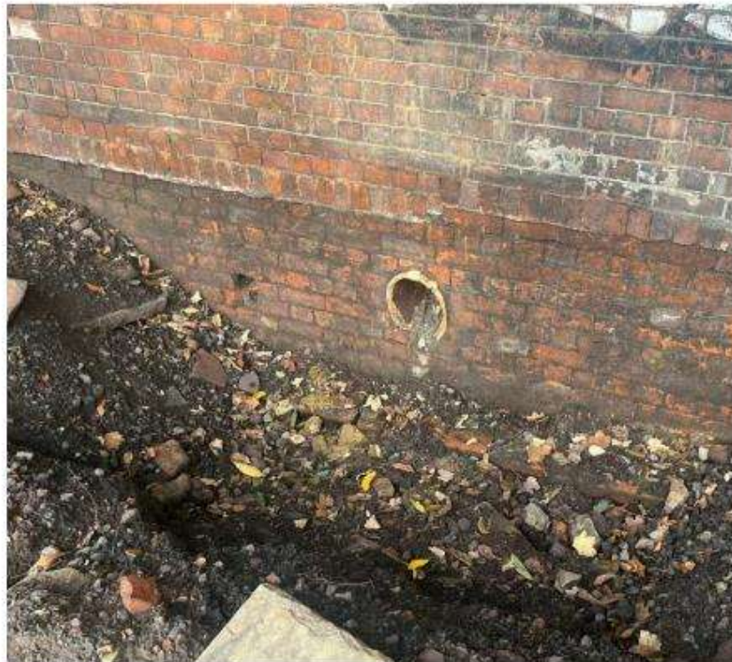
Fig. 10: A second 200mm pipe coming in from behind the wall, this one is dry.
