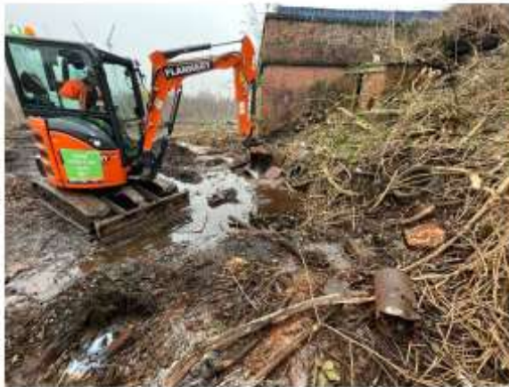
C. Area where water emerges from existing ground
