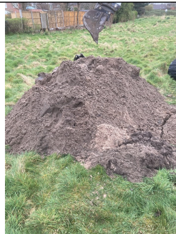
Trial Pit 101 Spoil
