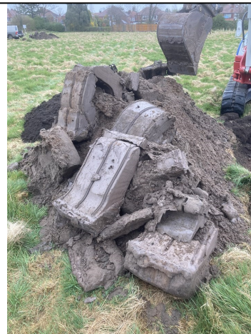
Trial Pit 107 Spoil
