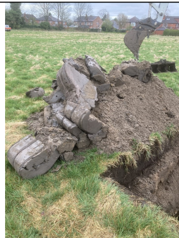
Trial Pit 108 Spoil
