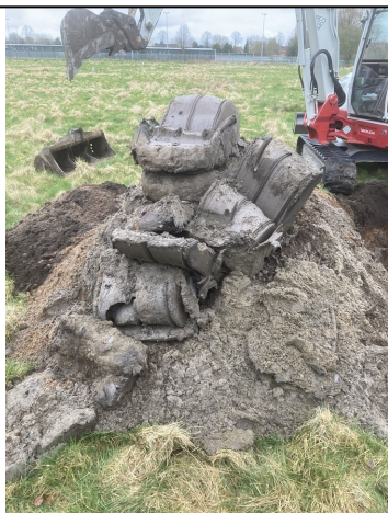
Trial Pit 112 Spoil
