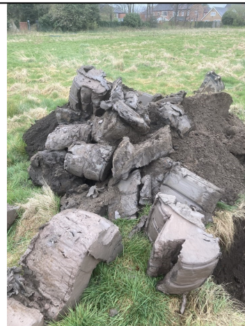
Trial Pit 109 Spoil
