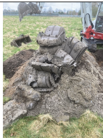
Trial Pit 112 Spoil
