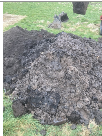
Trial Pit 110 Spoil
