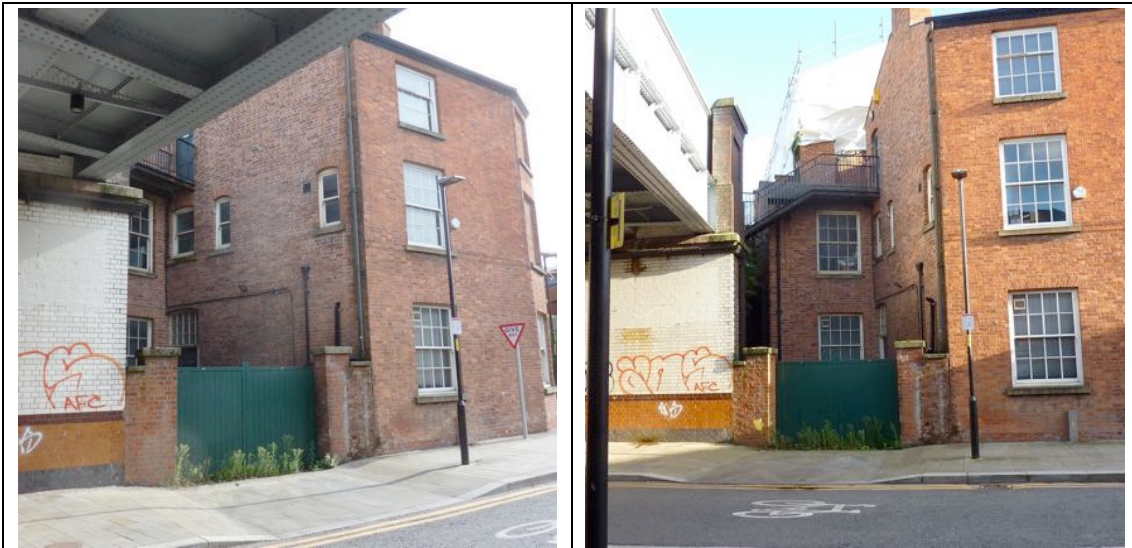
Photos of the rear elevation showing the current wall and gates to the yard.
