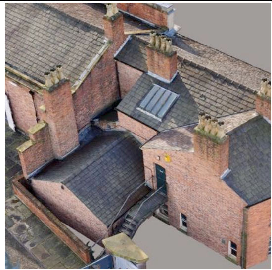
Photos showing the set back in the north roof pitch that we propose to infill so that the drainage of those roofs is not concentrated on the back gutter of the chimney stack
