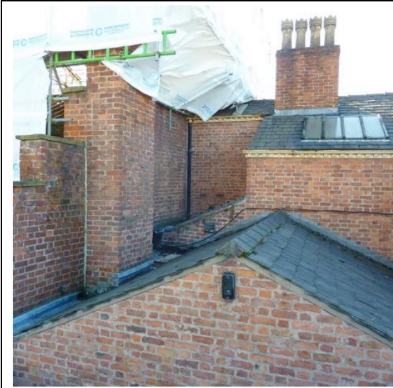
Photos showing the set back in the north roof pitch that we propose to infill so that the drainage of those roofs is not concentrated on the back gutter of the chimney stack
