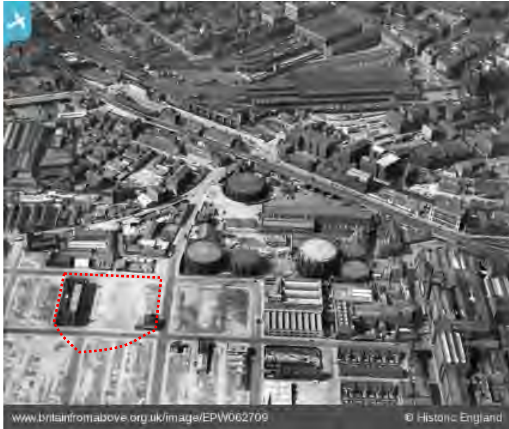
Figure 2.8: Aerial photography dating from 1939 showing the cleared area to the south of River Street, including the Site (red line shows approximate location of the Site). Only the Duke Street School and The Globe Inn public house remained within the area of the Site. Much of the terraced housing in the wider area had also been cleared.
