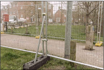
Example of herras fencing stabilisation measures
