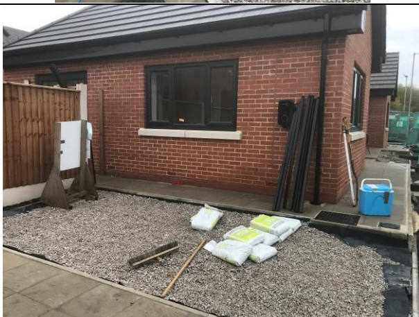
Photograph 3: View showing to front of plots.
