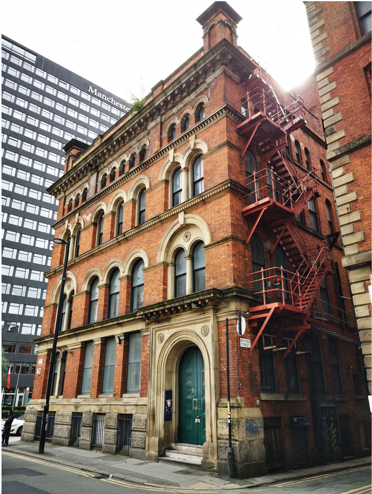
CHARLOTTE STREET AND REYNER STREET ELEVATIONS. (Image taken prior to current repair works)
