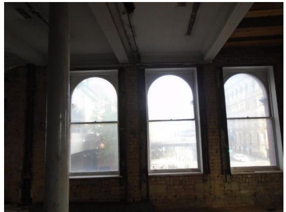
Typical sash windows (previously repaired). Include allowance for easing works.
