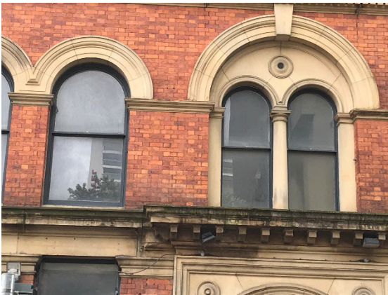
Typical sash windows for redecoration.
