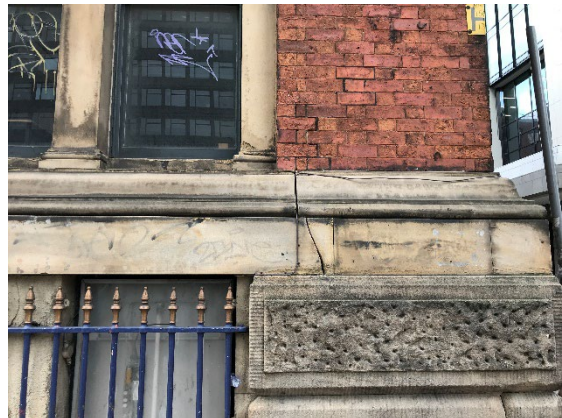
Typical indent repair to stone coursing.
