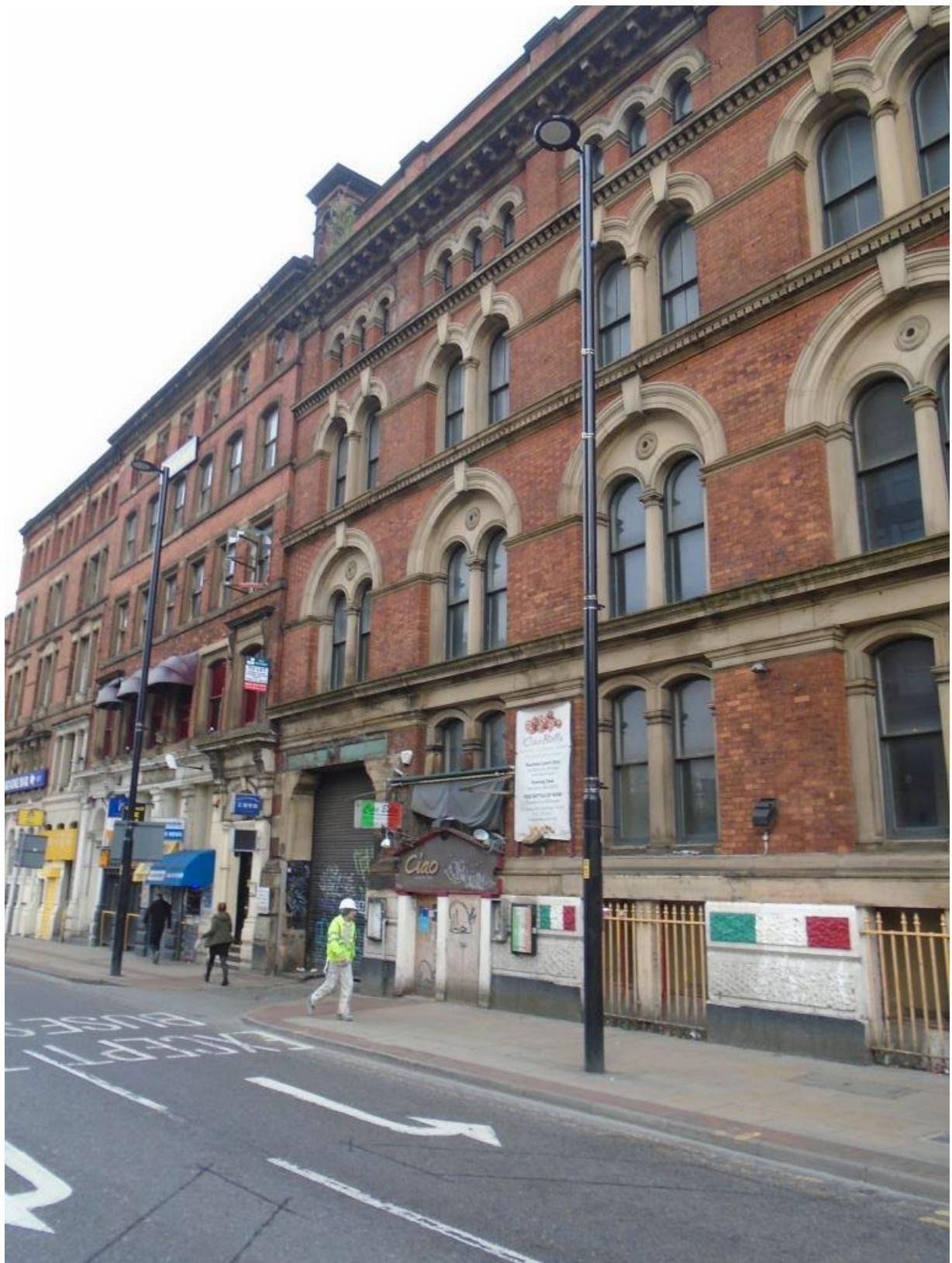
PORTLAND STREET ELEVATION. (Image taken prior to current repair works.)
