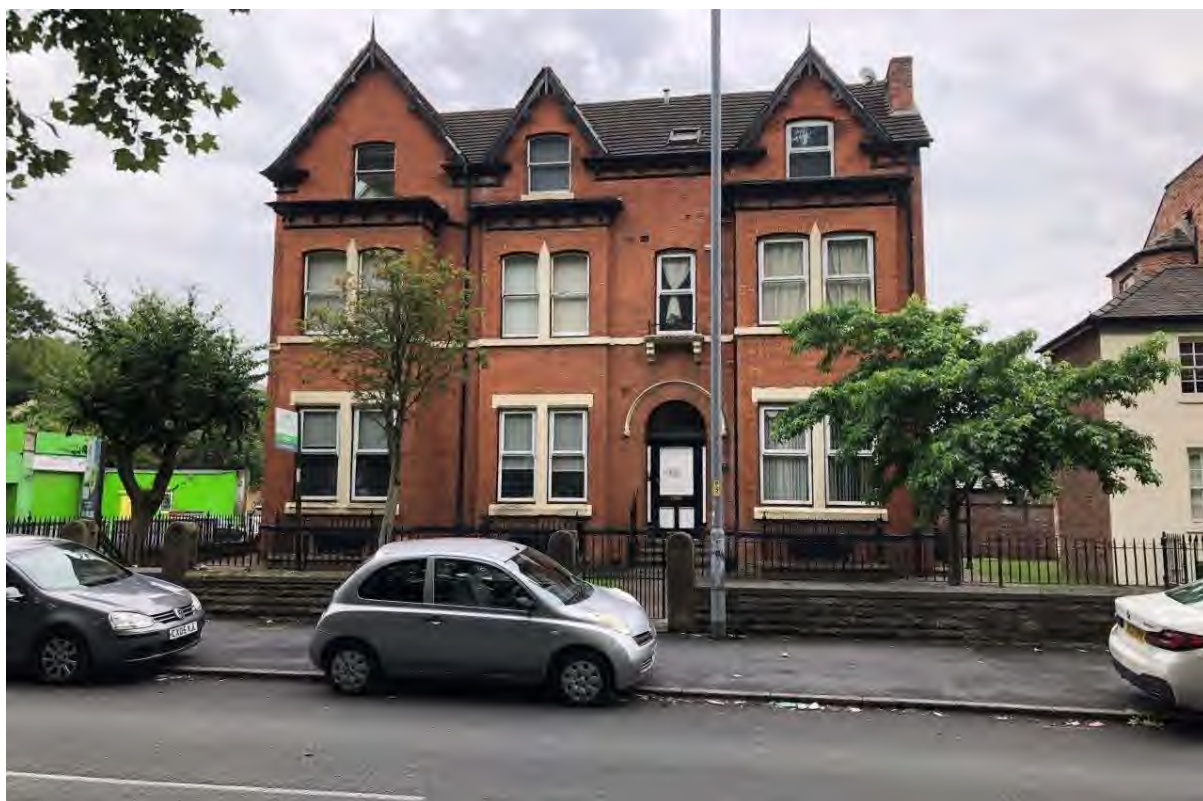
Plate 5: Sightline to the south from Moss Lane East highlighting the front (north-facing) elevation of 470-472 Moss Lane East
