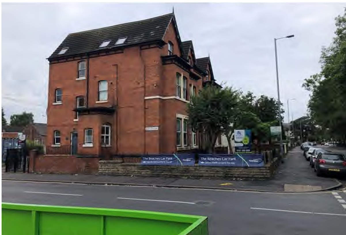
Plate 8: Sightline to the south-west from Heald Place highlighting the east-facing elevation of 470-472 Moss Lane East
