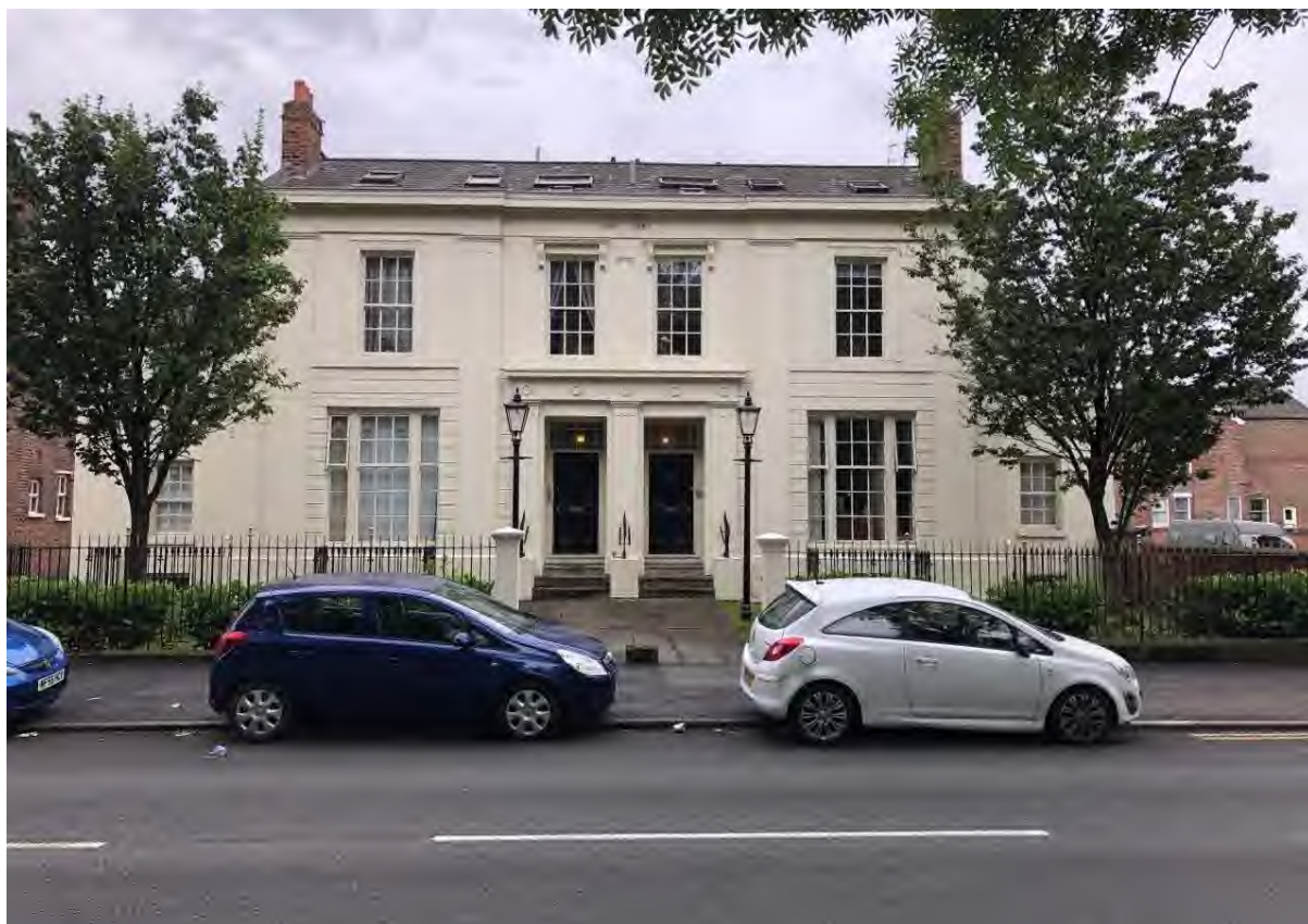
Plate 3: Sightline to the south from Moss Lane East highlighting the front (north-facing) elevation of 466-468 Moss Lane East
