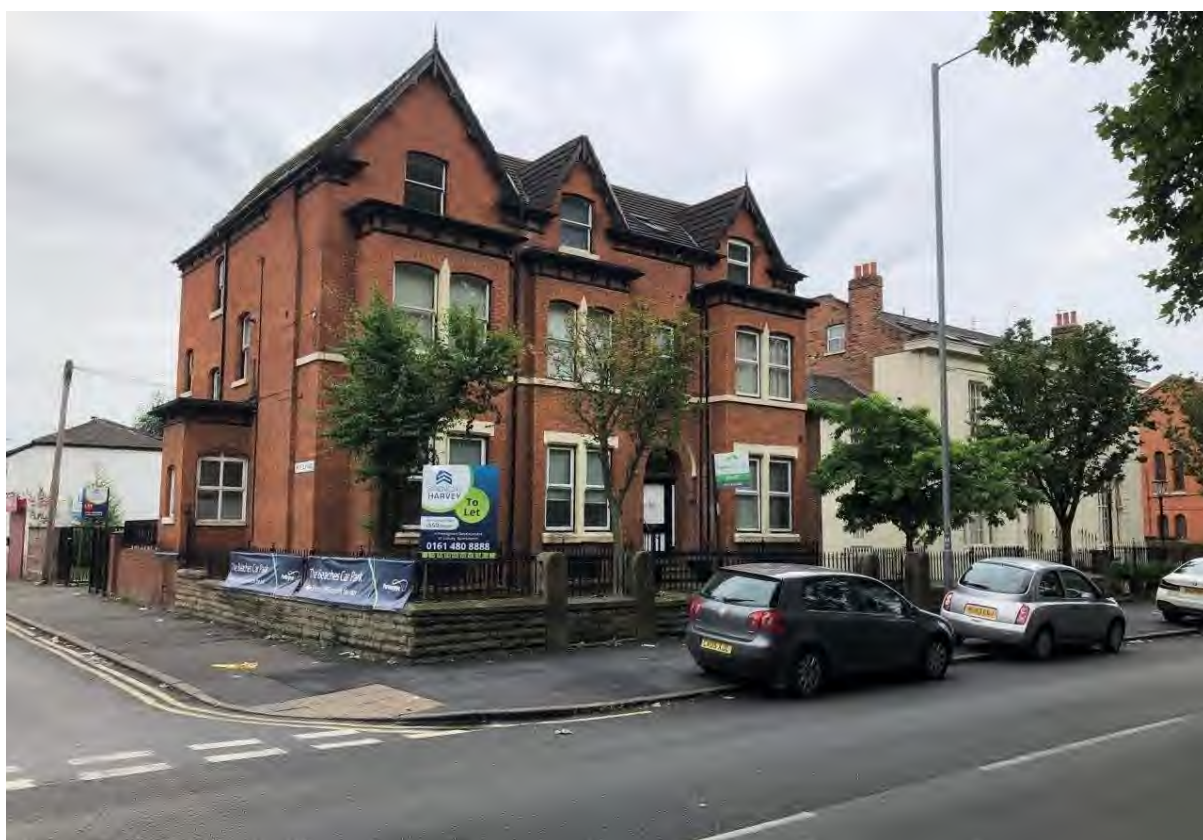
Plate 6: Sightline to the south-west from Moss Lane East highlighting the front (north-facing) elevation of 470-472 Moss Lane East and the projecting porch on the east-facing elevation with doorway stopped up and repurposed as a window
