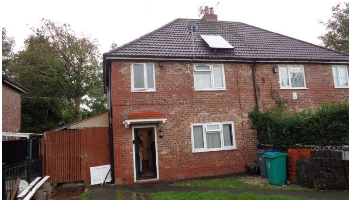
Front Elevation of Application Property.
