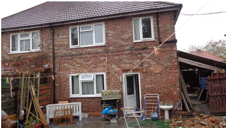
Rear extension to Application Property.
