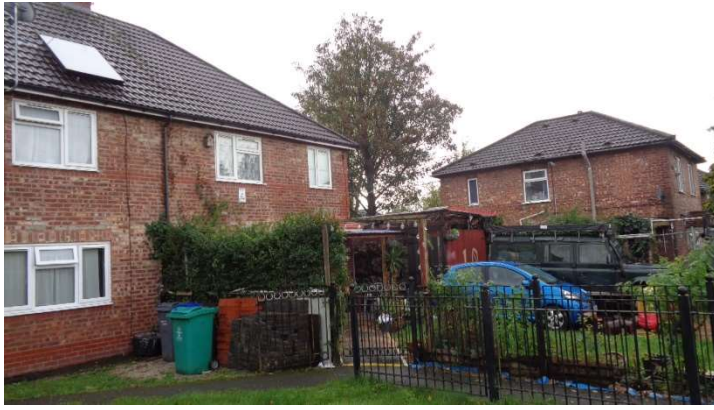
Nr 10 adjacent to Application Property.
