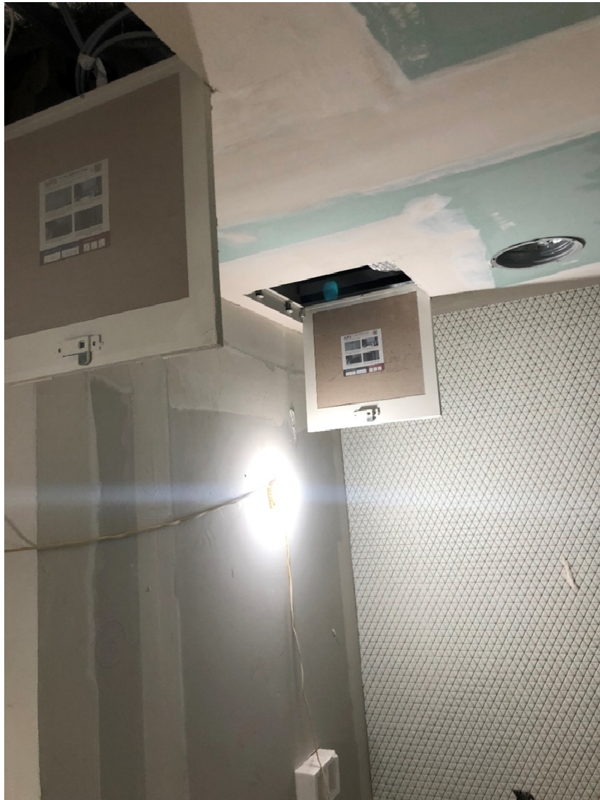
Figure 1-11 - Example of access hatches photographed during construction
