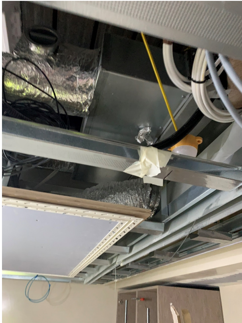
Figure 1-10 - FCU and ductwork photographed during construction
