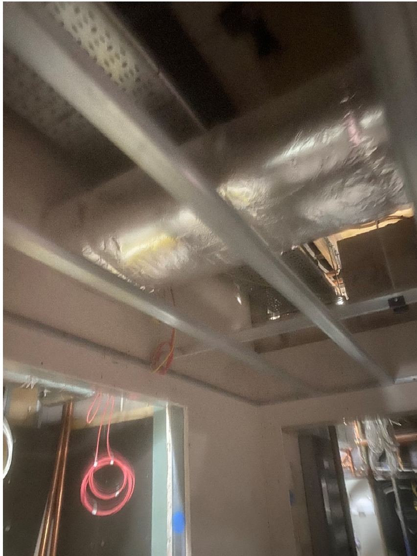
Figure 1-8 – Example of lagged ductwork photographed during construction
