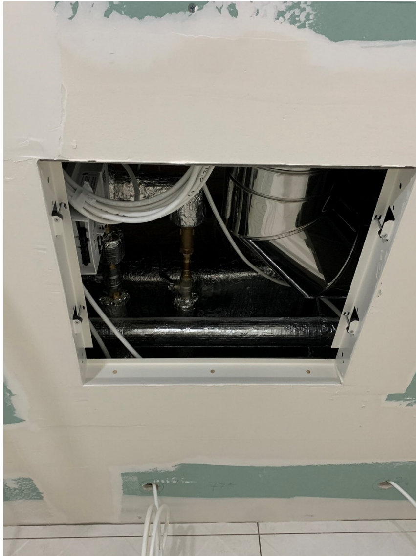
Figure 1-9 - Example of access hatch photographed during construction
