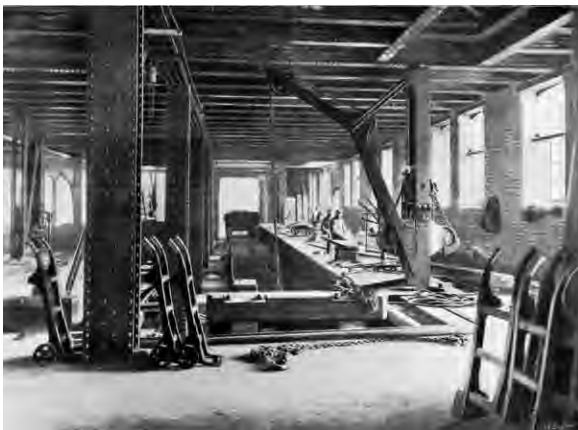
Figure 30 – A photograph taken looking south along the high level station of the newly completed warehouse in 1898, showing the original track beds and teagles.
