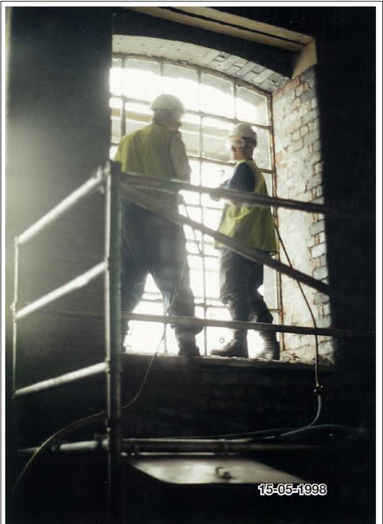
Figure 26: Original window pictured up close during late 1990s works.
