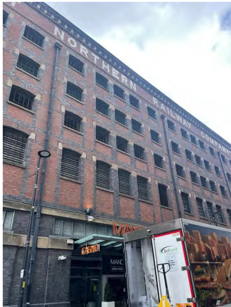
Figure 46 – The west elevation of the Great Northern Warehouse from Watson Street.
