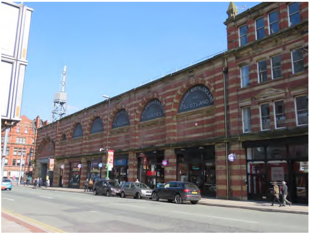
Figure 61 – The northern end of the terrace, showing the original destination lettering and former goods yard entrance to the left.
