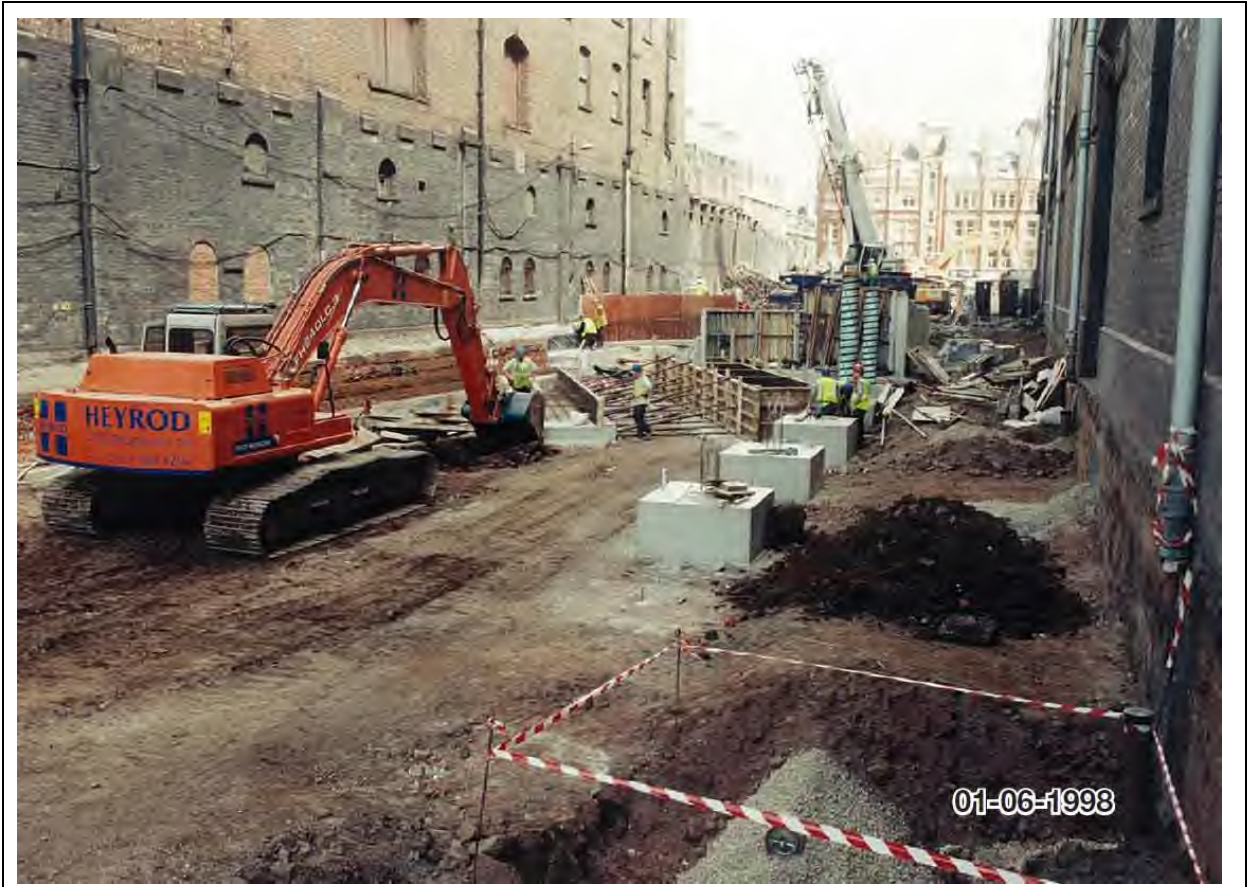
Figure 24: Looking south with views of the eastern elevation of the Goods Warehouse.
