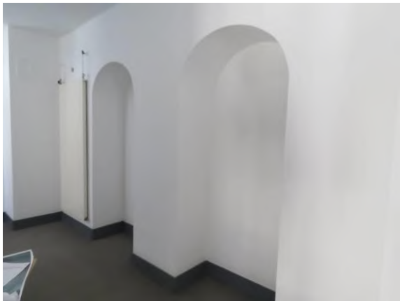
Figure 67 – Blocked window openings.
