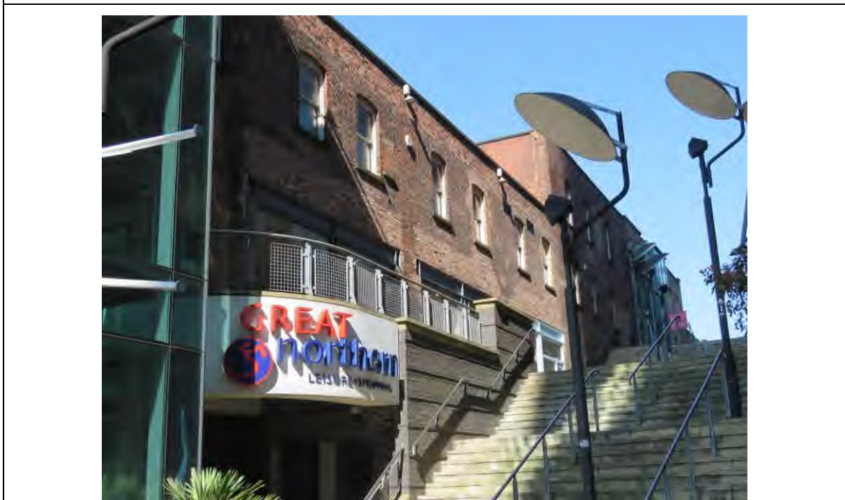
Figure 64 – Looking up to the c2000 inserted walkway.
