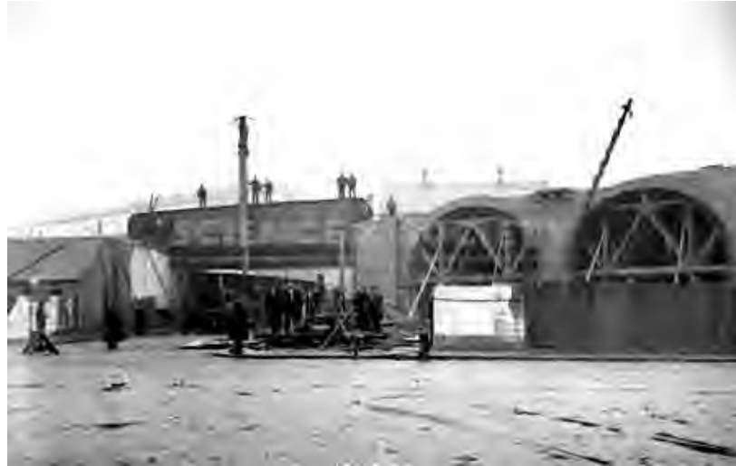
Figure 13 – The construction of the Great Bridgewater Street viaduct during construction in mid-1897. Note the roof and two roof cowls of the 1801 Wesleyan Methodist Chapel on Great Bridgewater Street.
