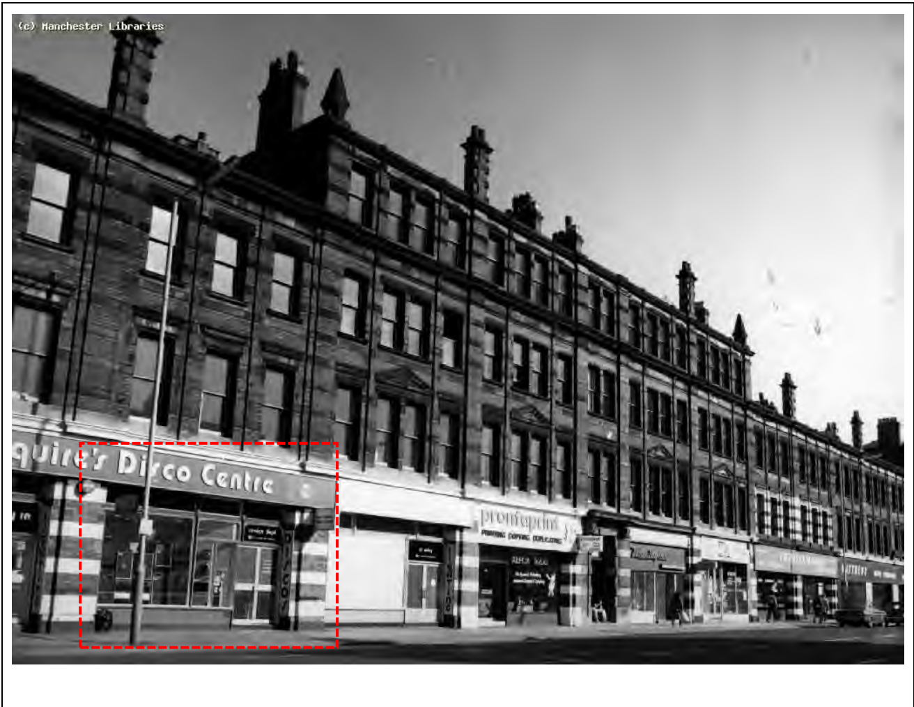
Figure 43: Deansgate c.1990 – Units 235 (left) to Unit 271 (right). Unit highlighted in red illustrates where modern stair was punched through shopfront to permit access to raised deck in the early-2000s works.
