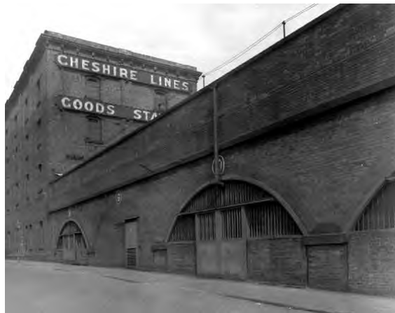
Figure 15 – 1938 – A view looking north-east along Watson Street showing the former Cheshire Lines Goods Station warehouse, adjoining Manchester Central Station.
