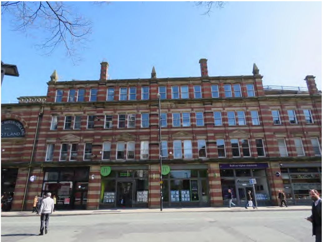
Figure 60 – The northern four storey block.
