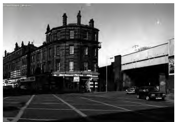
Figure 42b – 1990 – The southern corner of the Deansgate terrace, showing the original viaduct which carried rail traffic over Great Bridgewater Street into the rear of the warehouse.
