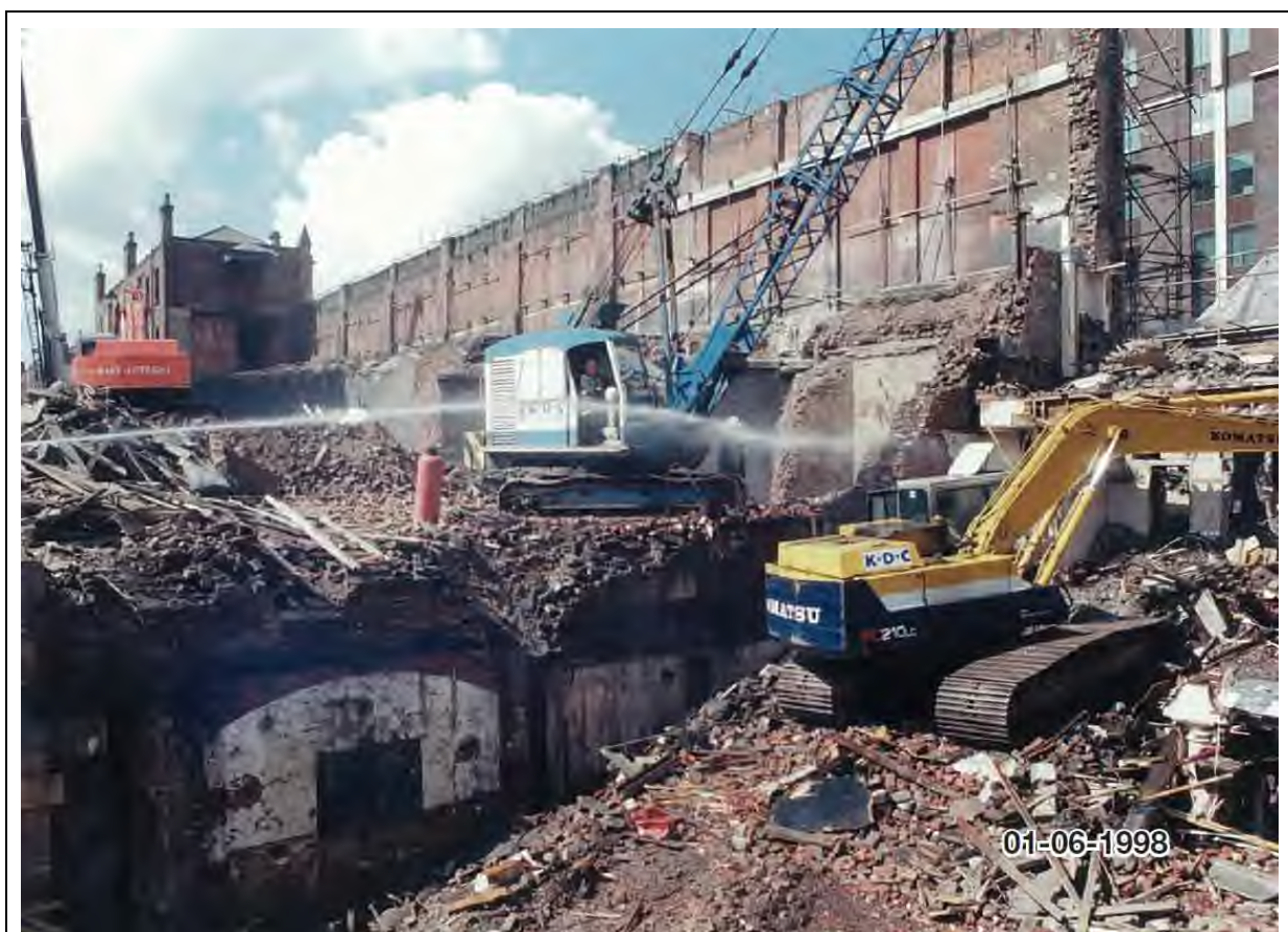
Figure 23: Looking south with views of Deansgate Terrace and Former Goods Station entrance c.1998. The carriage ramp is pictured as largely dismantled. Note the rear side of the goods entrance (now grade II) to the right of the image, elevation retained.
