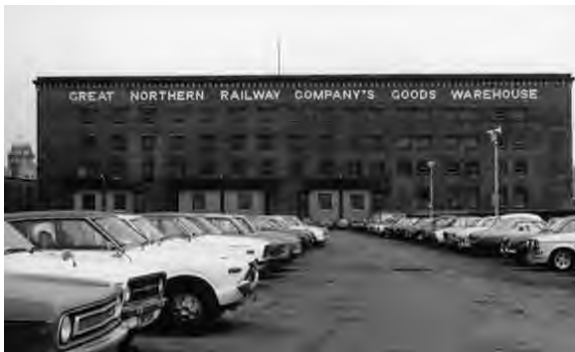
Figure 17 – 1986 – Looking north towards the rear of the warehouse during its use as a flat surface car park.
