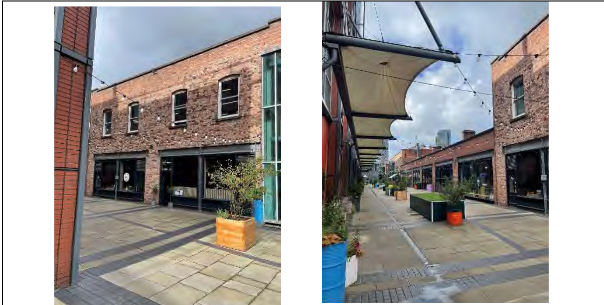
Figure 62 and 63 – The altered rear (east) elevations of the Deansgate shops range.
