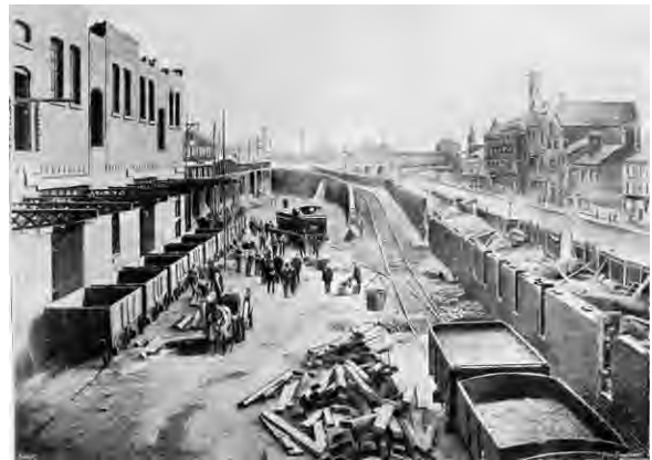
Figure 29 – An illustration of the construction of the Great Northern Warehouse in 1897, looking south. The warehouse can be seen partially constructed to the left, with the ground floor level of the range of Deansgate shops to the right.
