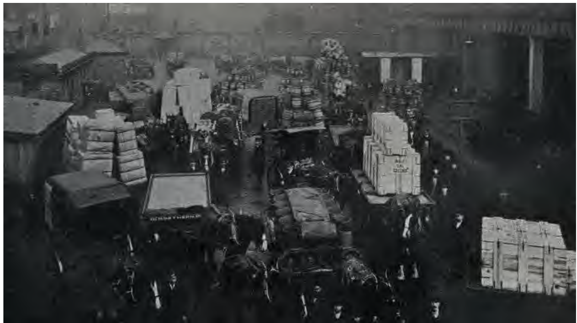
Figure 37 – The goods yard in the early 1900s, showing the entrances into the ground floor of the warehouse to the right, the rears of the buildings fronting Peter Street to the left, and the former walls and gated entrance into Watson Street in the background. This image shows the extremely busy and hectic nature of the site's early years.
