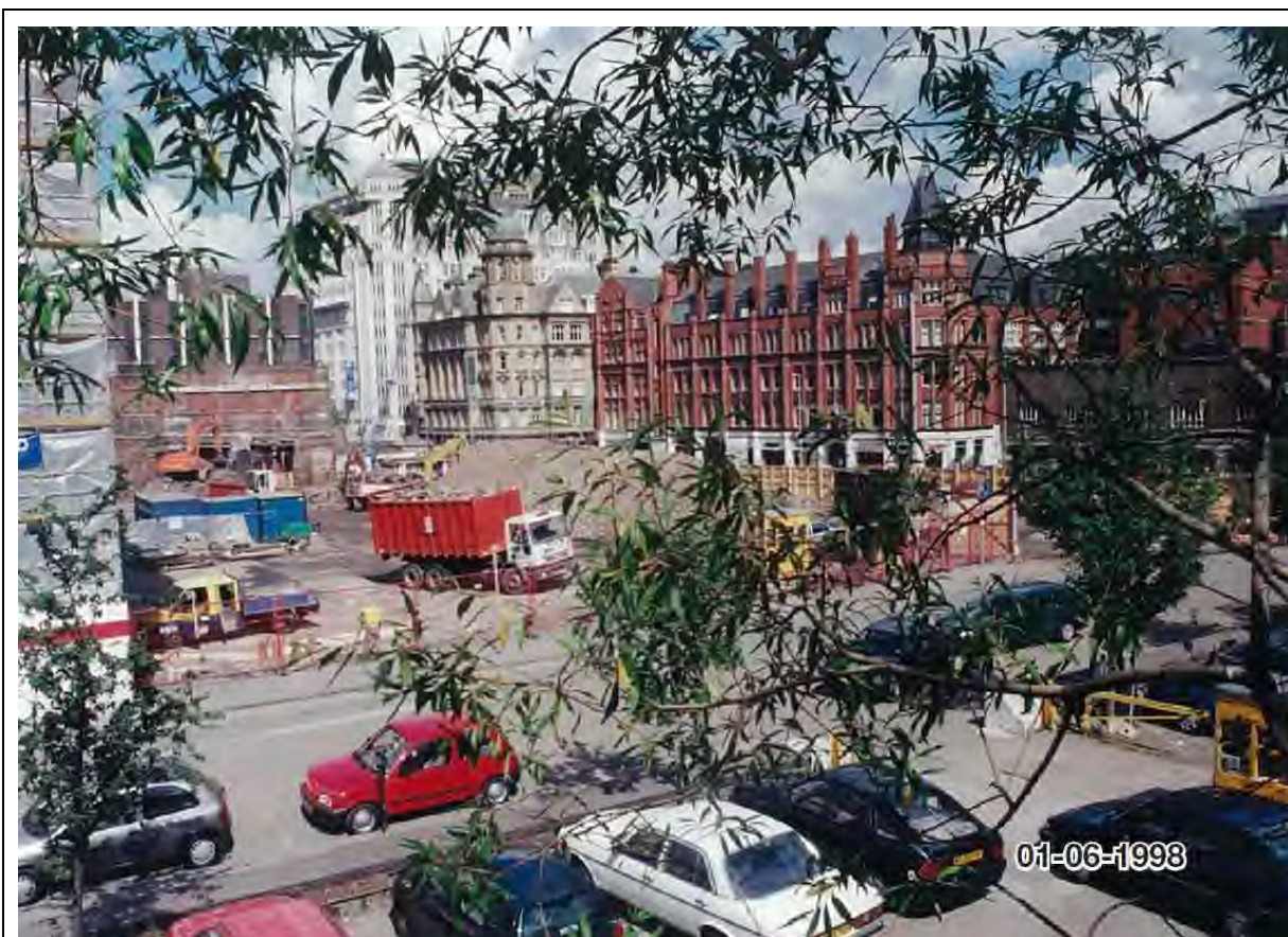
Figure 21: Looking west towards the northern aspect of the site in June 1998, demolition of carriage ramp and Peter Street buildings shown to be underway.
