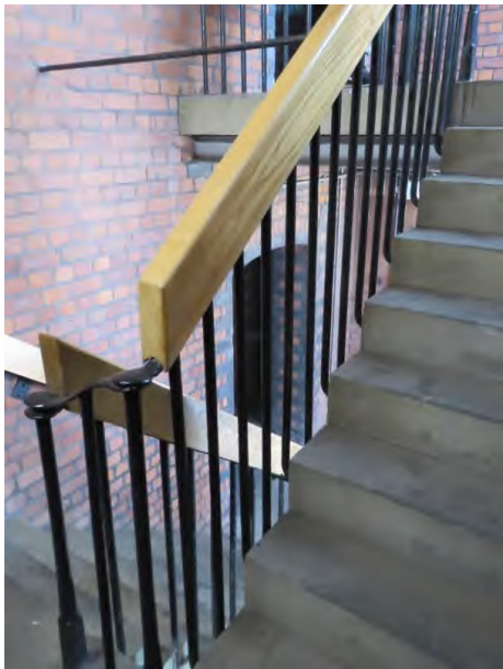
Figures 54: Example of one of the four remaining original cast iron/stone staircases, showing modern timber handrails.
