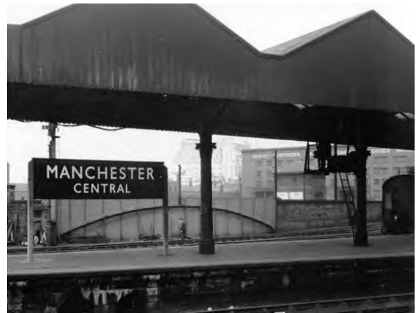
Figure 16 – c1958 – A view looking north-west from the former Manchester Central Railway Station, to the disused rear of the Great Northern Warehouse and sidings.
