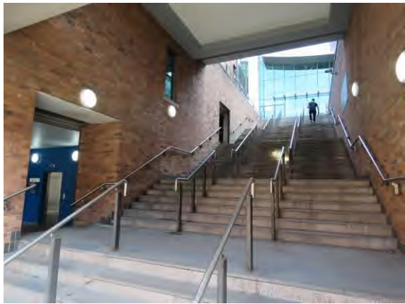
Figure 68 – The early c.2000s inserted stair and raised deck from Deansgate to the upper level.
