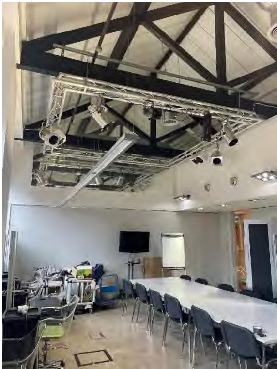
Figure 65 – A typical shop unit. Modern alterations and subdivisions. Modern roof and truss arrangement.
