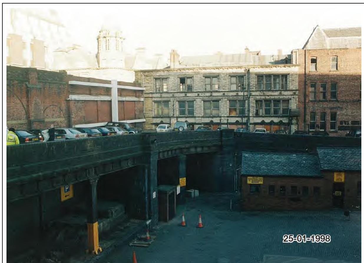
Figure 19: Looking north towards Peter Street (rear side) c.1998. The sloped carriage ramp is well represented from this location, pictured here before it was dismantled. Note the rear side of the goods entrance (now grade II) to the left of the image.
