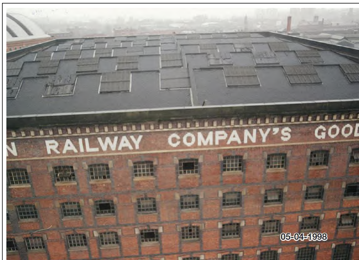
Figure 24: Looking south with views of the original roof to the Goods Warehouse, prior to alterations made in early 2000s.
