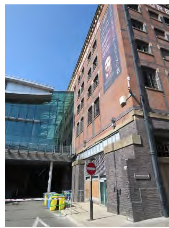
Figure 51 – The south elevation showing the c2000 leisure box link building supported upon the original steel track bed.
