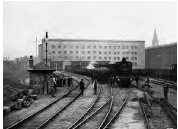
Figure 31 – A view looking north towards the southern end of the newly completed warehouse in 1898, showing the high level station and tracks which enter the warehouse at this first floor level.
