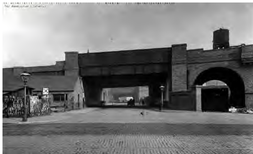
Figure 14 – The completed viaduct as seen on the 31 st August 1900. Note the empty plot housing construction workers huts on the left, of which the Deansgate Terrace of shops is to be soon built upon.
