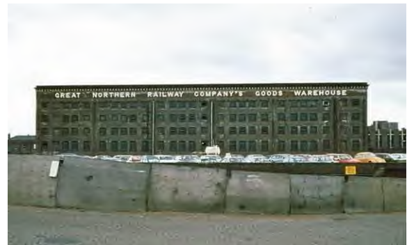
Figure 18 – 1988 – A view looking west towards the eastern elevation of the warehouse, as seen from the cleared Cheshire Lines Goods Station site.
