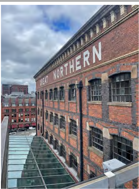
Figure 49: Modern extension to west elevation, pictured from elevated location on modern car park ramp. Looking north
