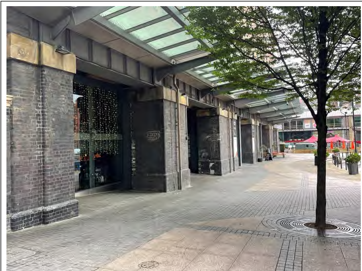
Figure 47 – The north elevation of the warehouse, showing the ground floor entrances and c2000 glass canopy.
