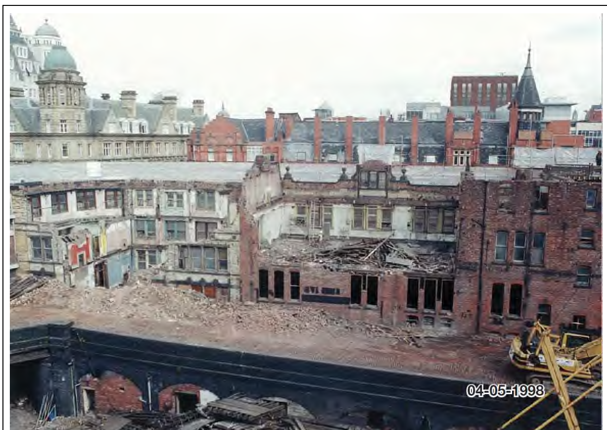
Figure 22: Looking north towards Peter Street (rear side) May c.1998. The sloped carriage ramp is pictured here before it was dismantled. Peter Street buildings pictured being demolished.
