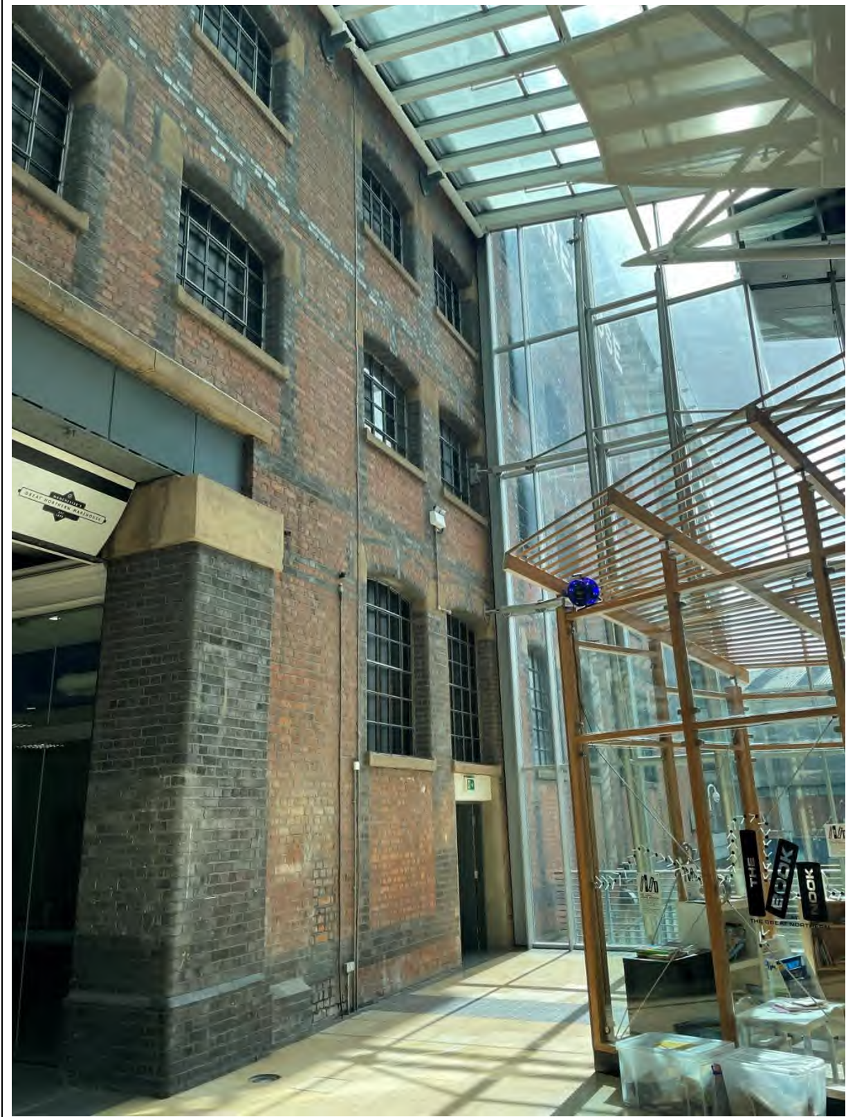
Figure 52: Looking north from inside the first floor link building towards the former train openings.
