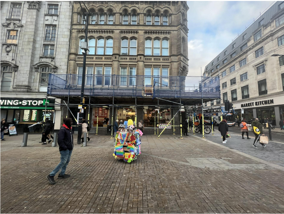
02 PHOTO OF SCAFFOLDING ON PICCADILLY SCALE NTS@A3
