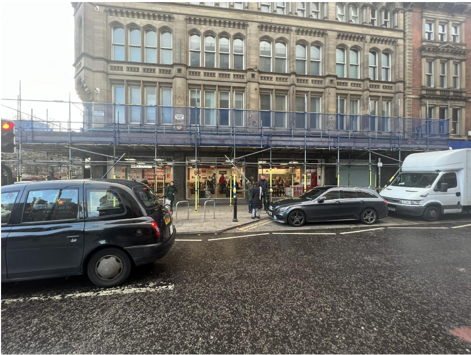
03 PHOTO OF SCAFFOLDING ON OLDHAM STREET SCALE NTS@A3
