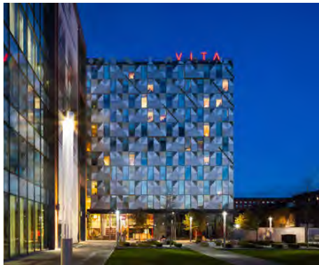
12. Vita, First Street (up to 12 Storeys), 5plus Architects
