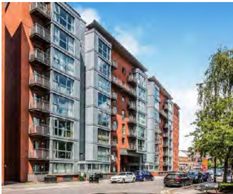
9. The Nile Building, (up to 8 storeys)
