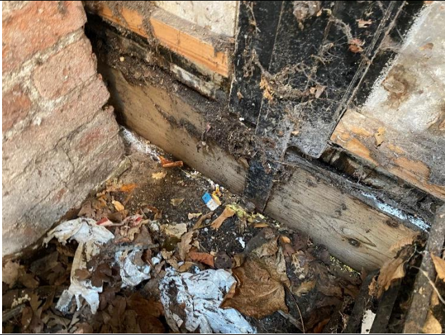
Existing sliding door wheel bracket
