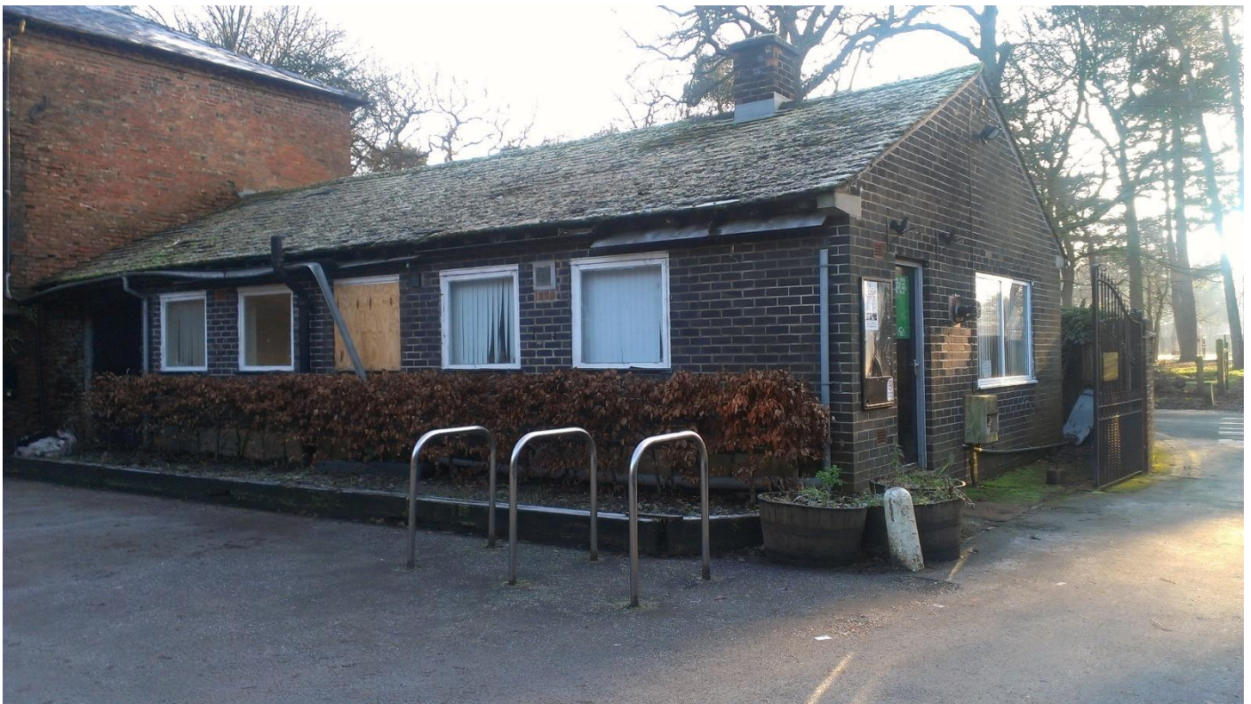
Figure 19 Former 1950s office and bungalow demolished in 2015.
