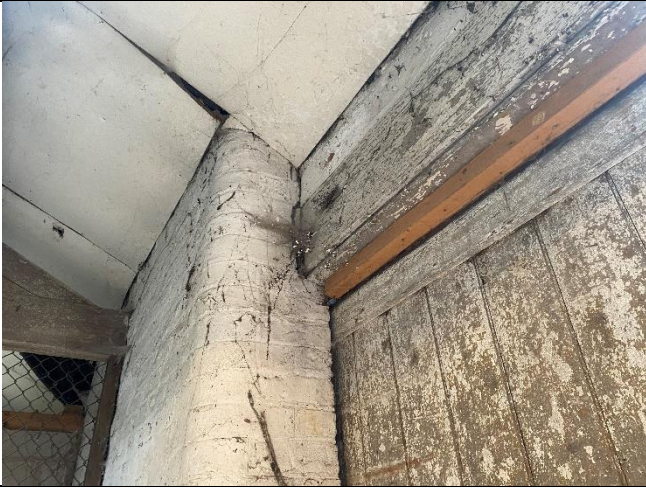
Existing doors to rear
