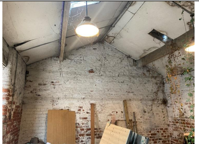
Inside the new facility looking south.
