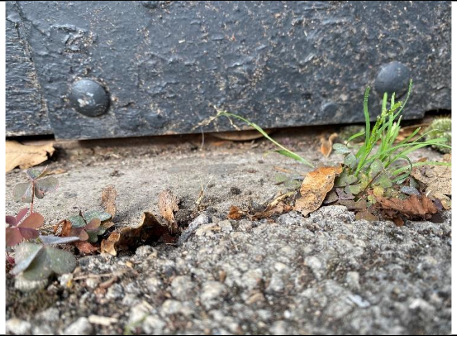
Existing sliding door wheel
