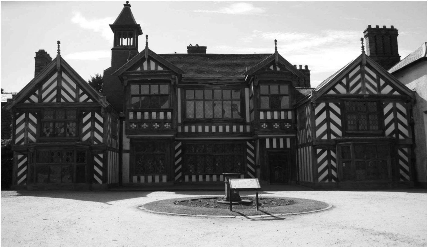
Figure 5 Hall Forecourt, before the fire, 2010.
