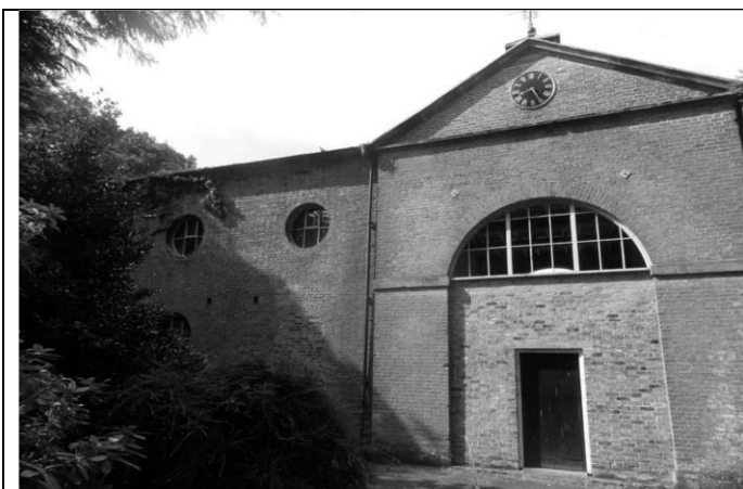
Figure 17 Former Stable Block, 2016.
