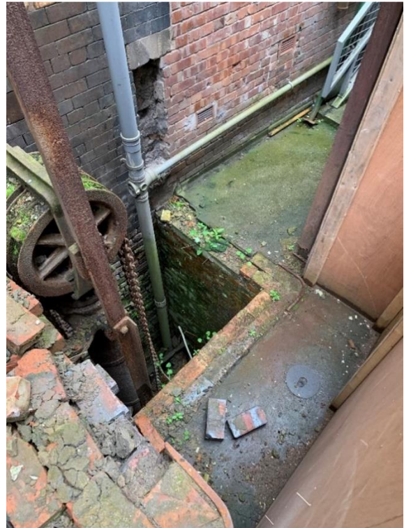
Photo 2: Courtyard – Location of Plant compound
