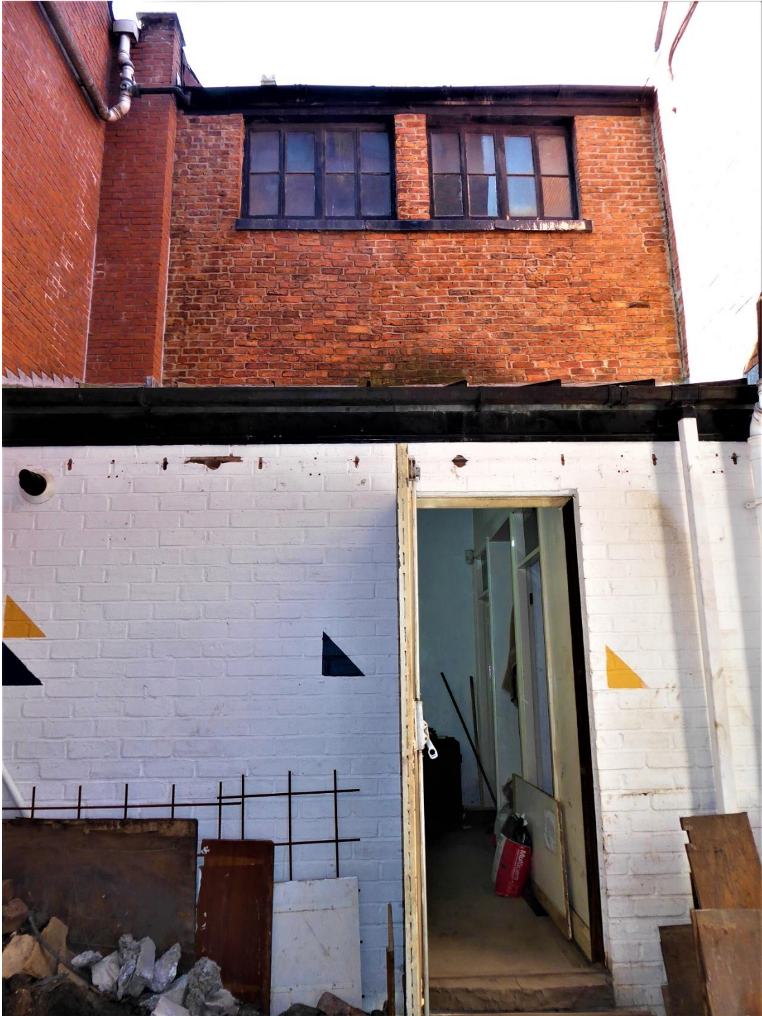
Photograph 2 – Rear elevation of property.
