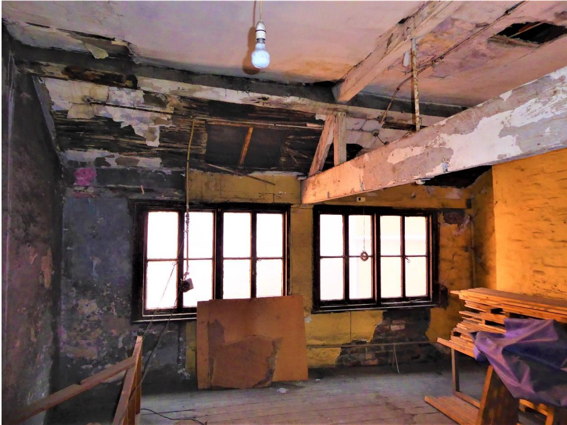
Photograph 6 – Internal view of rear elevation at second floor level.
