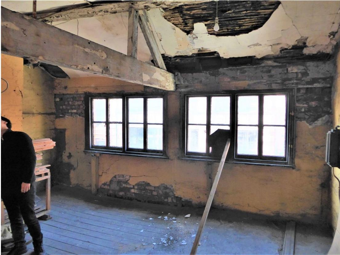
Photograph 7 – Internal view of front elevation at second floor level.
