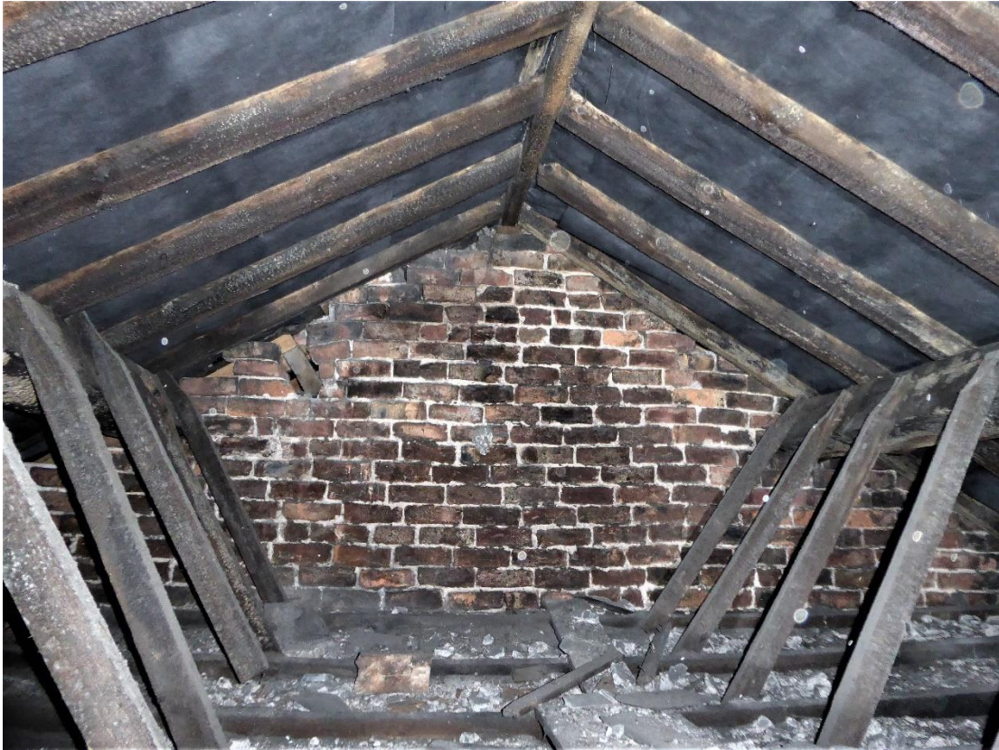
Photograph 3 – General view of internal roof structure.
