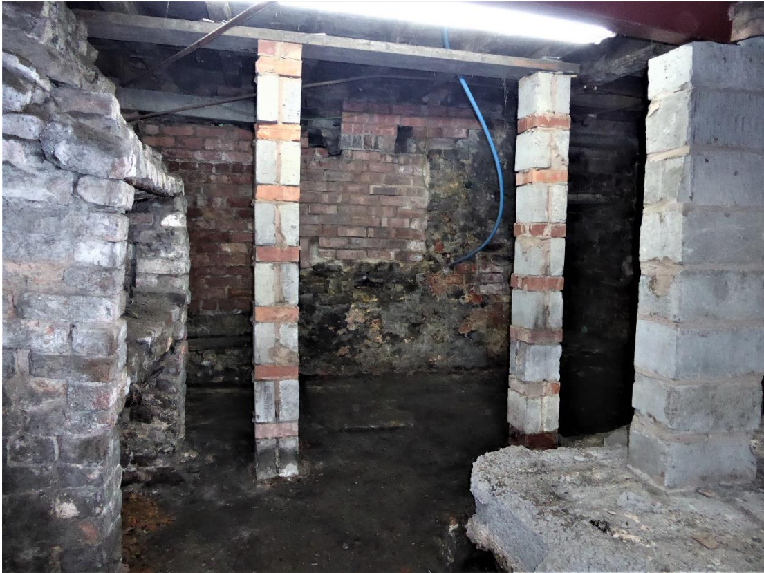
Photograph 18 – Showing modern masonry piers in basement.
