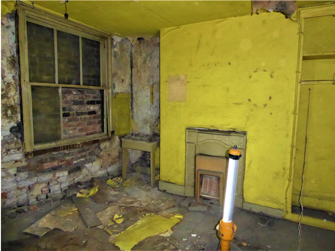
Photograph 13 – Showing internal view of rear room at first floor level.
