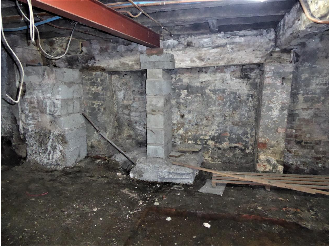
Photograph 20 – Showing more remedial strengthening to ground floor.
