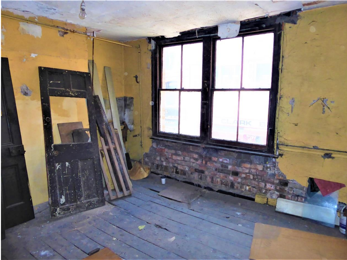
Photograph 10 – Inside view of front elevation at first floor level.
