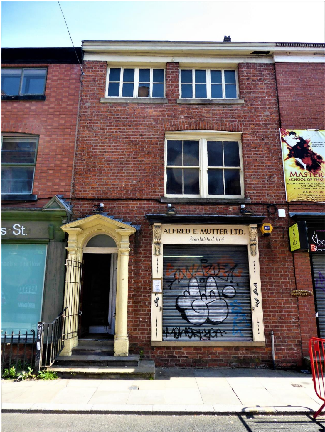
Photograph 1 – Front elevation of property.
