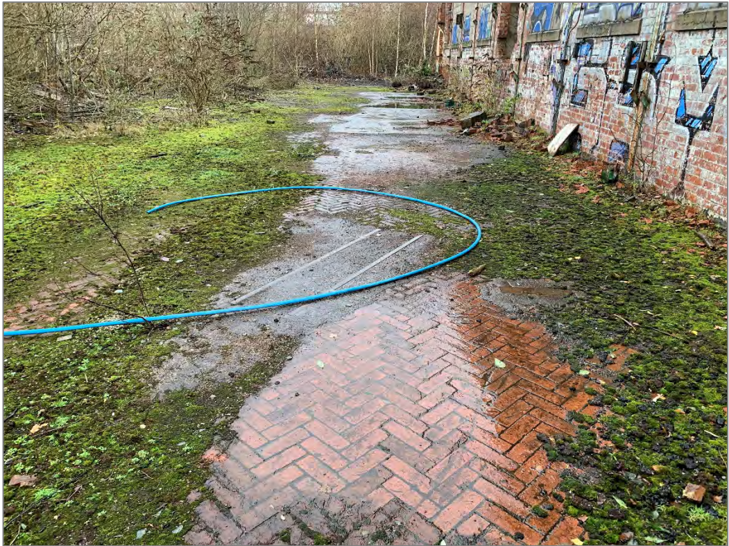
Photograph 15: View of brick flooring in the east of the site looking north
