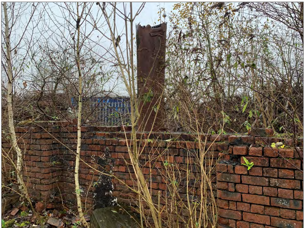
Photograph 12: View of structure remains in the north of the site looking northeast
