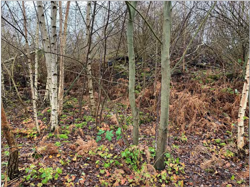
Photograph 11: View of possible demolished structure looking south from towpath
