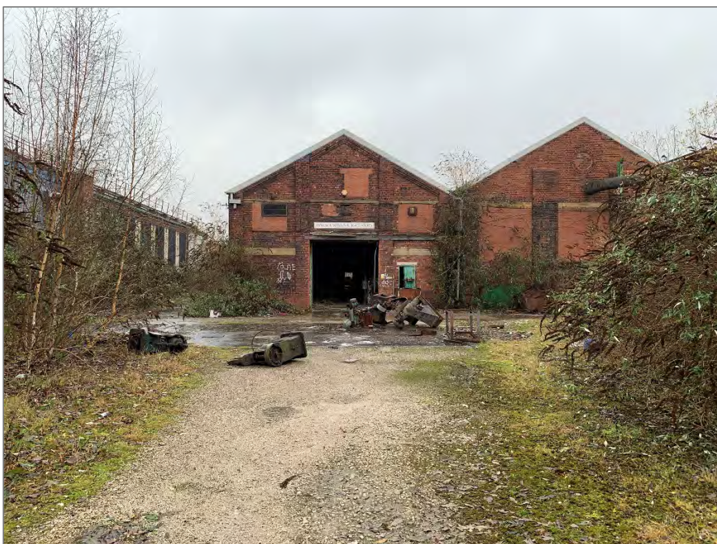
Photograph 5: View of warehouses from centre of site looking north
