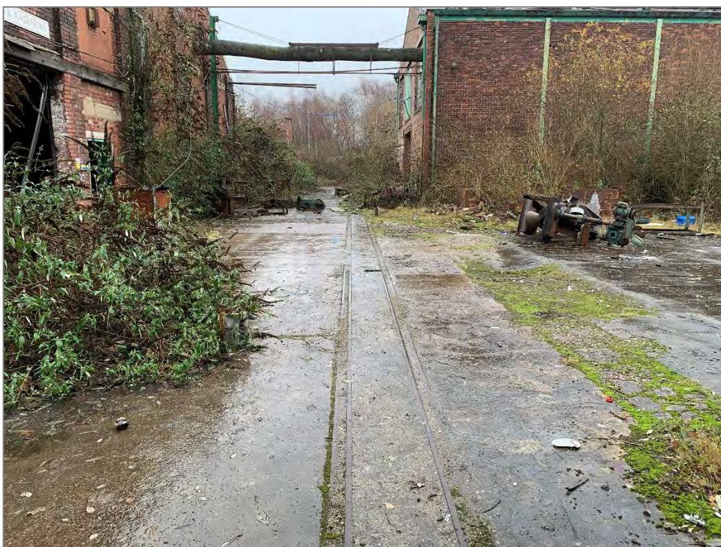
Photograph 9: View of tramway looking east
