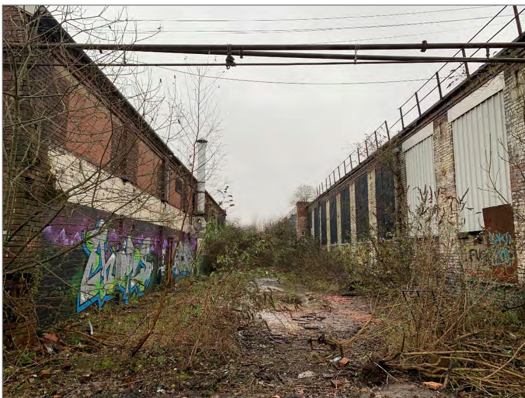
Photograph 7: View of warehouses from the north of the site looking south
