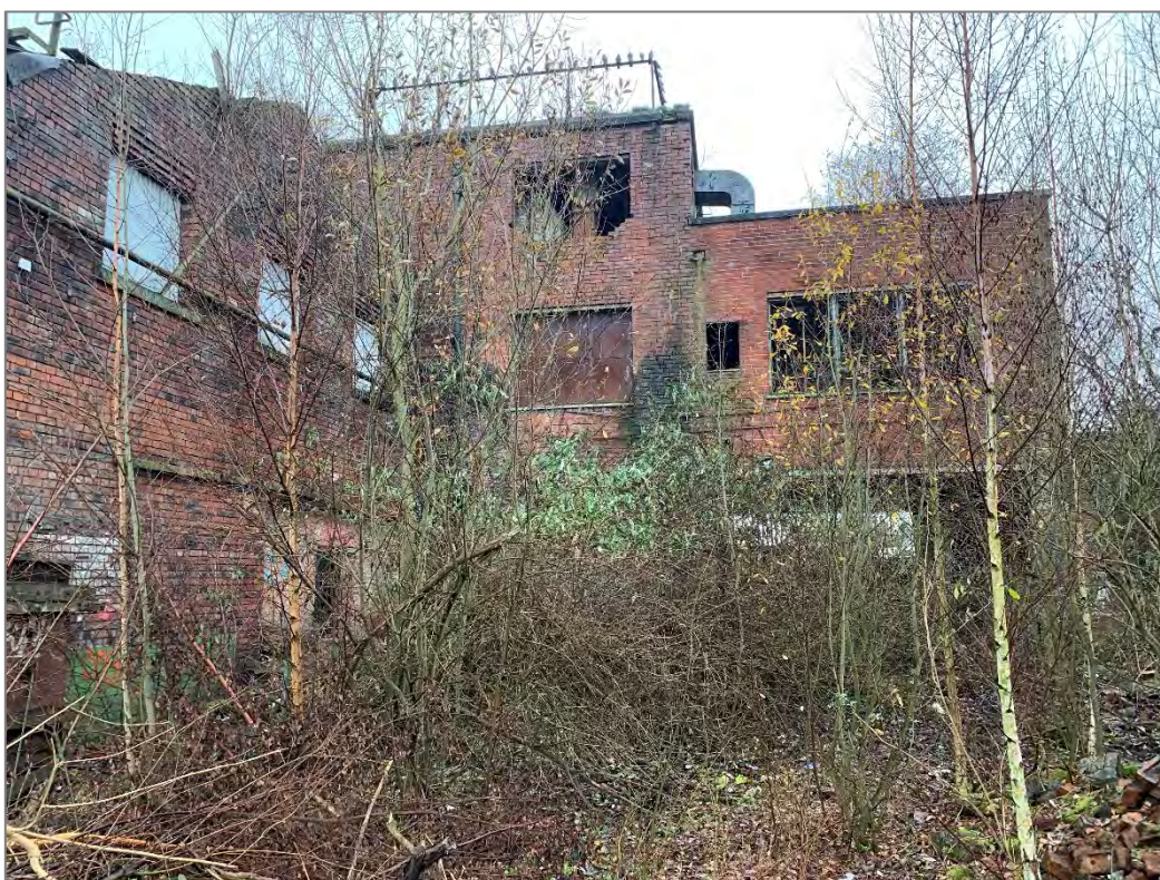
Photograph 6: View of warehouse from the north of the site looking west
