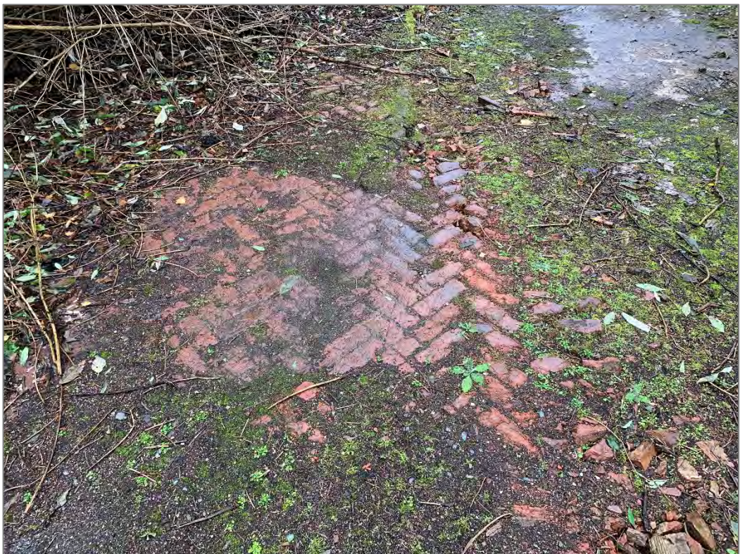
Photograph 14: View of brick flooring looking north
