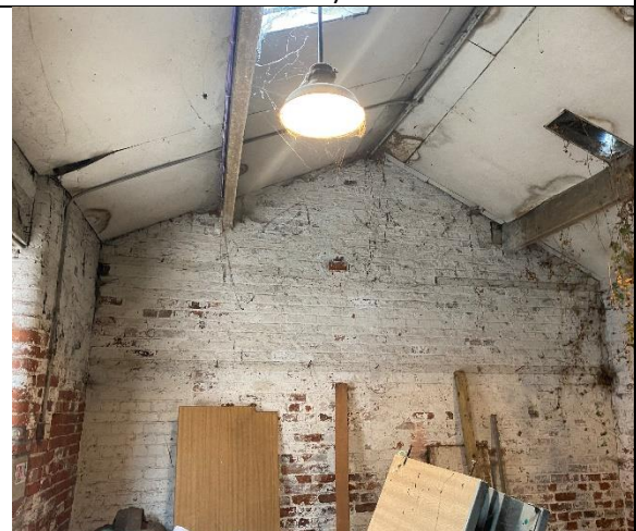
Inside the new facility looking south.
