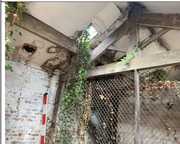
Inside the new facility looking North.
