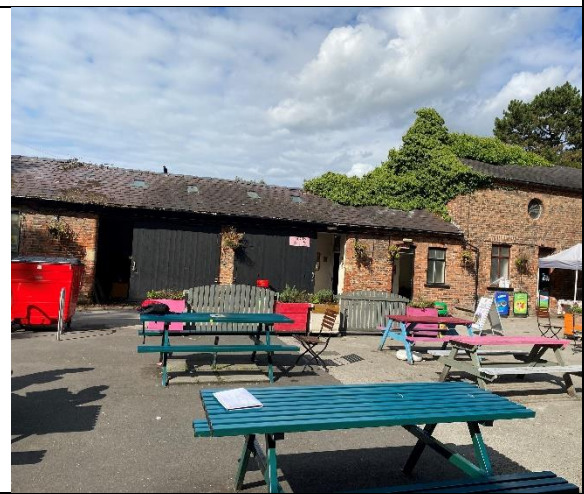
Location of new facility (behind door on the left)
