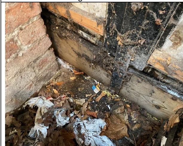
Existing sliding door wheel bracket
