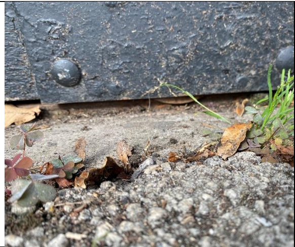
Existing sliding door wheel
