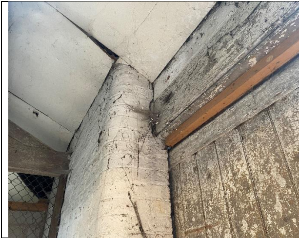
Existing doors to rear
