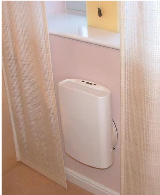
Figure 6 In-situ Titon Sonair acoustic vent
