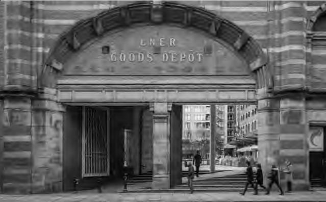
Entrance arch at the North end of the facade. Characterised by deep reveals. Signage in the semi-circular tympanum
