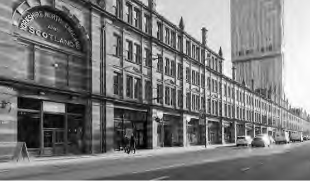
Pilasters mark the rhythm of the facade along its full length. In the first section of the facade a smaller arch reveal with a tympanum graphic.
