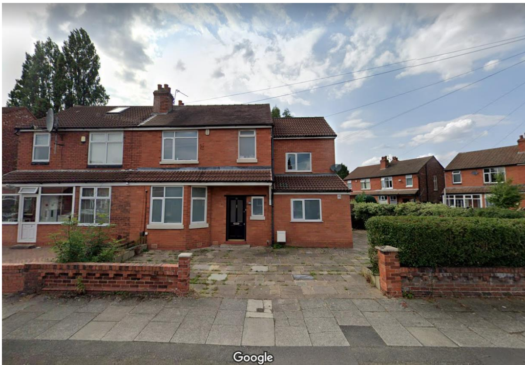
Photograph 1 Application site as viewed from Brocklebank Road. Source : www.google.com/maps accessed 23.11.2022
