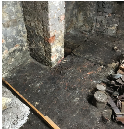
04 ORIGINAL BRICK FLOORING IS VISIBLE THROUGH THE DIRT FLOOR. UPON INSPECTION, THE BRICKWORK IS SATURATED WITH WATER AND BREAKS APART EASILY SO IS UNFORTUNATELY UNSUITABLE FOR RE-USE. NEW FLOORING WILL BE CHOSEN TO REPLICATE THE ORIGINAL INTENT / LAYING PATTERN.
