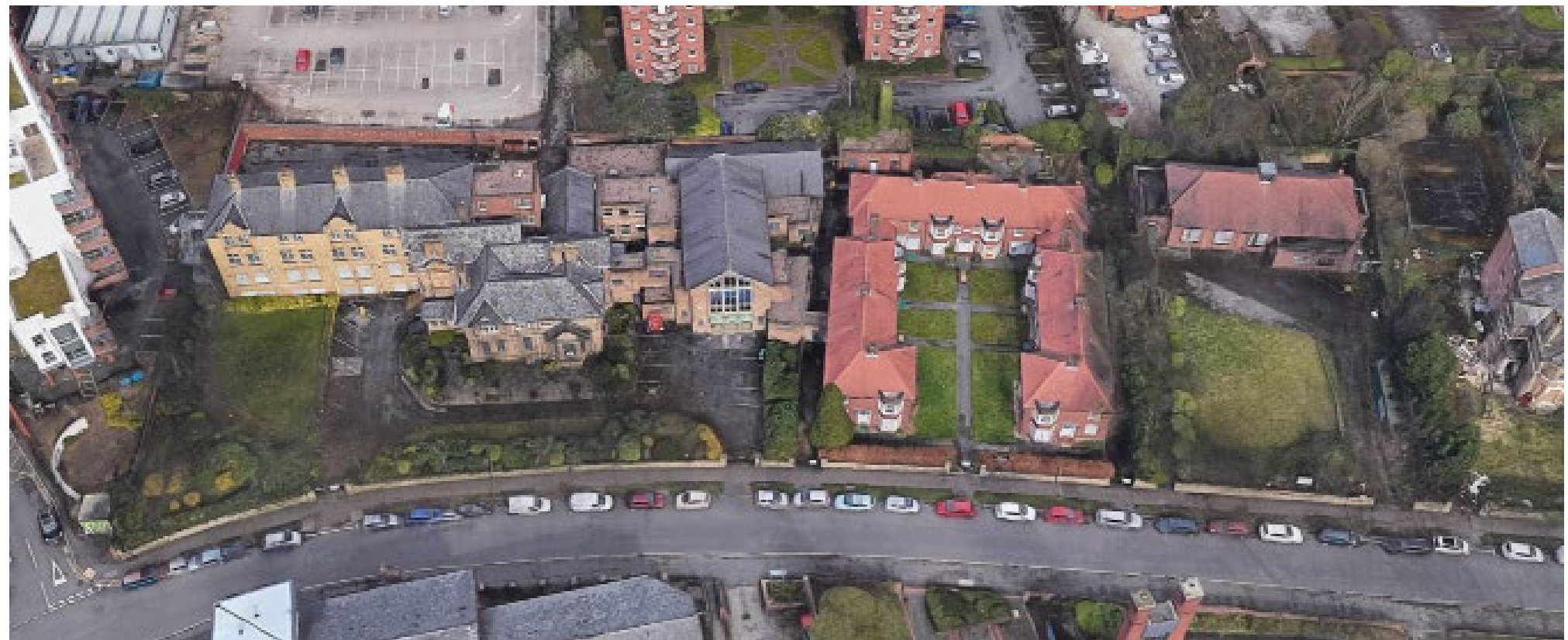
Current site Aerial
