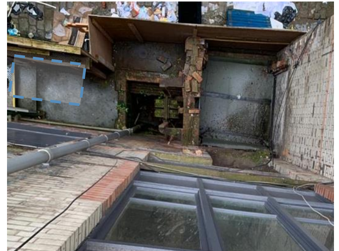
High level view of proposed generator location
