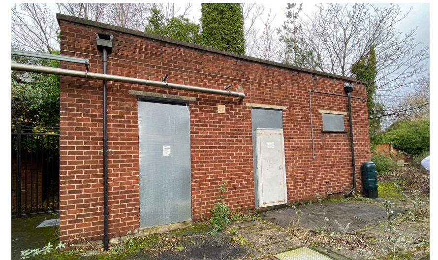
Photo of existing boiler room
