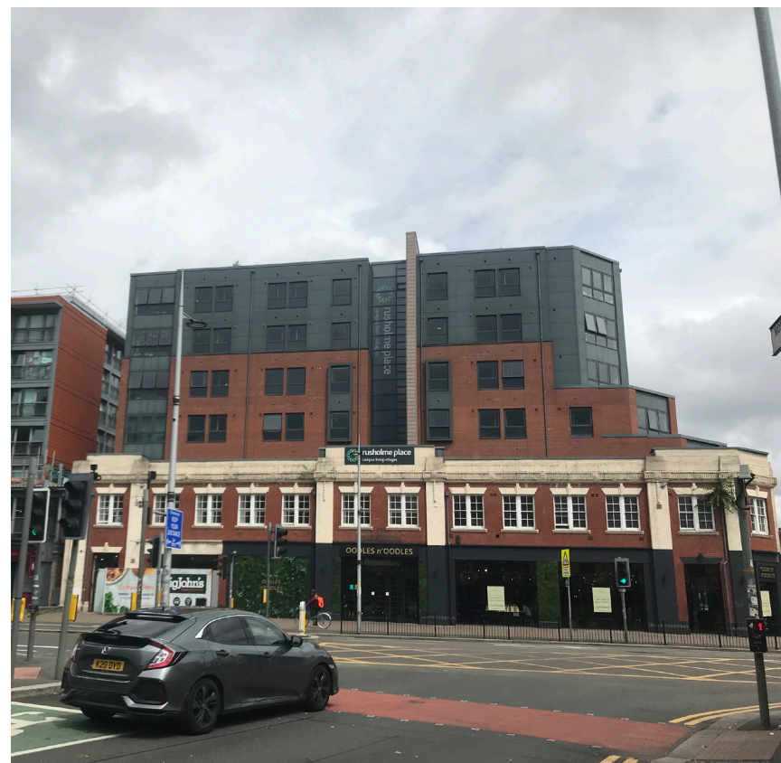
B - View of Rusholme Place, student accommodation, from Oxford Road
