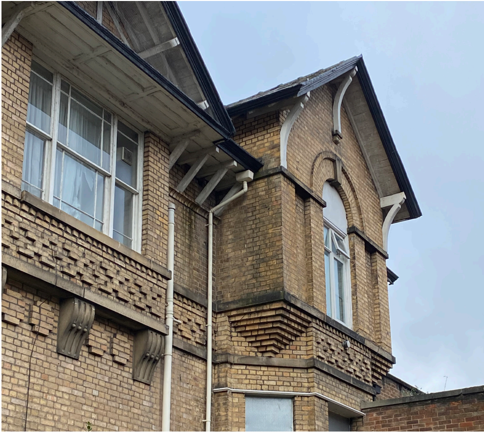
PHOTOS OF EXISTING BRICKWORK TO ST GABRIEL'S
