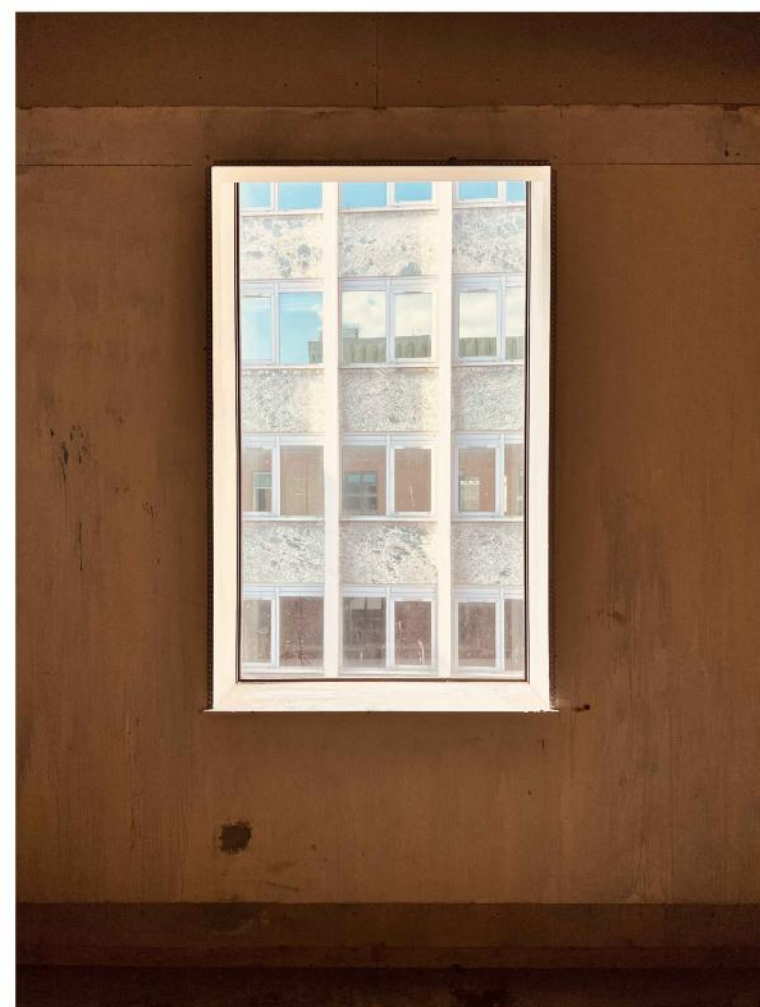
03 THIRD FLOOR EXISTING WINDOW PHOTO SCALE - N/A PHOTOGRAPH
