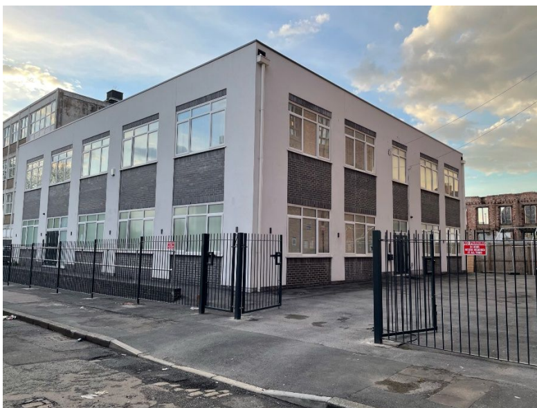
Plate 4-3: Photograph of completed development.
