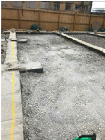
CLEAN MOT BEING INSTALLED
