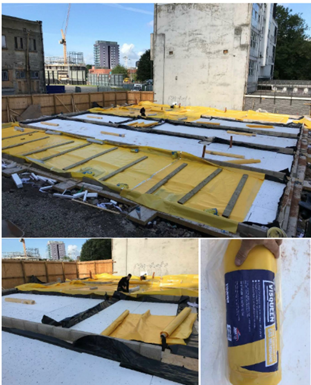
Plate 4-2: Membrane installation photographs.
