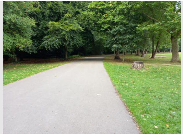
Photo 26: Path surrounding the site
