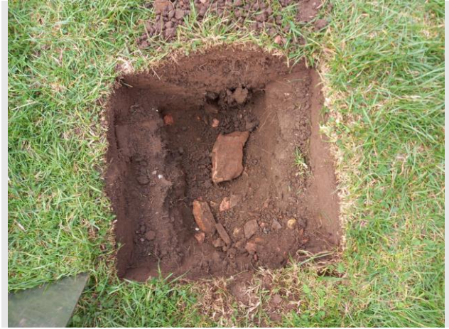
Photo 20: Drain line excavation
