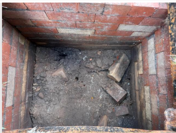
Photo 9: Outlet manhole chamber in the south-western corner
