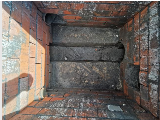
Photo 7: Manhole chamber in the north centre of the site
