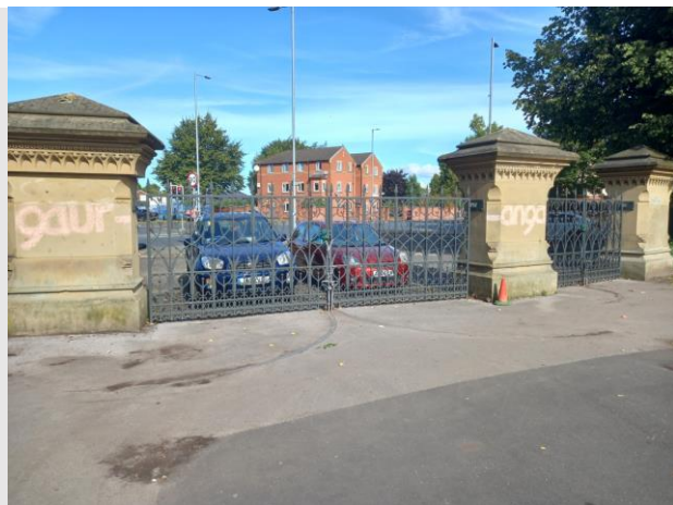
Photo 27: Existing access – maintenance access
