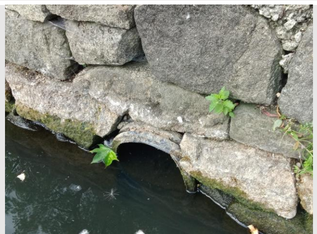
Photo 10: Existing outlet into pond, 200 mm plastic unperforated pipe
