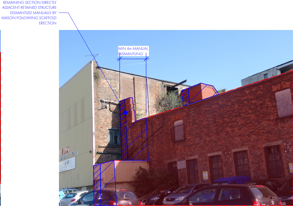
IMAGE 002- PIGEON STREET - Junction between retained and demolished
