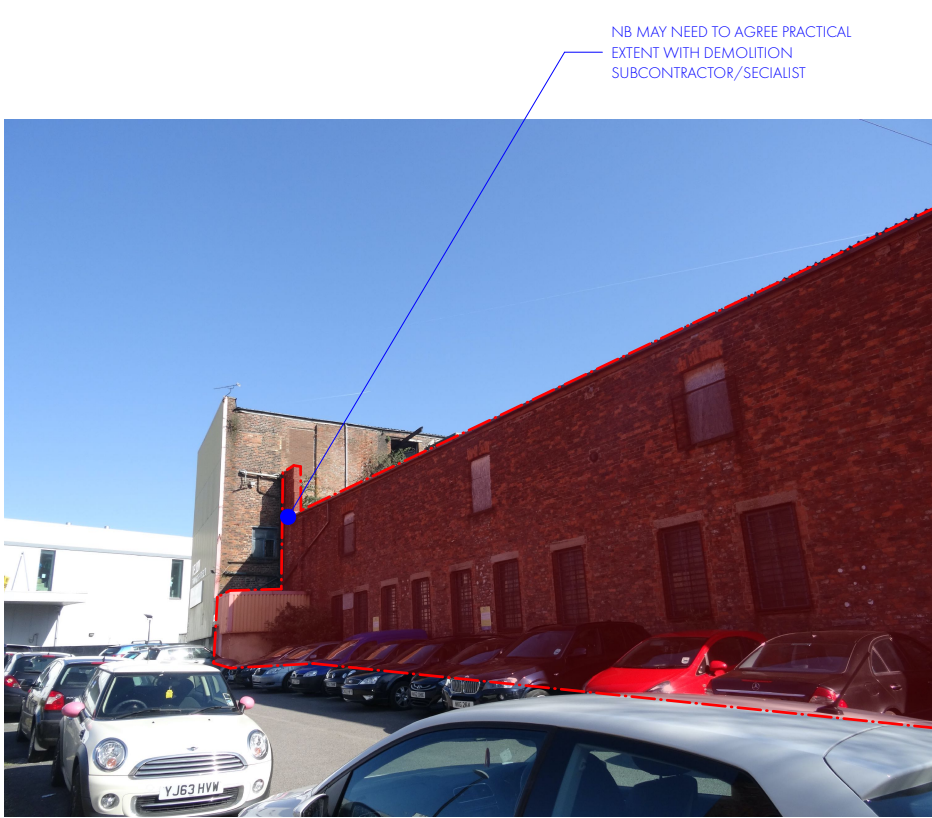
IMAGE 001 - PIGEON STREET - Junction between retained and demolished
