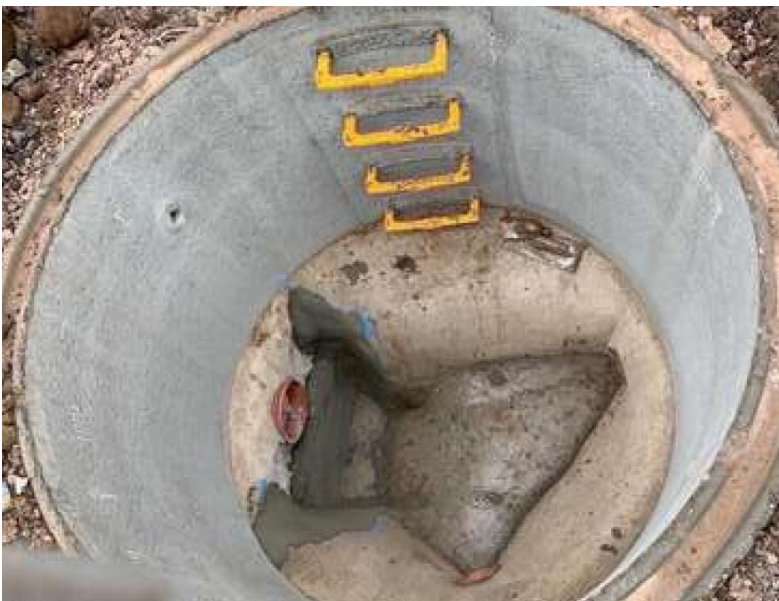
Photo 2 – Chambers SW7 and SW9 either site of the attenuation tanks are in place and being benched up
