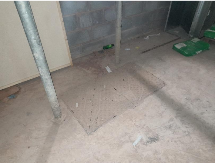
Photo 5 – SW07 Catchpit Cover
