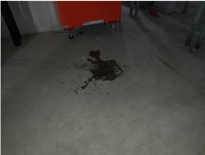
Photo 12 – Surface Water Gully
