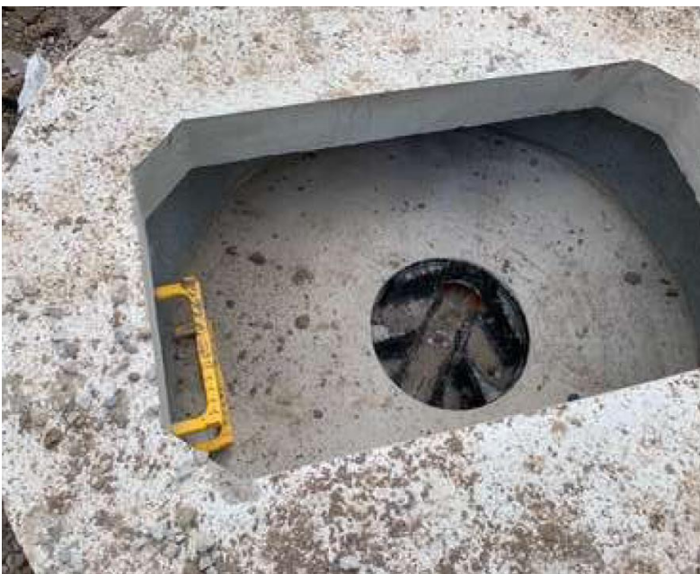
Photo 1 – As built Chamber SW02 Access Point
