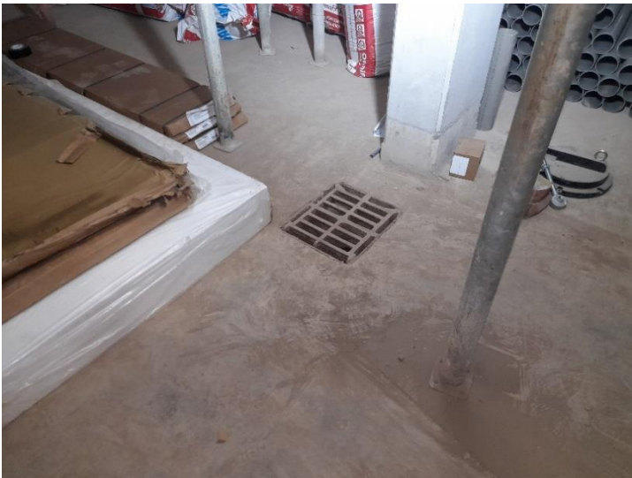
Photo 9 – Surface Water Gully
