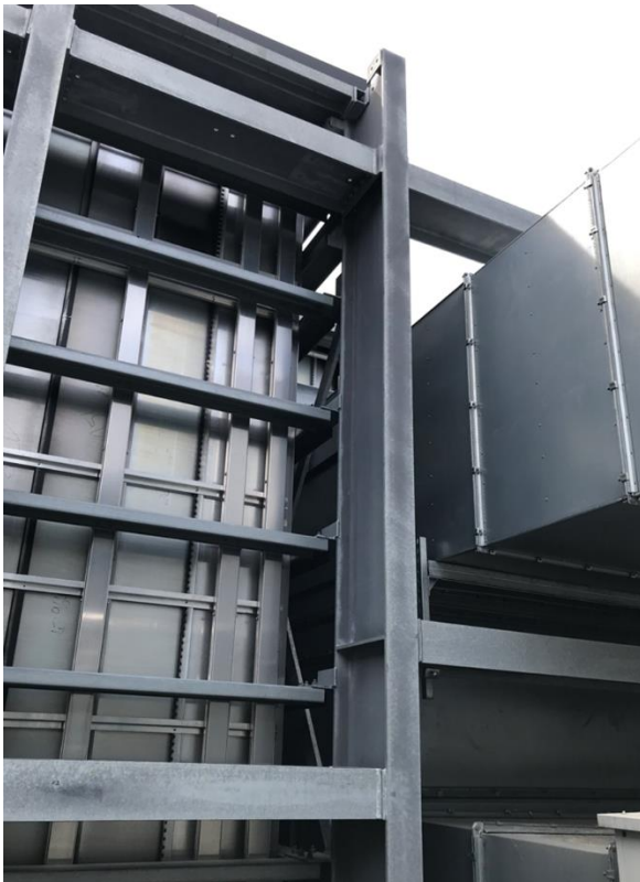
Figure 3 Photograph of installed plant screen
