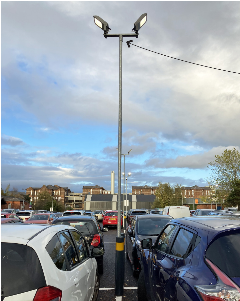
TWIN LIGHTING EUROFLOOD MIDI LED MOUNTED ON 6M POST
