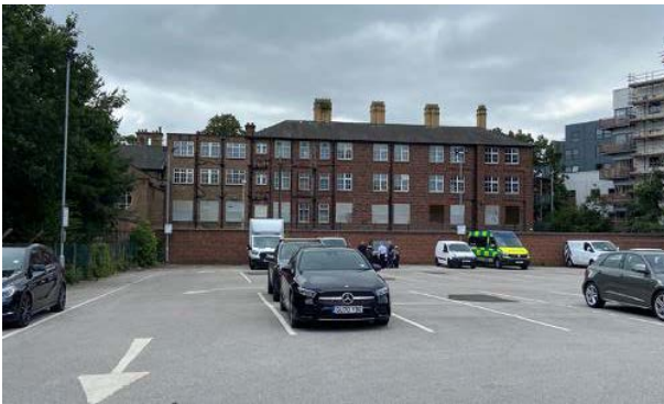
Figure 31: North elevation of the 1922 extension and 1950s extension/ infill to the left.
