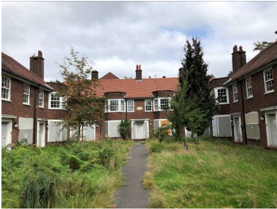
Figure 44: South, west (left) and east (right) elevations of Woodthorpe Hall
