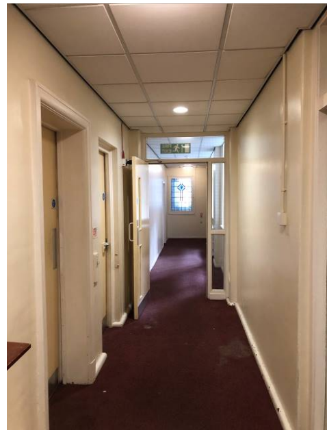
Figure 39: Internal corridor within the 1922/ 1950s extension to the villa.
