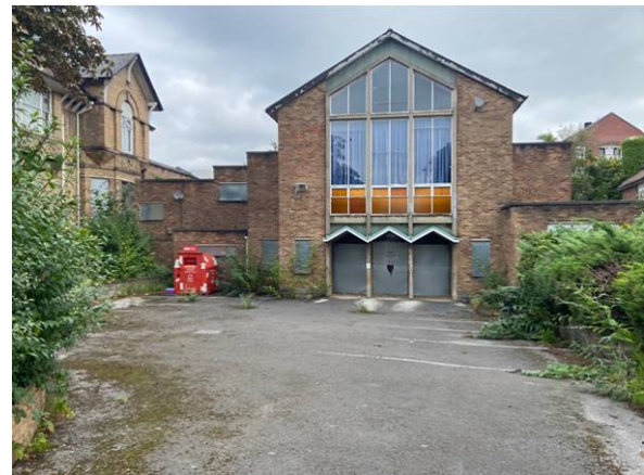
Figure 30: South elevation of the 1963 chapel
