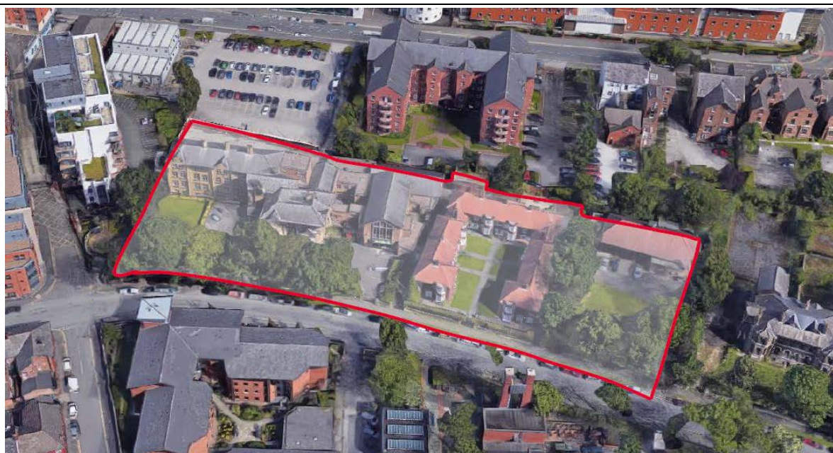
Figure 1: An aerial view looking north-east across the Site (outlined). Source: Google, c.2020.
