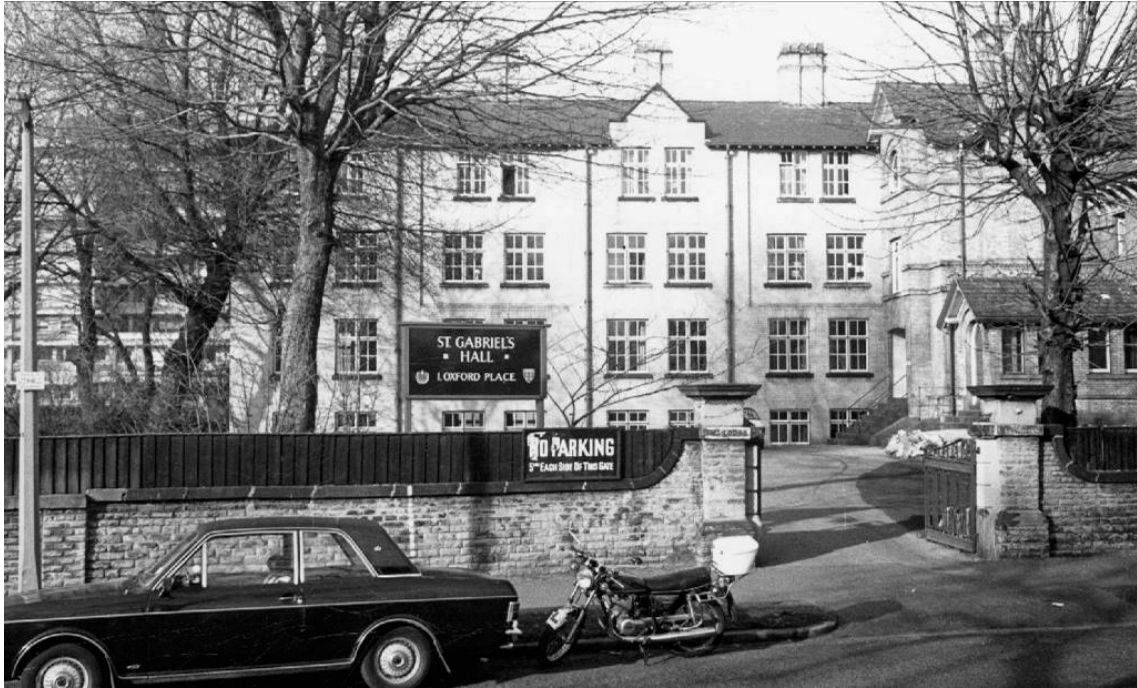
Figure 15: The 1922 extension in 1976. (Source: Manchester Archives)
