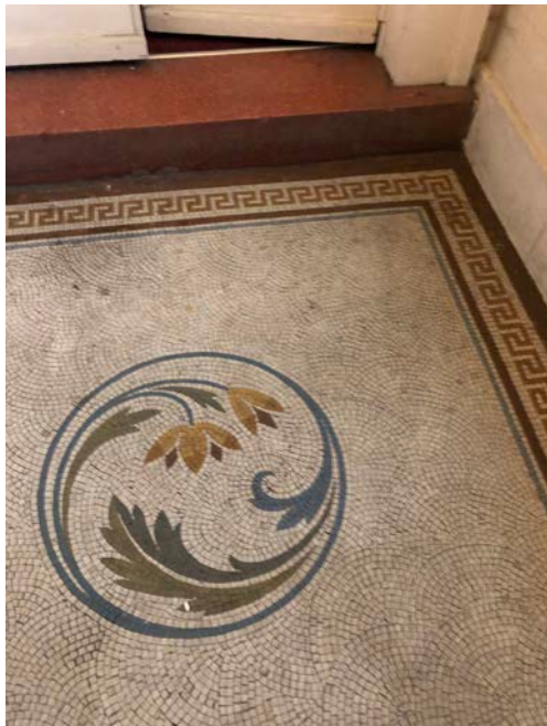
Figure 34: Detail of the 19 th century mosaic lobby floor.
