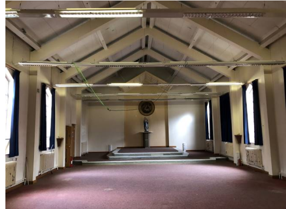
Figure 41: Looking north across the first floor 1963 chapel.
