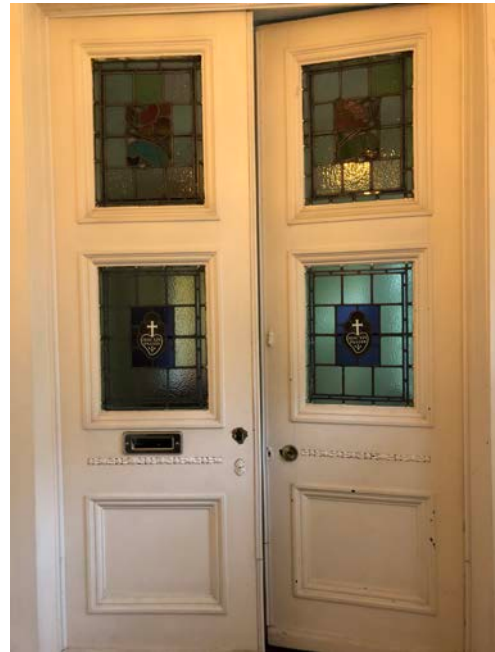
Figure 33: Inner entrance doors to the lobby, with original c1850s double stained glass doors.
