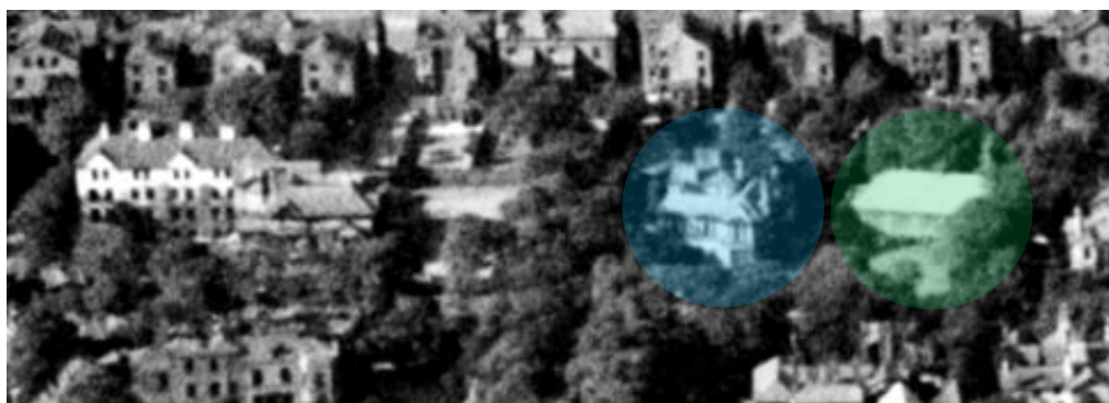
Figure 17a: Looking north over the Site in 1937, showing the original Woodthorpe villa shortly before its demolition (shaded blue), and the completed St David's Church Hall shaded green to its right. (Source: Britain From Above)
