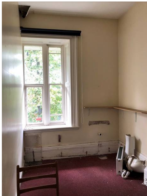
Figure 38: Example of the alterations that have taken place to the first floor of the c.1850s villa; rooms have been subdivided and original features removed
