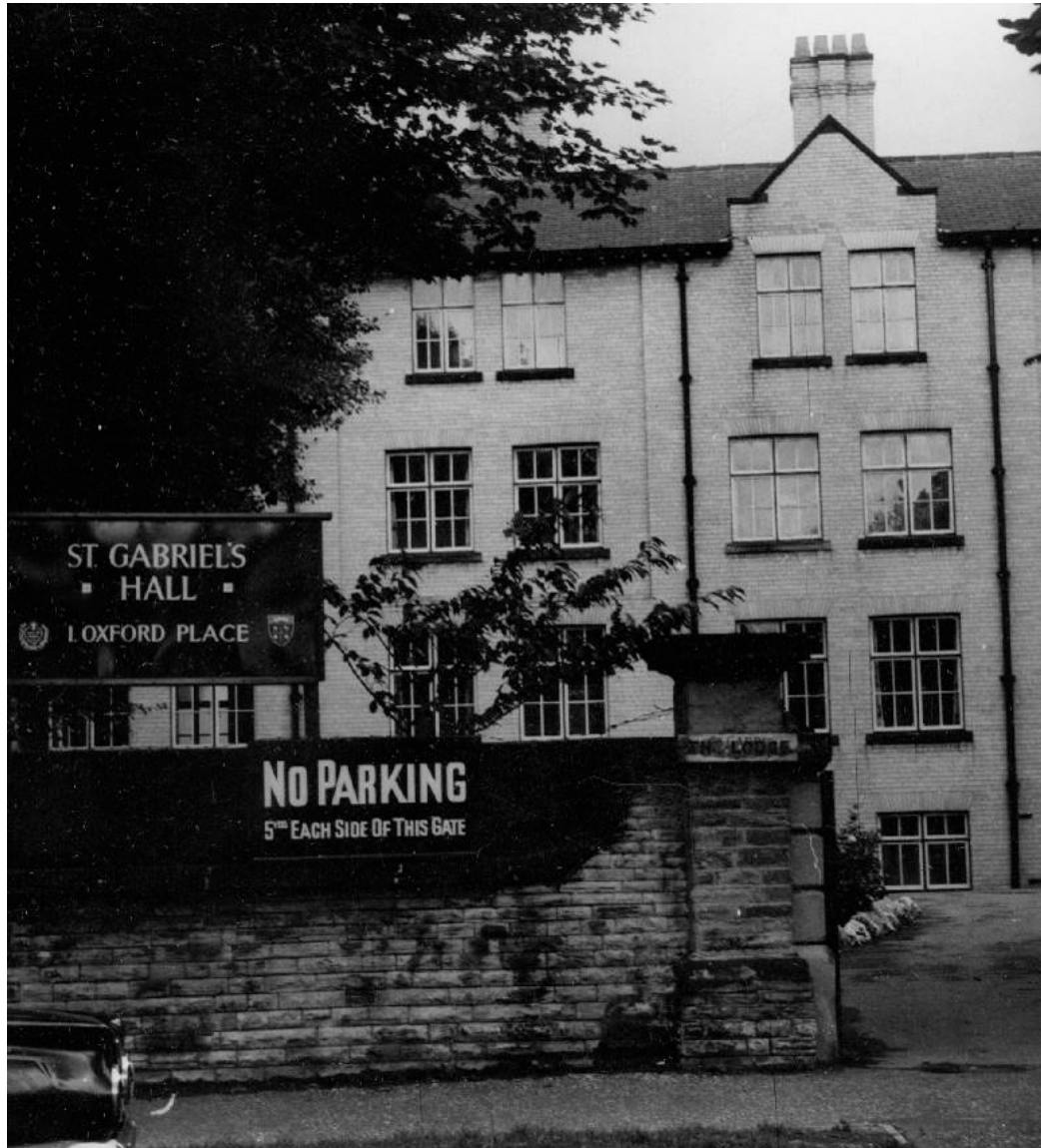
Figure 14: The 1922 extension seen in 1970. Note the original windows which are now replaced with UPVC. (Source: Manchester Archives)
