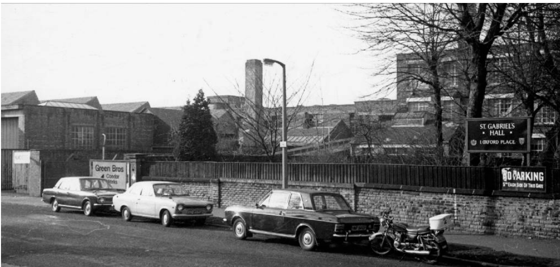
Figure 16: The western end of the Site as seen from Oxford Place in 1976. The lamp post denotes the location of the original gate lodge, which was demolished in the 1930s. (Source: Manchester Archives)
