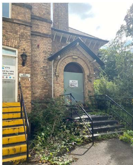
Figure 27: West elevation of the original entrance of the c.1850s villa to the right; additional entrance to the left created by altering a historic window opening.
