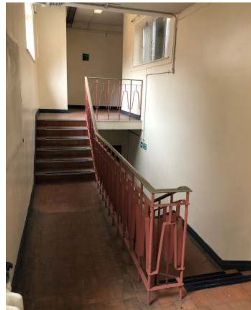
Figure 43: Interior of the 1963 extension that links the chapel with the villa.
