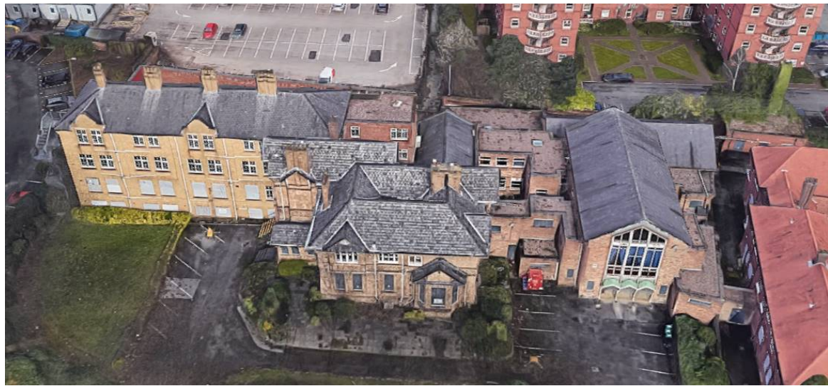
Figure 6: Aerial view of the western part of the site. From left to right – the 1922 extension, the c.1850s villa, and the 1963 Chapel
