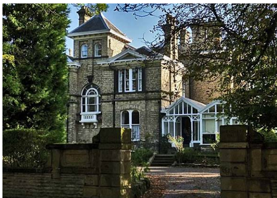
Figure 10: Greygarth Hall, originally called Lilly Villa, built in c1868 immediately south-east of the Site.
