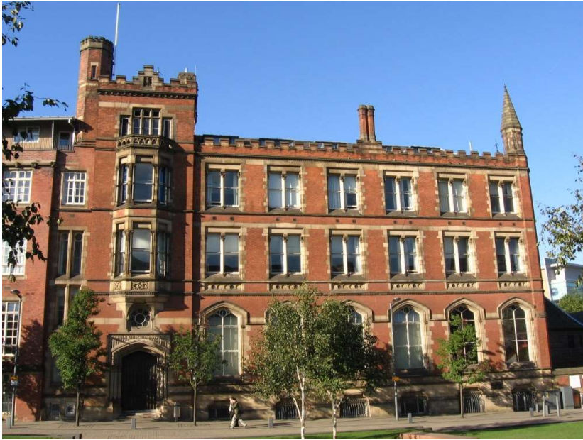
The Millgate Building, Long Millgate: The double height windows in Whiteley Hall are visible before the fire.
