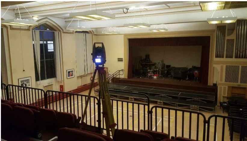
Whiteley Hall Before the Fire
