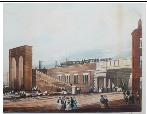
The western approach with the Stationmasters house at the right hand side,
